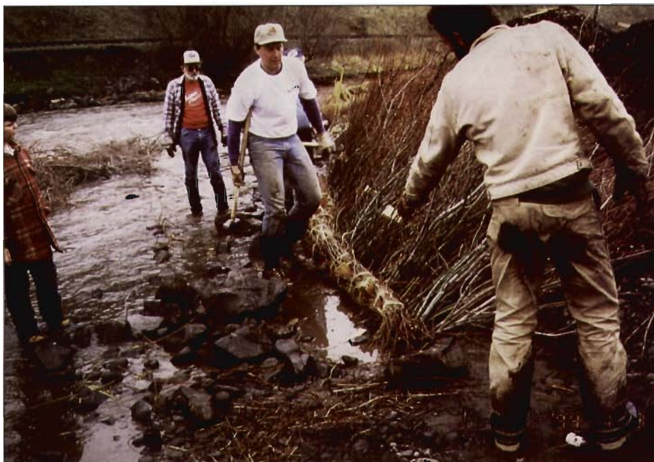
Figure 6-10. Brush mattress with live fascine during construction.
