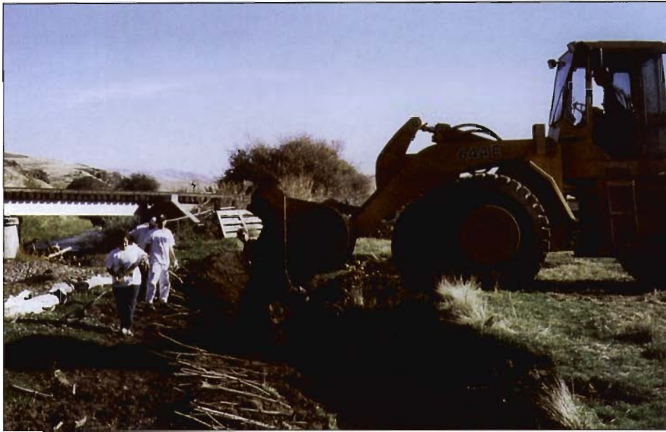
Figure 6-13. Brush layer during construction.
