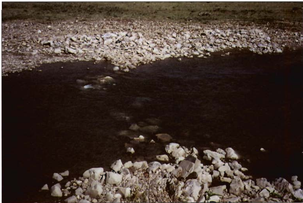
Figure 11-7. Rock V-weir in the Castle River, Alberta. Scour immediately downstream of the point of the weir caused the point rocks to slip downstream during a >1:200-year flood.
