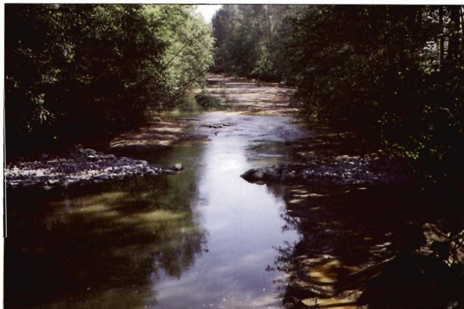
Figure 11-2. Opposing deflectors in the lower Coquitlam River, B.C. These structures have survived several flood events in a low gradient, sand/gravel bed section of the river. Note stable, well-vegetated banks.
