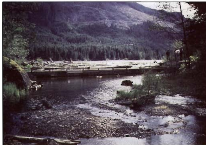
Figure 14-3. A small concrete control dam with a manually operated control gate, located at the outlet of Keogh Lake on northern Vancouver Island.
