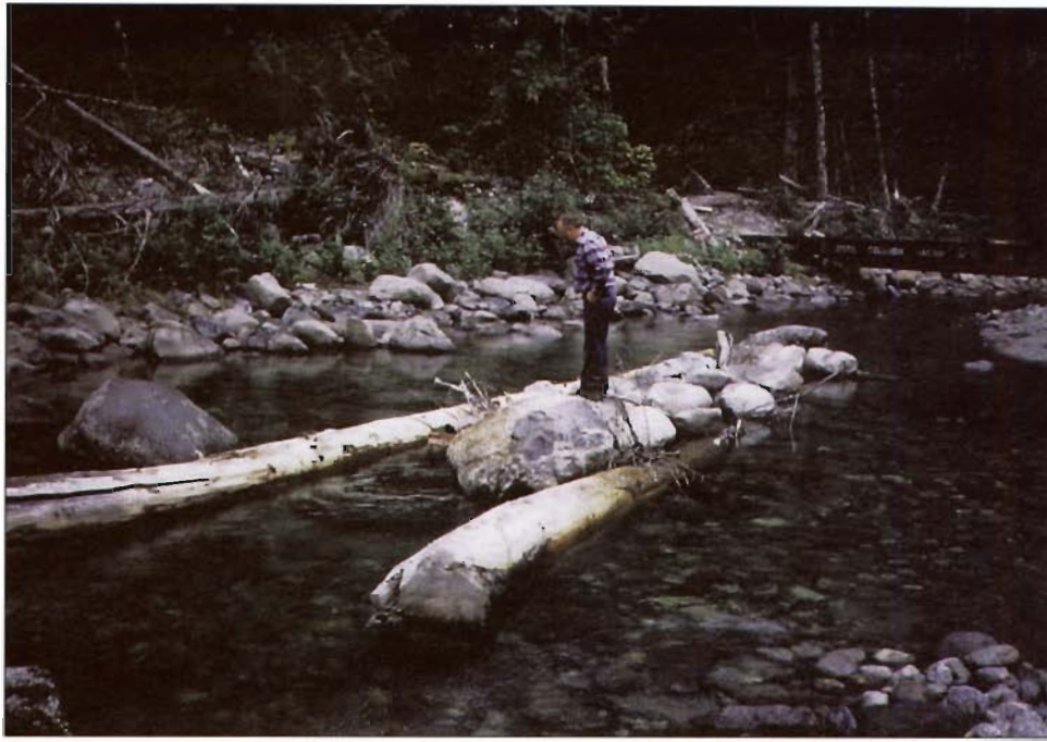
Figure 9-22. A low profile reef installed in a coastal stream is inspected for fish utilization and depth of scour. Cables were wrapped around the main logs at the two points where notched cross logs were attached. A matrix of small poles and branches was used to support the cobbles and boulders required to sink and secure the reef.
