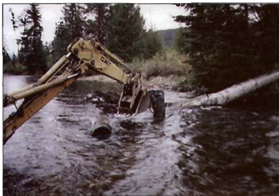
Figure 9-20A. Loading a floating pile debris catcher with a rootwad and large key log connected from the V of the catcher to the base of a tree on shore.
