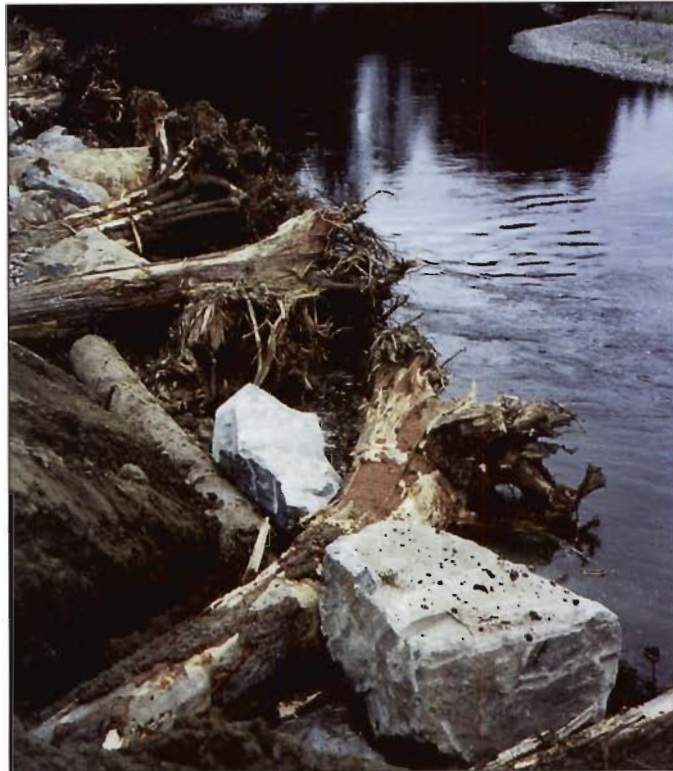
Figure 9-15. Use of large boulders and full length rootwad complexes to stabilize an eroding bend of the Green River, Washington; the upper bank was treated with geotextile, cuttings and staking, revegetation and riparian tree planting (Hamakami Biostabilization Project; photo by Johnson and Stypula).
