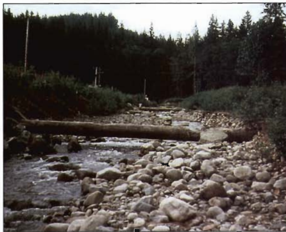
Figure 5-12. Log weir that has been seriously undermined as a result of being installed perpendicular to the bank and too high in the water column.
