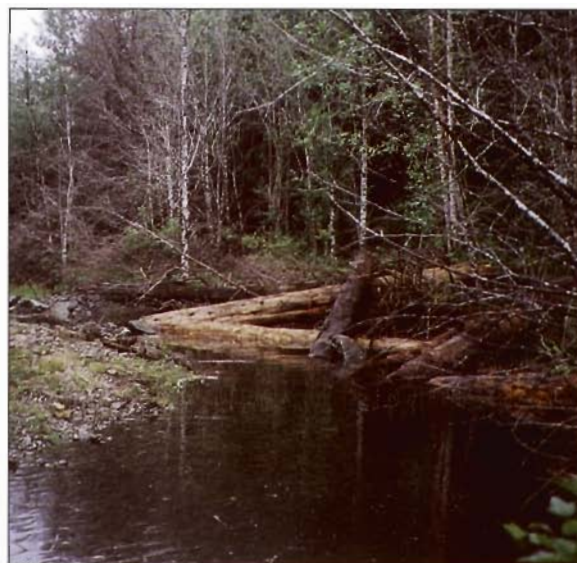
Figure 9-14B. After: a deepened pool that was backwatered to increase its depth by increasing the height of the downstream riffle (see Chapter 12); a LWD-boulder complex was anchored into the tail of the pool, also armouring the eroding stream bank.
