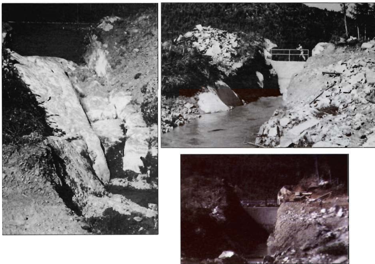
Figure 14-1. A small flow control structure provides increased flows during the summer and early fall to improve spawning conditions and rearing habitat for coho and steelhead juveniles. The left photograph shows the initial construction stages of an open-cut channel which was blasted through bedrock to allow water to be drawn from the lake. The right photograph shows a simple, reinforced concrete wall installed with a manually-operated sluice gate to control the discharge from the lake.
