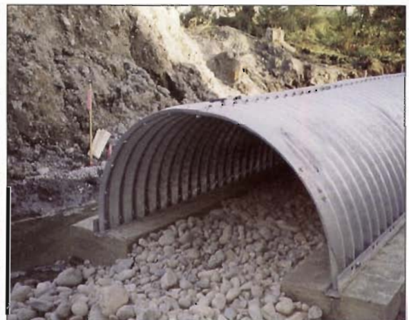
Figure 5-2. This culvert has addressed fish passage by providing a semi-natural streambed throughout.
