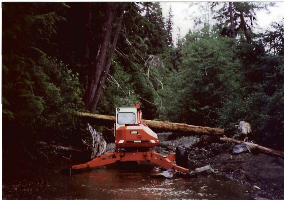
Figure 9-13. Spider excavator installing a right-angled LWD-boulder lateral jam at a minor bend of the Keogh River to restore large woody structure for scour pool formation. Most of the boulders, logs and rootwads were transported by helicopter to this reach where there was no adjacent road access.
