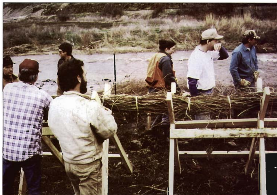
Figure 6-8. Live fascine being assembled.
