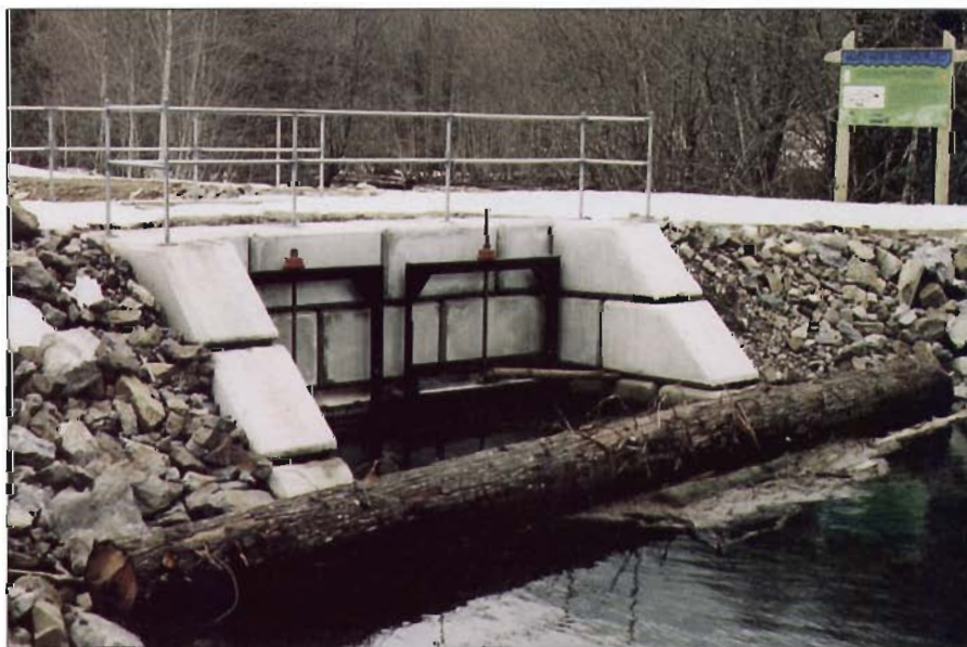
Figure 7-12. Concrete intake with box culverts and manually operated slide gates, Centennial Channel, Chilliwack River.
