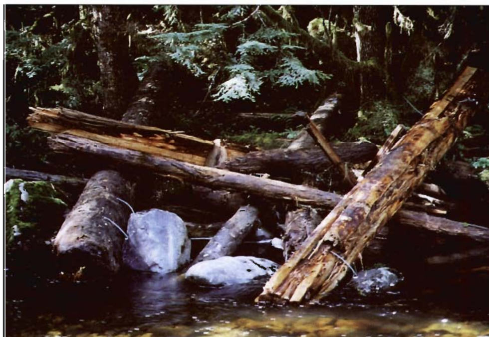
Figure 10-7. At sites where large woody debris (LWD) had historically been present on the Keogh River, bank-side debris jams were constructed by importing LWD and boulders; key logs were anchored with large (>0.8 m diam.) boulders using wire rope cables and epoxy, and the whole structure was interconnected and secured to riparian trees. These structures have been stable following winter freshets, often capturing additional LWD. They have created highly usable habitat for juvenile salmonids during summer and winter, as well as cover for spawning adults.
