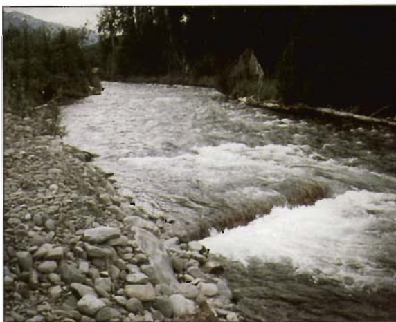
Figure 5-11. Log deflector extending halfway across channel. A pool has formed downstream of the deflector, with gravels accumulating upstream of the deflector and at the tail of the pool.
