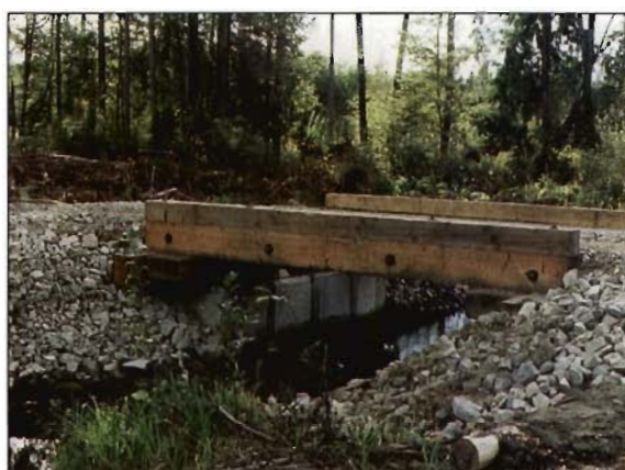
Figure 5-4. This timber bridge retains the natural streambed and provides for passage of juvenile fish.
