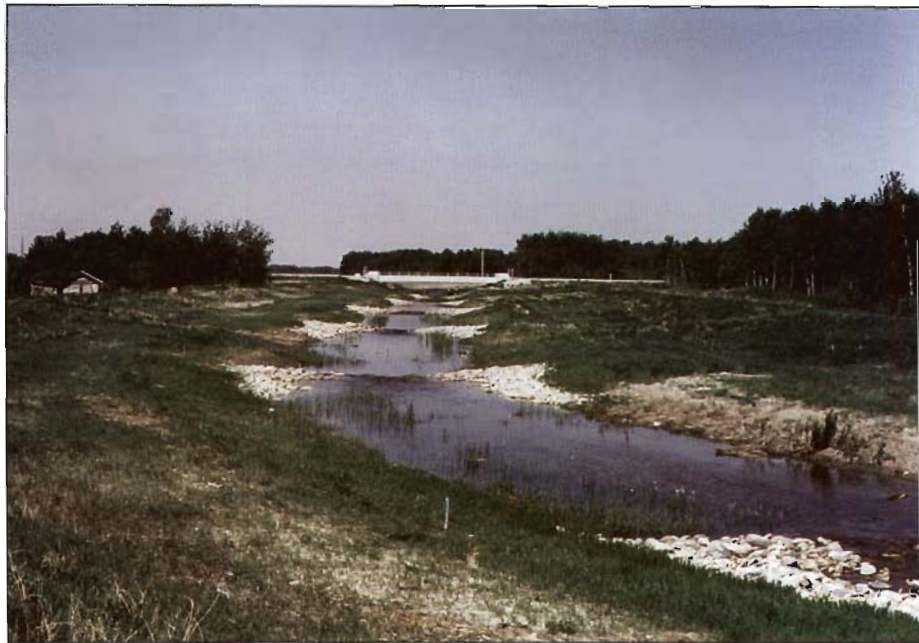
Figure 12-17. Mink Creek Walleye Spawning Restoration Project 1988, Central Manitoba. The channelized reach three years after rock riffles were added. After several bankfull and greater flood events formed downstream pools, the channel has stabilized. The riffles and pools are utilized by spawning walleye.
