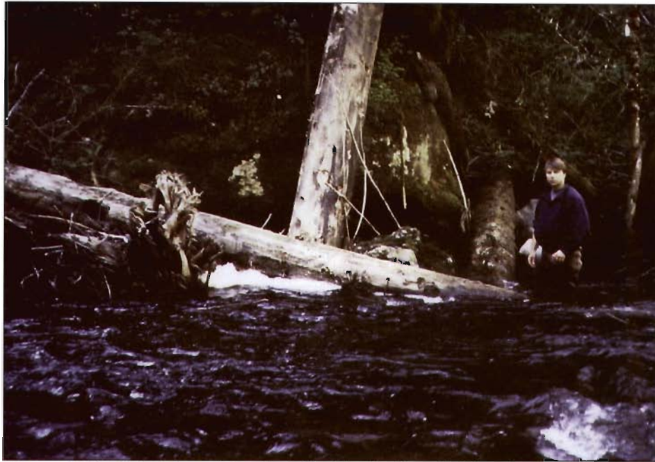
Figure 9-19. A debris catcher installed in the Keogh River in 1996 to create complex lateral pool habitat.
