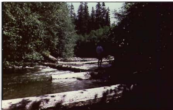
Figure 8-17. Attached LWD at USFS project on the Mount Baker Snoqualmie National Forest. Logs are secured by boulders and rebar. (Myron Kozak photo)
