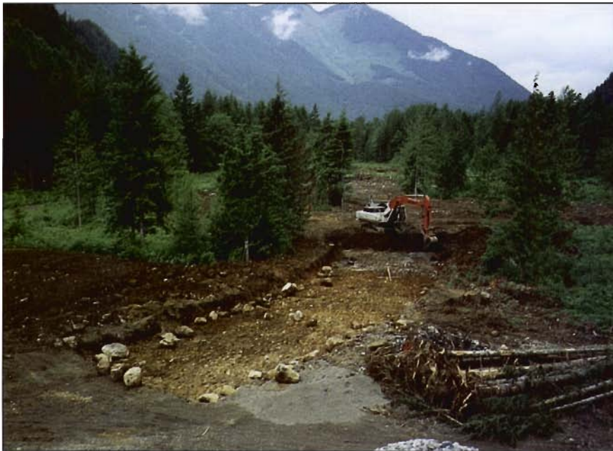
Figure 7-22. Excavation of a surface-fed channel showing stock piles of conifer trees and boulders, Centennial Channel, Chilliwack River.
