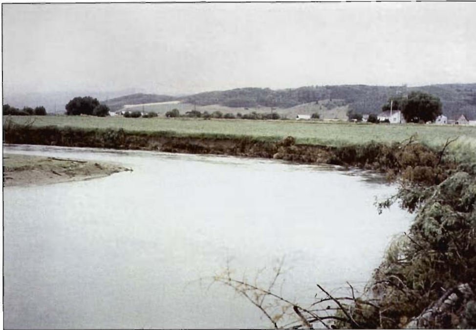
Figure 6-20. Tree revetment installed at a low energy site.
