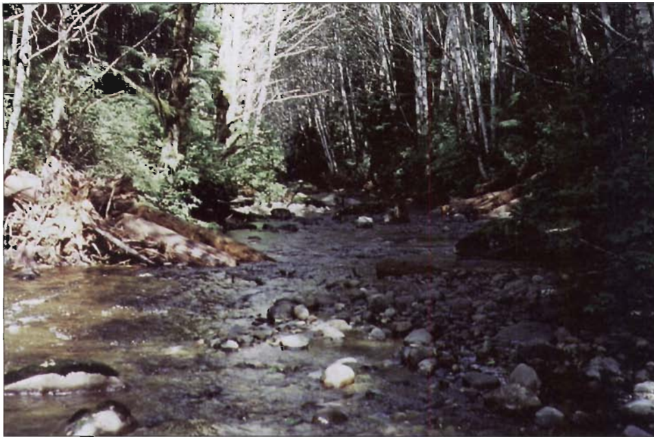
Figure 9-5. A series of lateral jog jams installed in 1996 (pre-scour before winter floods) at bends in residual low gradient sites adjoining steeper (2%) sections of a reach of the upper Keogh River. Post-freshets, these boulder and bank anchored logs and rootwads formed lateral scour pools. (Encroachment of LWD complexes on the channel were limited because of stream bank confinement associated with past road fills.)
