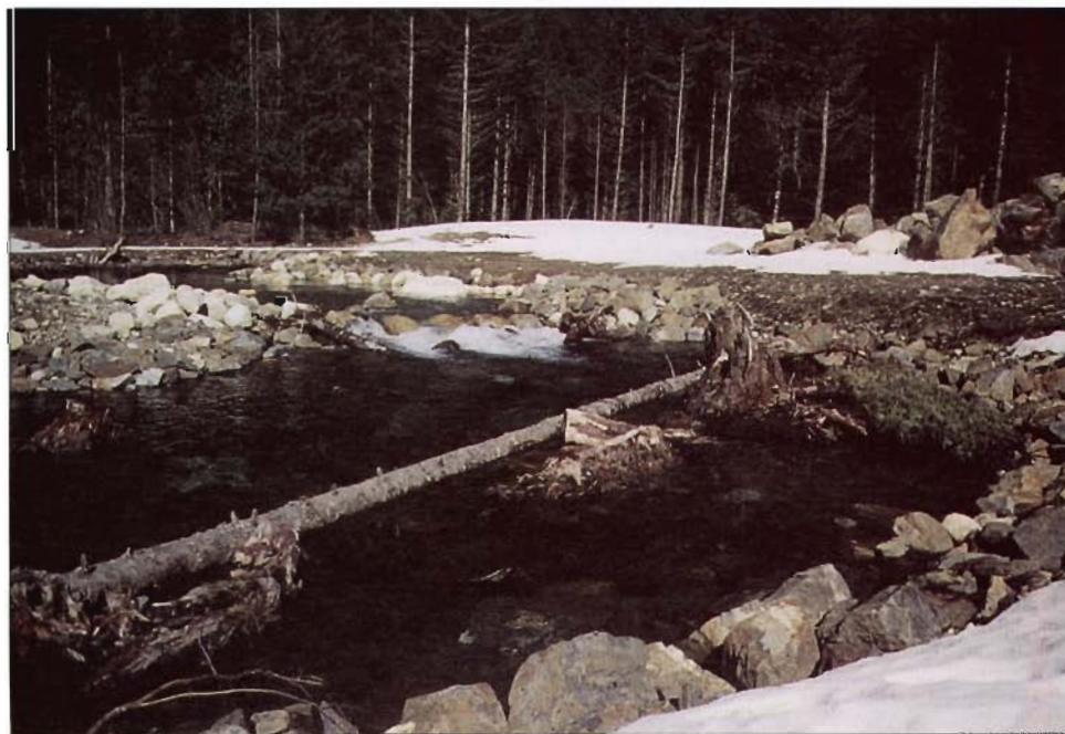
Figure 7-17. Pool with riprap bank armour and wood debris cover, Centennial Channel, Chilliwack River.
