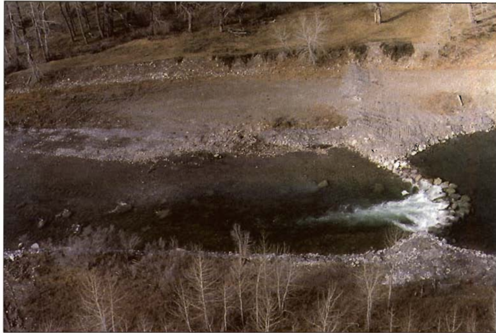
Figure 11-6. Rock V-weir in the Oldman River, Alberta. Note excavated pool/run and cover rocks downstream of the weir. The left upstream arm of the weir extends across the gravel bar to tie in to the bank.
