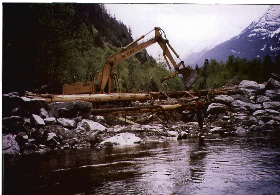
Figure 7-9. Log curtain wall under construction, Shovelnose Creek, Squamish River.
