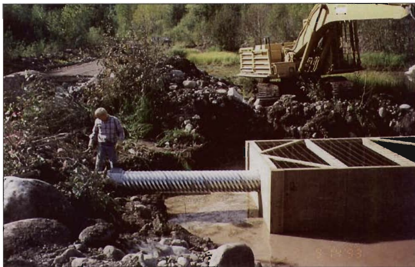
Figure 15-9. Dewatered plywood cage attached to upstream end of culvert.
