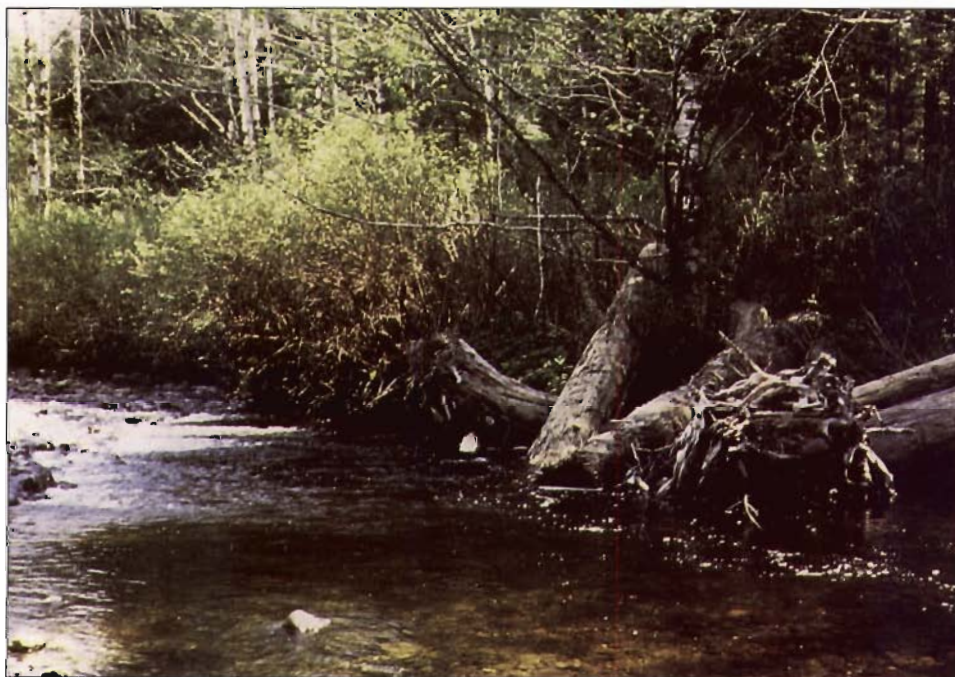
Figure 9-10. A triangular lateral log jam anchored with large boulders in the channel and to tree bases on the bank. The log-rootwad-boulder composite structure was installed in a residual pool within a minor bend of the Keogh River, logged to the stream banks by past logging practices.
