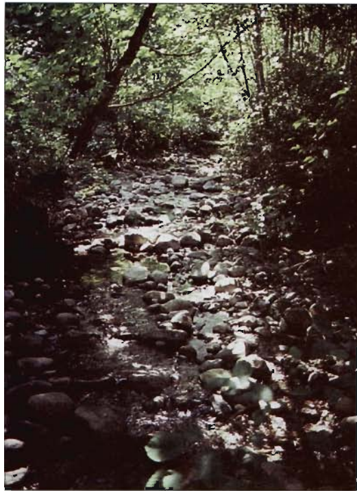
Figure 12-22. Oulette Creek 1993, Howe Sound, B.C. The channelized reach degraded approximately 1 m between 1978 and 1994, developing a uniformly sloping bed of large cobbles with limited hydraulic and habitat diversity.
