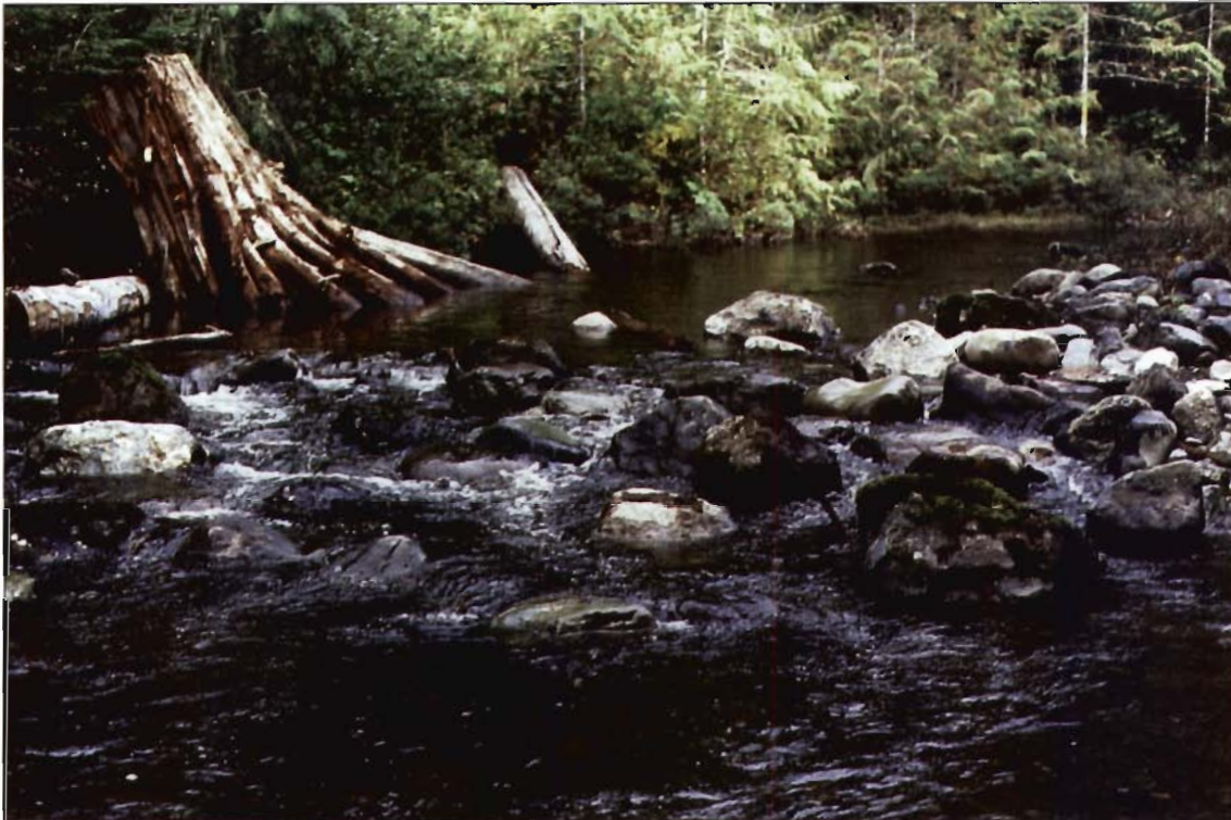
Figure 12-13. Riffle-pool reconstruction at the upper Keogh River in 1996. The riffle crest was increased in height to add 30 cm depth to the pool upstream and to maintain a deep pool at the base of the riffle. As a key component, LWD was anchored (epoxy technique) upstream and downstream of the riffle to maintain sufficient cover for both rearing juveniles and adult spawners.
