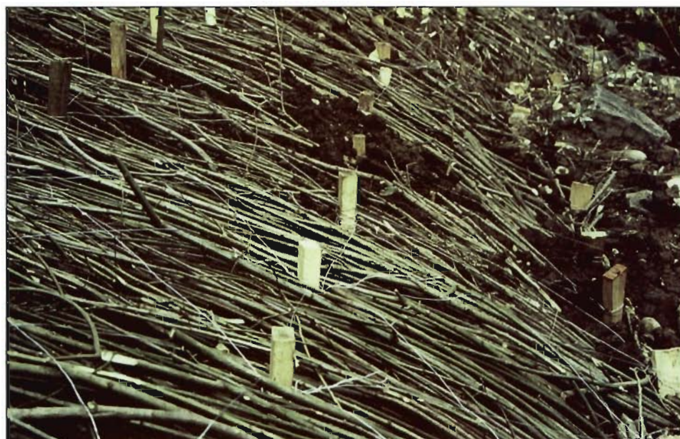
Figure 6-11. Brush mattress during construction; note rock toe.
