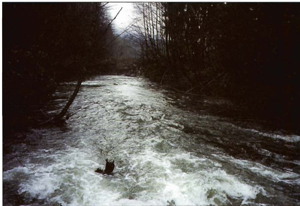
Figure 12-9. Oulette Creek Restoration Project 1994, Howe Sound, B.C. Downstream view overlooking constructed riffles at the bankfull flood discharge. The low-flow pool and riffle steps are submerged as the average gradient of the water surface and stream bed become parallel. Critical velocities are occurring locally on the riffle crest.
