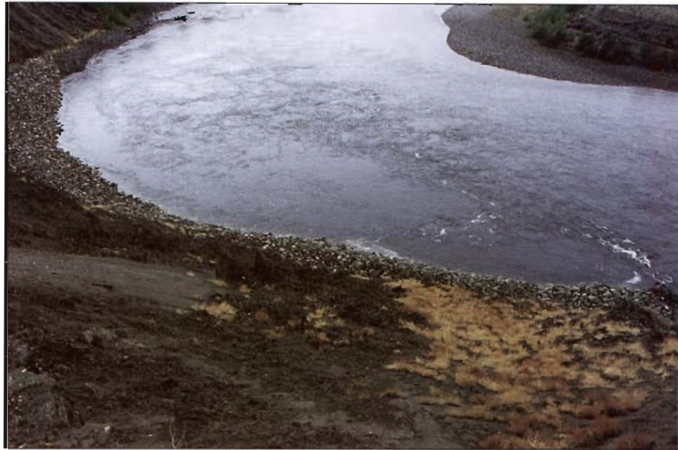
Figure 6-4. Rock revetment with groyne at Thompson River, B.C.
