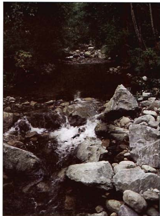
Figure 12-23. Oulette Creek Restoration Project 1994, Howe Sound, B.C. The channelized reach following the addition of rock riffles. Shallow gravel bars deposited in the pools are utilized for spawning. Juvenile fish have occupied the deeper sections. The habitat is now equally distributed between riffles and pools.
