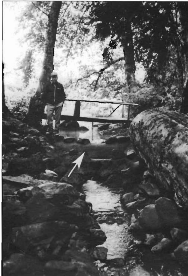
Figure 14-2. A one-meter high dam constructed of hand mixed concrete and boulders. The dam provided storage in 27 ha (69 acre) Matheson Lake, Vancouver Island, to increase summer flows for rearing juvenile coho and trout.
