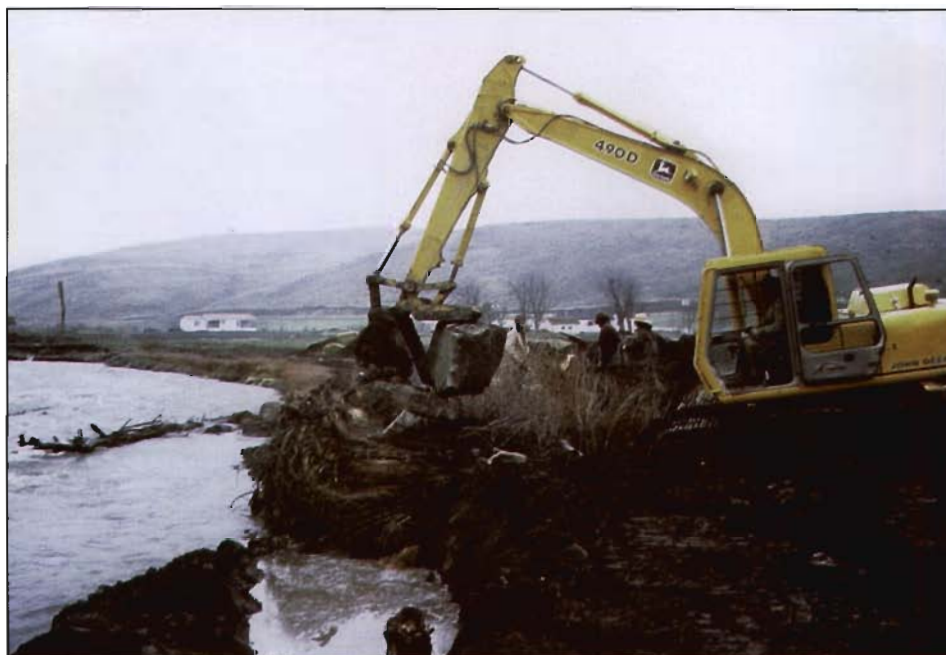
Figure 6-22. Tree revetment during installation at a moderate energy site.
