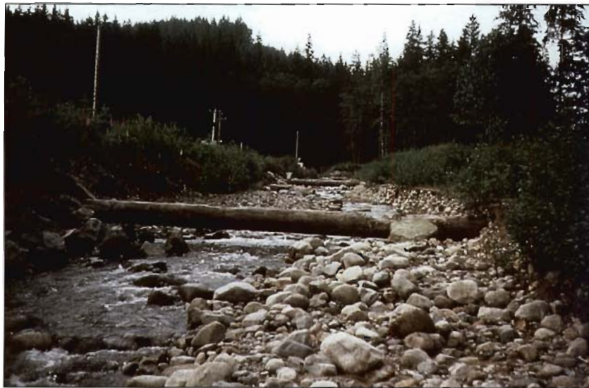
Figure 12-19. Oulette Creek 1982, Howe Sound, B.C. In the first three years following channelization, the single log drop structures added to the uniform channel were undercut and the single-line boulder drop structures were buried in deep scour holes formed immediately below the structure crests. There were no shallow downstream riffle slopes to convey the flows away from the toe of the structures.
