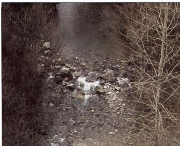
Figure 5-8. Aerial view of a riffle template to create spawning habitat. Large boulders are located at the crest of the riffle to provide stability.
