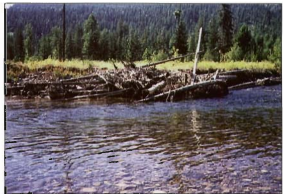
Figure 9-20B. A lateral log debris jam created in 1994 by a floating V-log debris catcher in the West Kettle River. The resulting 2 m deep and complex pool was inhabited in 1996 by 15-20 rainbow trout and about 40-50 mountain whitefish.
