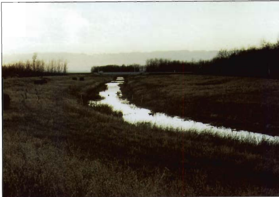
Figure 12-15. Mink Creek Walleye Spawning Restoration Project 1985, Central Manitoba. The channelized and unstable reach prior to the addition of rock riffles. The drainage area tributary to the reach is 250 km 2 .
