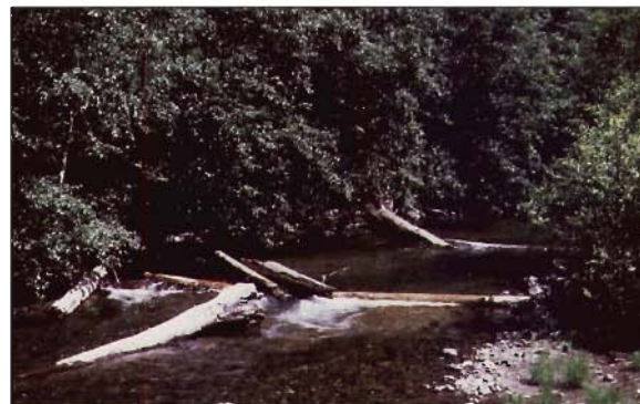
Figure 8-18. Attached woody debris at a USFS project on the Mount Baker Snoqualmie National Forest. Logs are attached to bedrock (epoxy-cabled) and the stream bank. (Myron Kozak photo)
