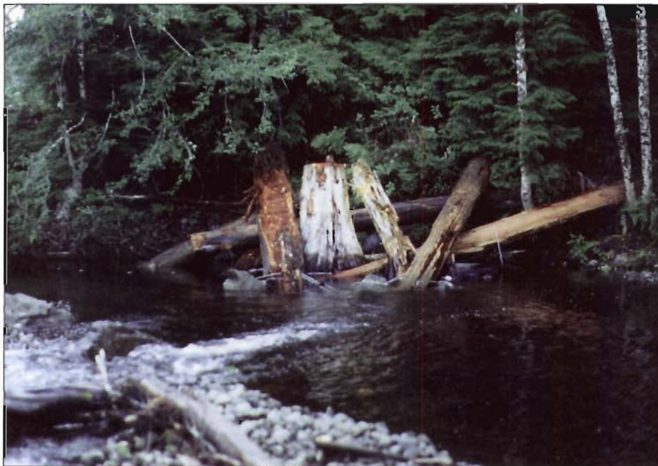
Figure 9-8. A lateral log jam installed in the Keogh River aligned to a sharp bend, to armour an eroding bank, catch debris and scour a deep pool as prime habitat for juvenile and adult fish.
