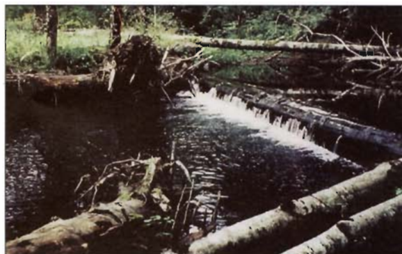
Figure 8-8. Porter Creek, WA. Full-spanning log, rootwad and energy dissipation.
