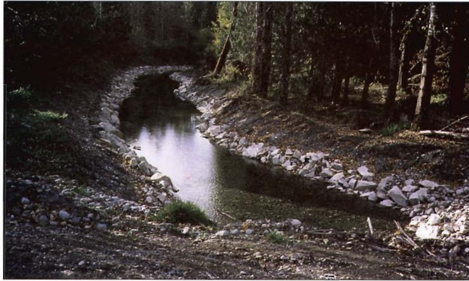
Figure 7-7. A groundwater channel just after construction, Usher's Channel, Chilliwack River.
