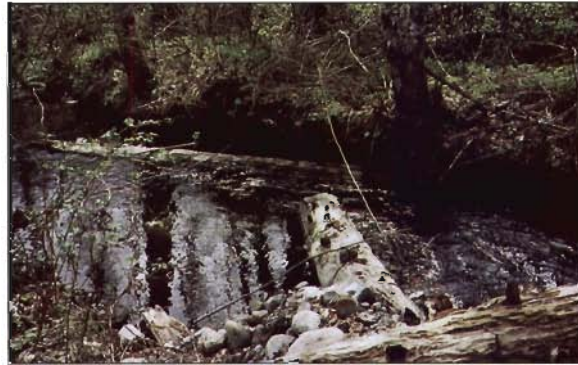
Figure 8-16. A log deflector with floating bank cover installed in Shop Creek in the upper Squamish River watershed
