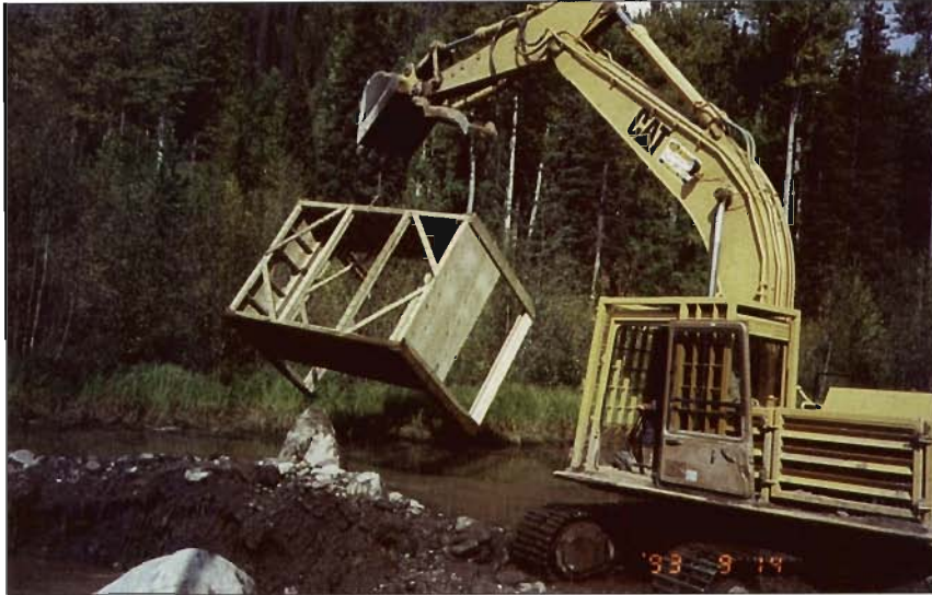
Figure 15-8. Installation of plywood cage with wire mesh top and bottom.
