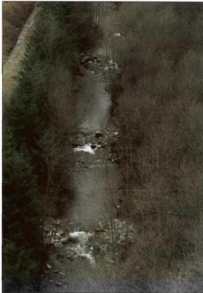
Figure 12-20. Oulette Creek 1994, Howe Sound, B.C. Rock riffles have been added to the former drop structure sites. In the ensuing 16 years, the riparian zone has revegetated with firs (planted), alders, maples and a shrub understory.
