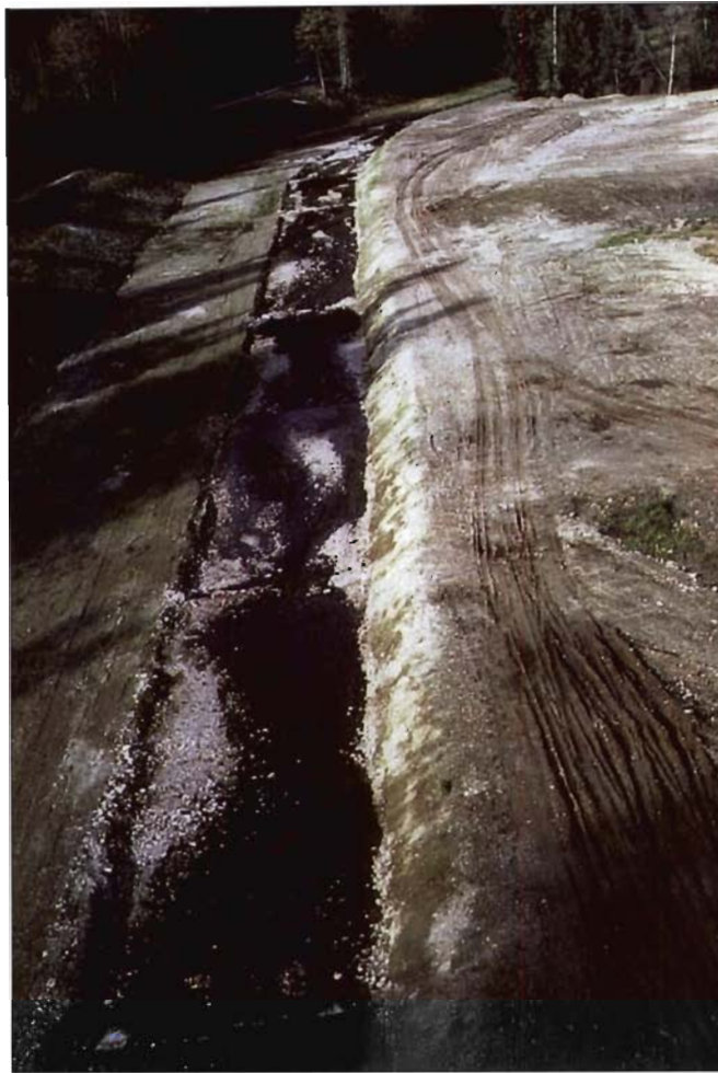
Figure 12-1. Oulette Creek 1978, Howe Sound, B.C. In 1978, the lower reach was diverted and channelized to create a sawmill and log sort yard on the alluvial fan. Single log and rock drop structures were constructed in the channel that subsequently failed.
