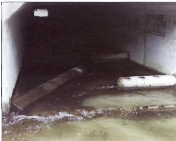
Figure 5-1. Baffles in this culvert alter hydraulic conditions to improve fish passage.
