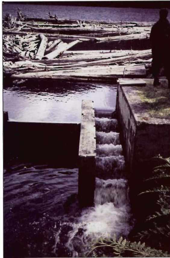
Figure 14-4. Manually-operated stop logs and an adjustable juvenile fishway were installed to improve summer flow releases to the Keogh River from Keogh Lake on northern Vancouver Island.
