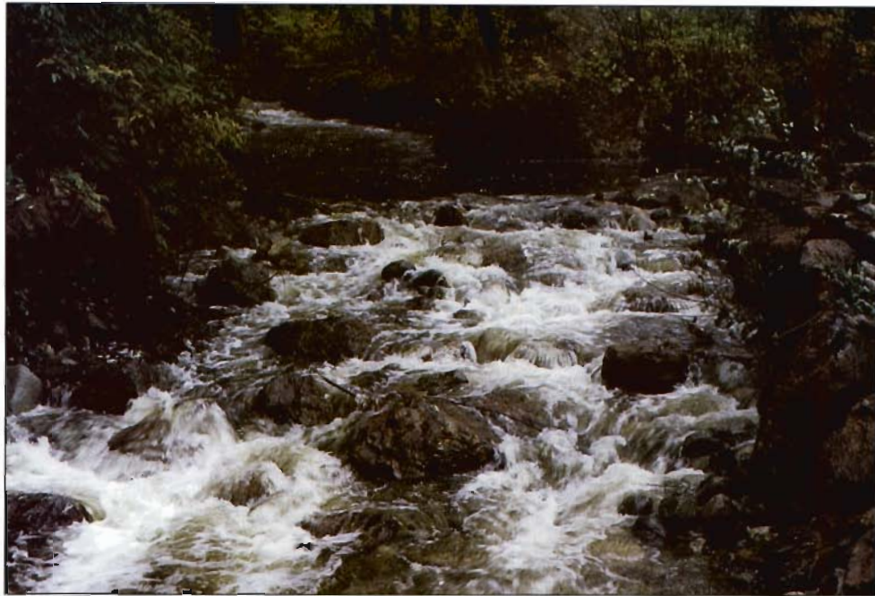
Figure 12-11. Langdale Creek Restoration Project 1995, Howe Sound, B.C. Diverse hydraulic conditions have been created by strategically placing large boulders on the downstream face of this constructed riffle. Note the well riprapped banks in the riffle zone adjacent to the reconstructed Sunshine Coast highway.
