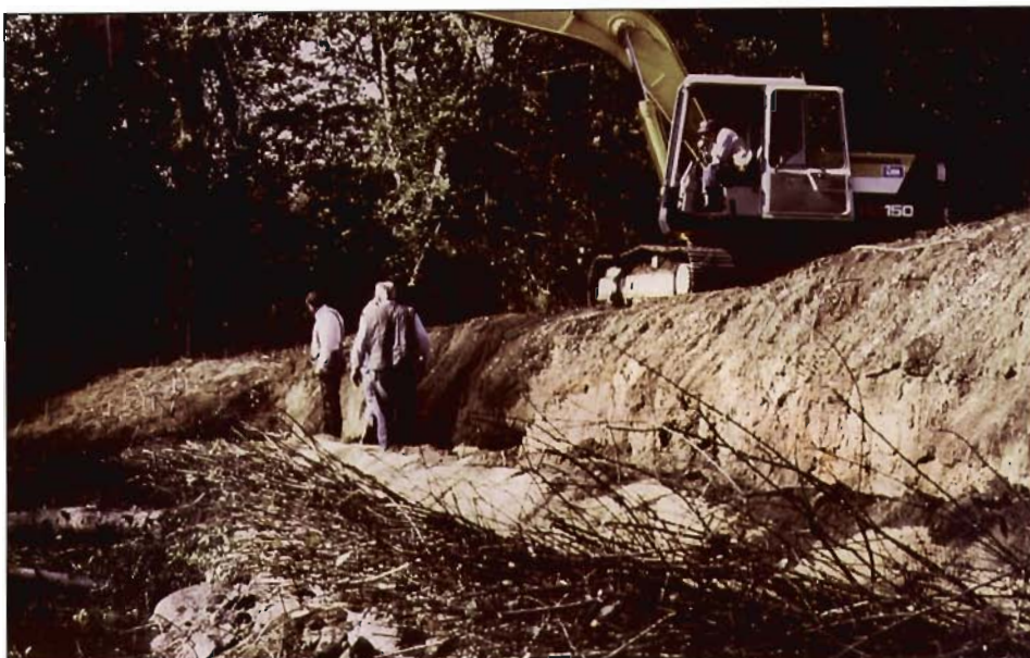
Figure 6-16. Vegetated geogrid during construction; note live cribwall in lower left corner.
