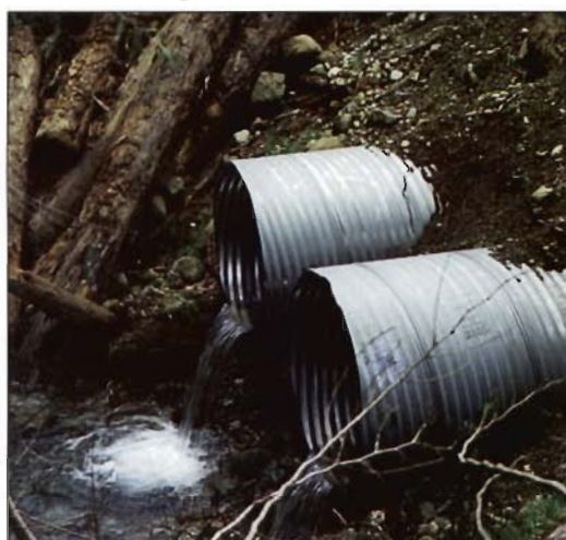
Figure 5-3. Juvenile fish are generally incapable of entering and/or swimming through poorly installed culverts.
