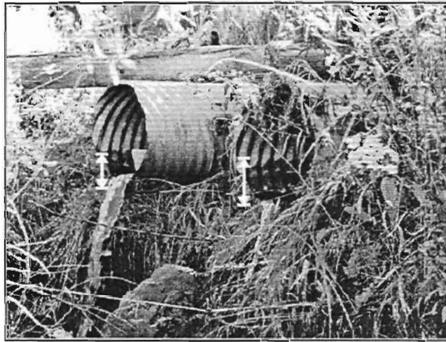
Figure 4. Rust stains on these dual culverts in the Swift River watershed show a high water mark.
