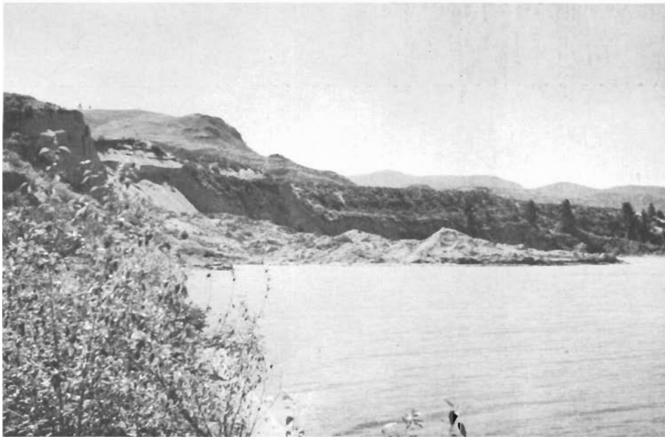
Plate VI. A landslide which occurred in glacial-lake silts on the shore of Osoyoos Lake. The silts were apparently saturated by excess irrigation water. The movement took place rapidly and was completed within a few minutes.
