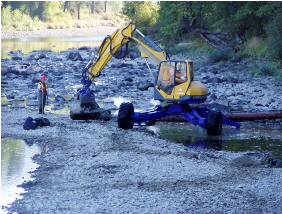
Photo A 4. Spyder-hoe excavator used in constructing triangular ramp-log structure on the Kettle River in 2008.
