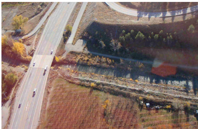
Photo 8. Trout Creek fan and Highway 97 crossing.
