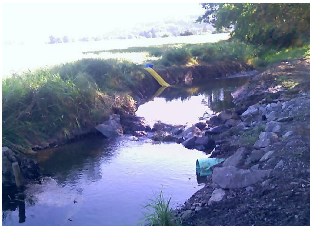
Photo 8. Big Ditch sediment trap post-maintenance.
