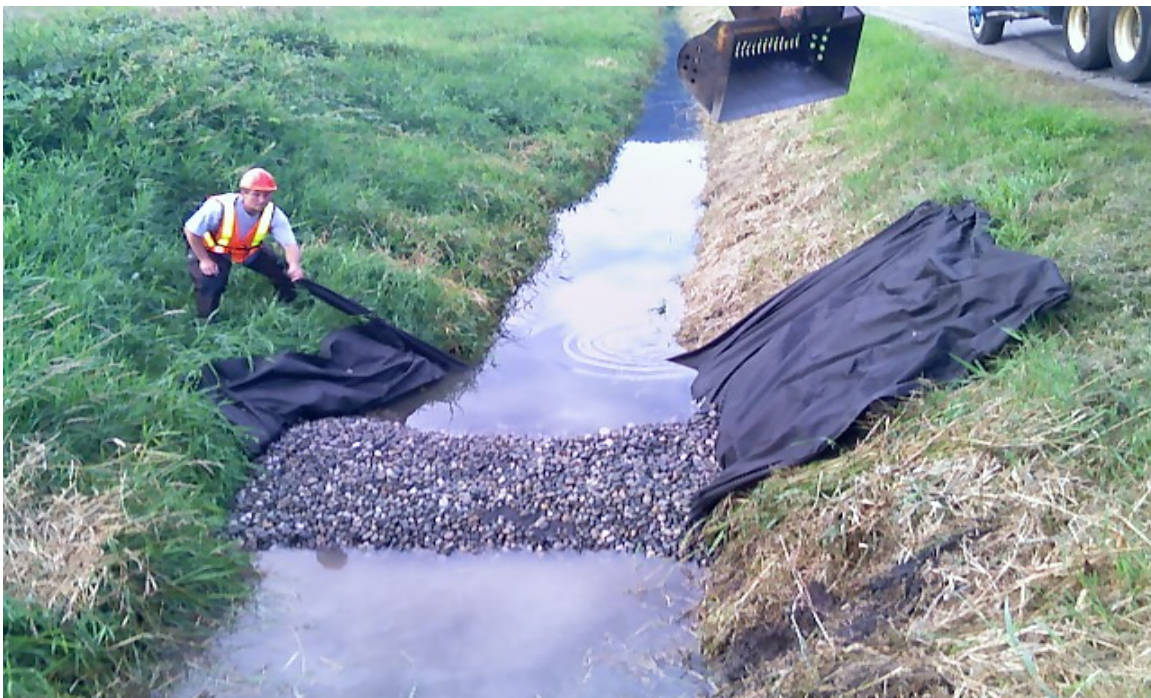
Photo 2. Turbidity control measures at downstream end of maintenance area.
