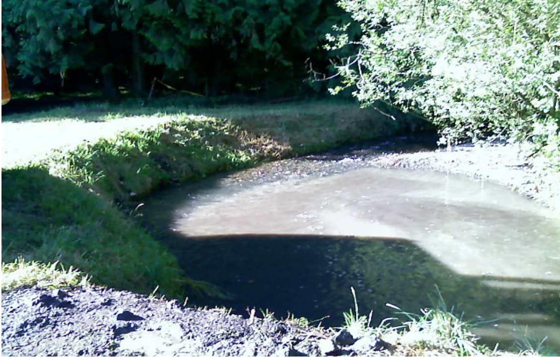
Photo 1. Nevin Creek sediment trap during excavation.
