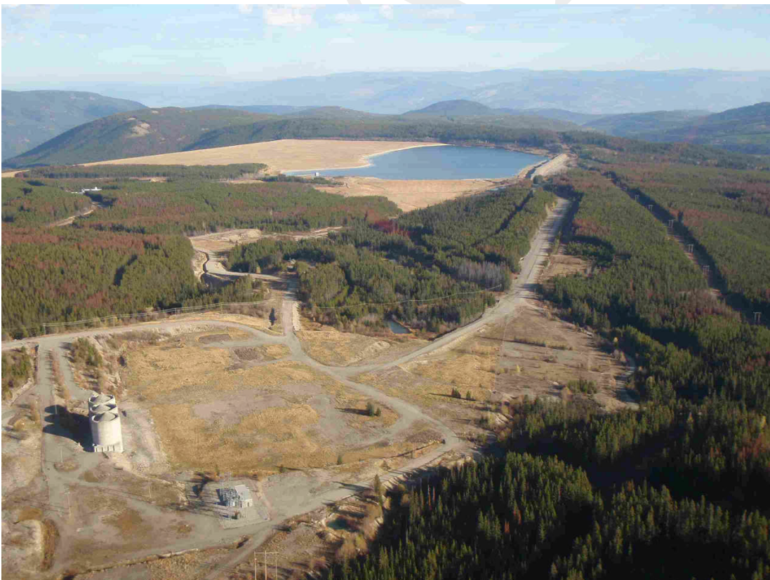
Photo 6. Brenda Mines tailings pond in MacDonal Creek sub-basin, looking east towards Okanagan Lake. Trepanier Creek valley is on upper left of photo.
