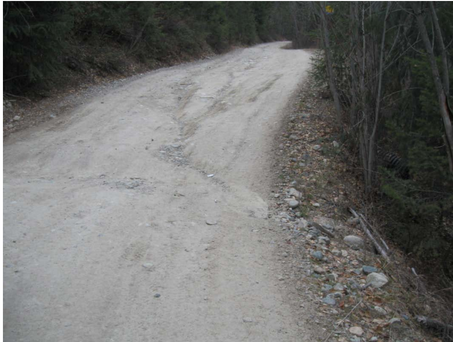
Photo 21 – Surface condition of Monroe Forest Road – drainage directed across road surface causing erosion (P-3)
