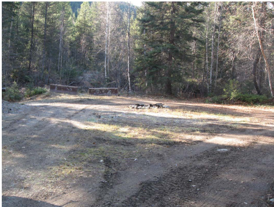
Photo 76 – End of road to Trepanier Park, bridge removed (T-12)
