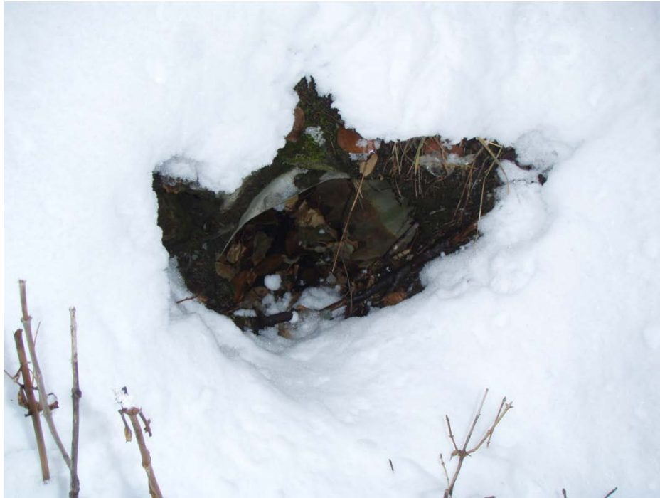
Photo 47 – Partially blocked culvert on Brenda Mine Road. (P26)
