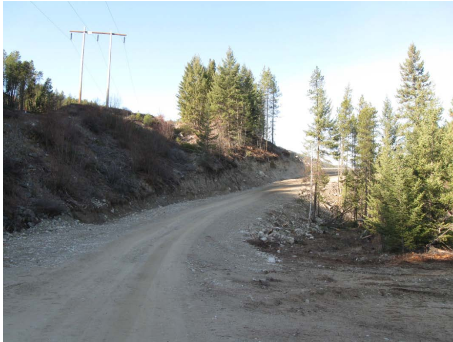
Photo 69 – Eroding cutbanks on newly created road to gravel pit (T-7)
