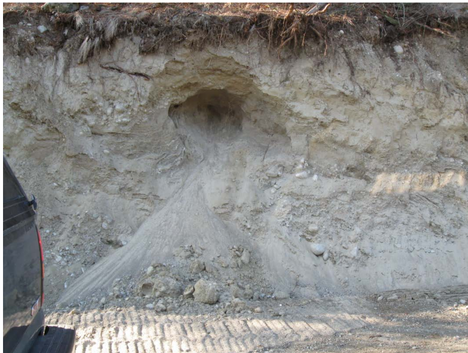
Photo 70 – Eroding cutbanks on newly created road to gravel pit (T-7)
