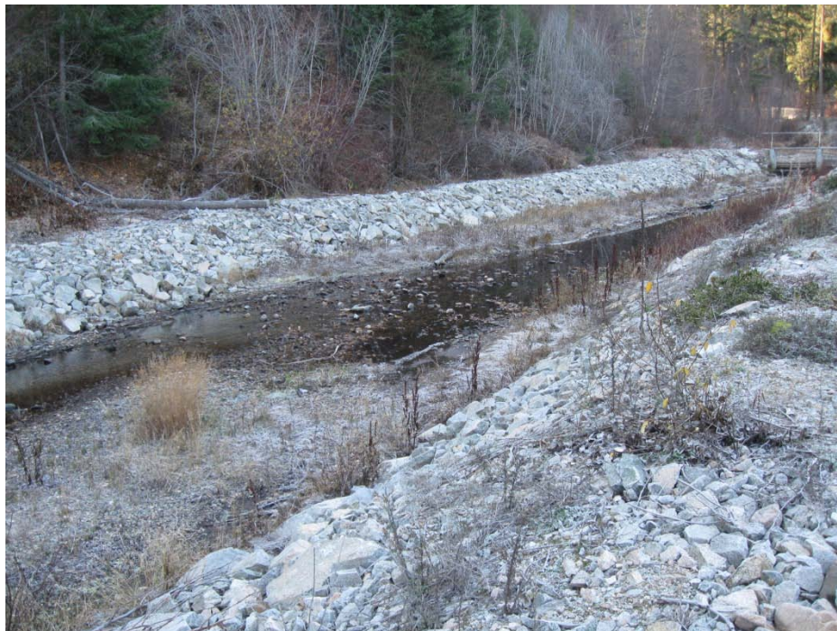
Photo 6 – Peachland Creek downstream of Intake weir
