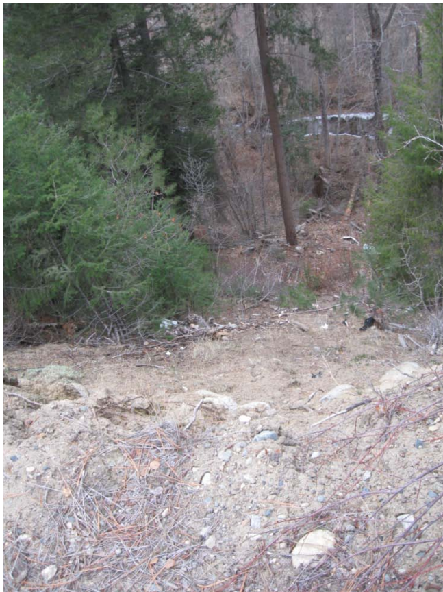
Photo 24 – Erosion at switchback on Monroe Forest Road – note creek (P-5)
