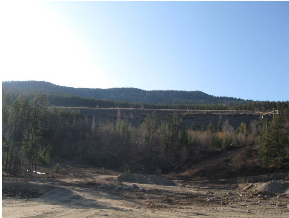
Photo 85 – Large exposed cuts on Highway 97C (T-32)
