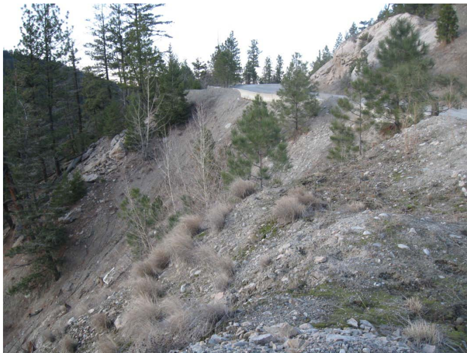
Photo 36 – Steep slopes on Princeton Ave. vulnerable to erosion and slides (P-12)
