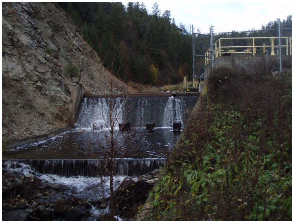
Photo 4 – Slope Peachland Creek –downstream—flow control-- weir
