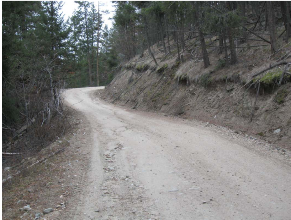
Photo 29 – Eroding cutbank at second switchback on Monroe Forest Road (P-7)
