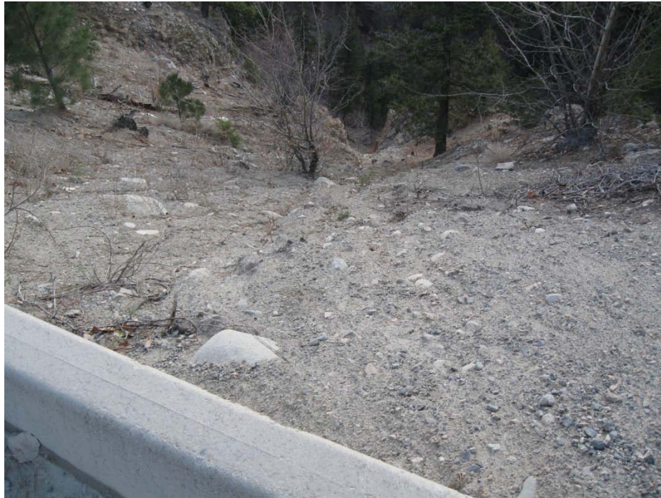
Photo 37 – Steep slopes on Princeton Ave. vulnerable to erosion and slides (P-12)
