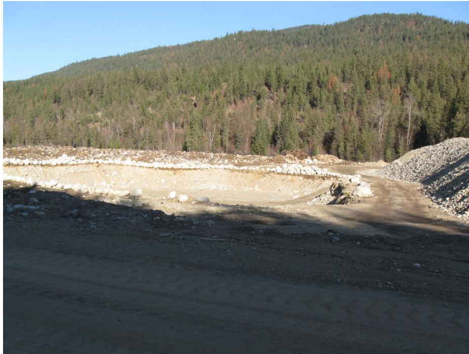
Photo 65 – Large extraction site beside Trepanier Creek (T-6)
