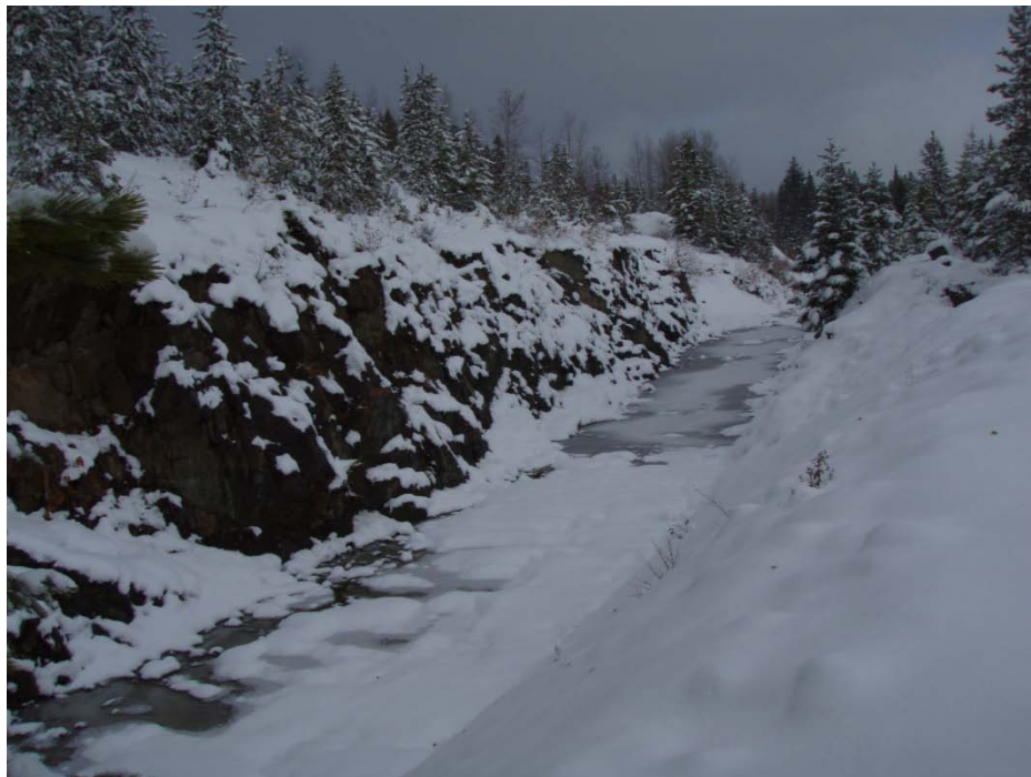
Photo 50 Exposed cuts in Peachland Lake spillway (P-28)
