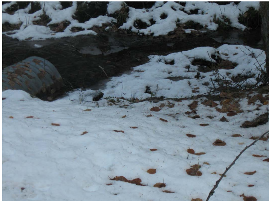
Photo 88 – Culvert at creek crossing upgradient of Silver Lake, cattle and wildlife access (T-35)
