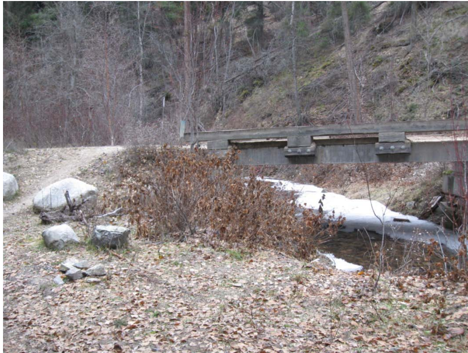
Photo 19 – Access to creek from both sides of Monroe Forest Road bridge over Peachland Creek (P-2)
