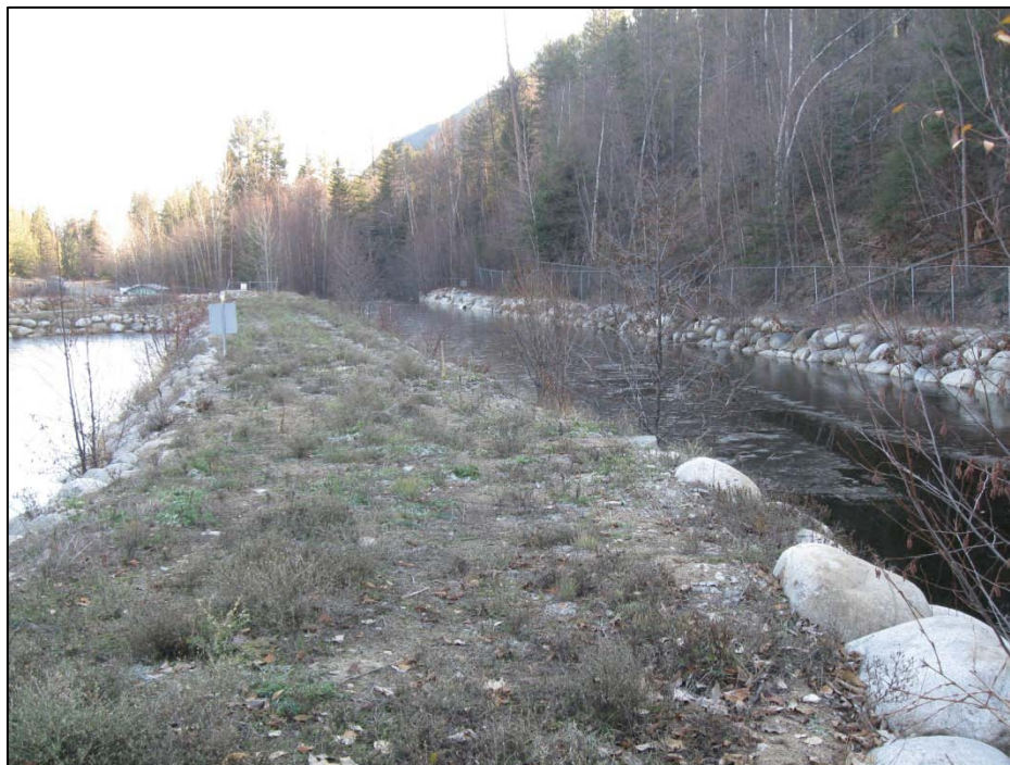
Photo 16 – Trepanier Creek at intake pipes, looking downstream (southeast)
