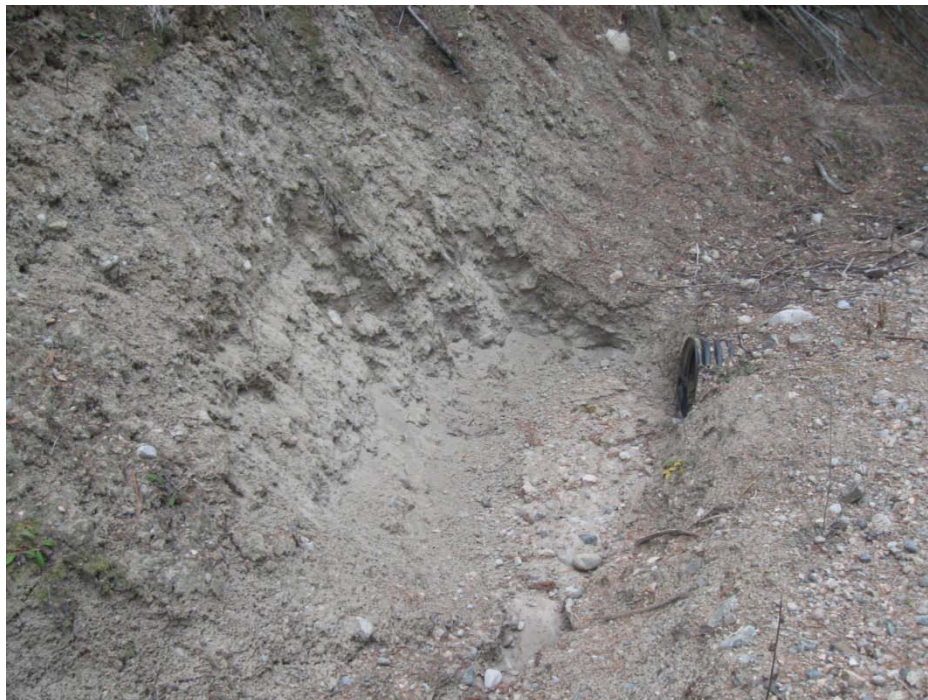
Photo 30 – Eroding cutbank at second switchback on Monroe Forest Road (P-7)
