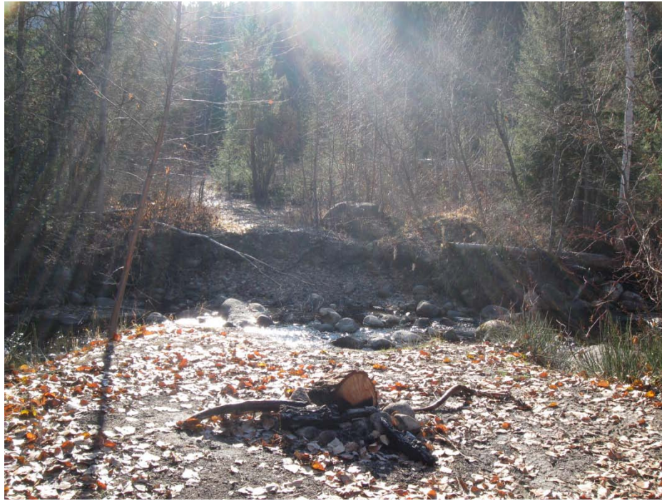
Photo 73 – Old creek crossing, bridge removed (T-10)
