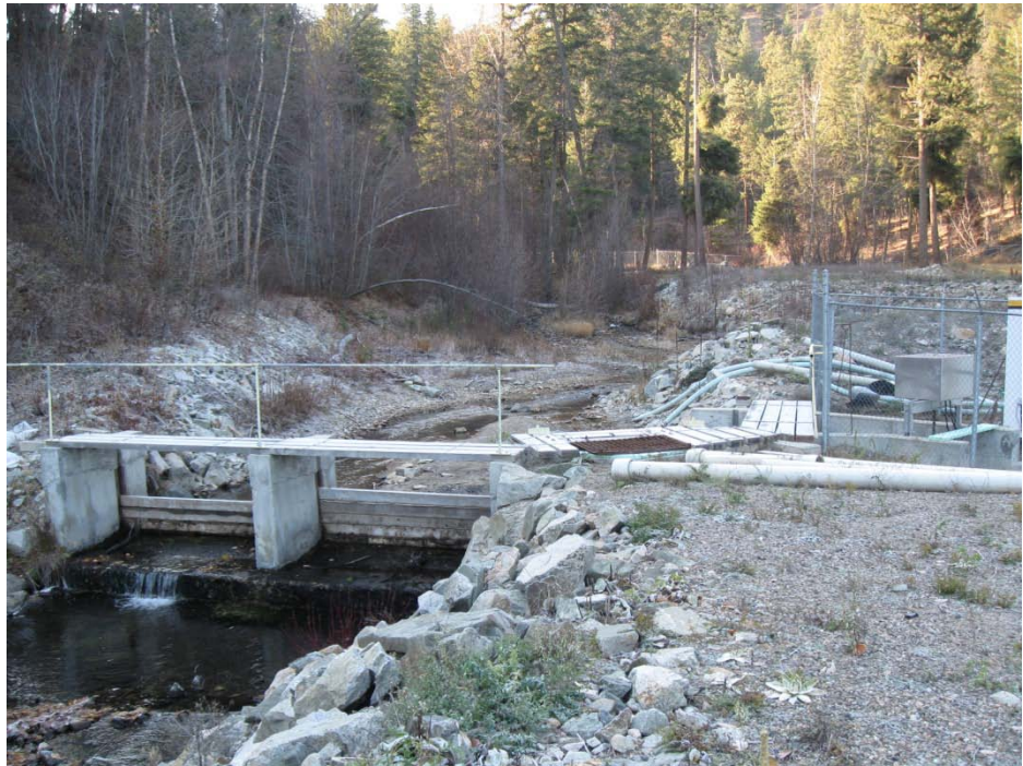
Photo 2 – Peachland Creek Intake weir, looking upstream
