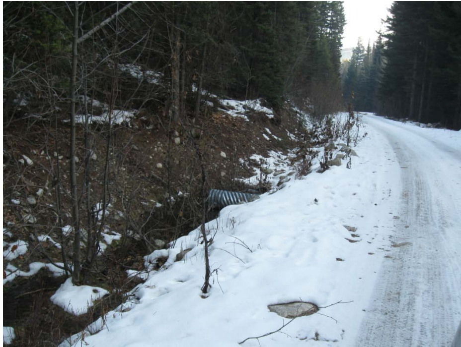
Photo 89 – Road example in Silver Lake area, cattle and wildlife access to water in ditches (T-36)
