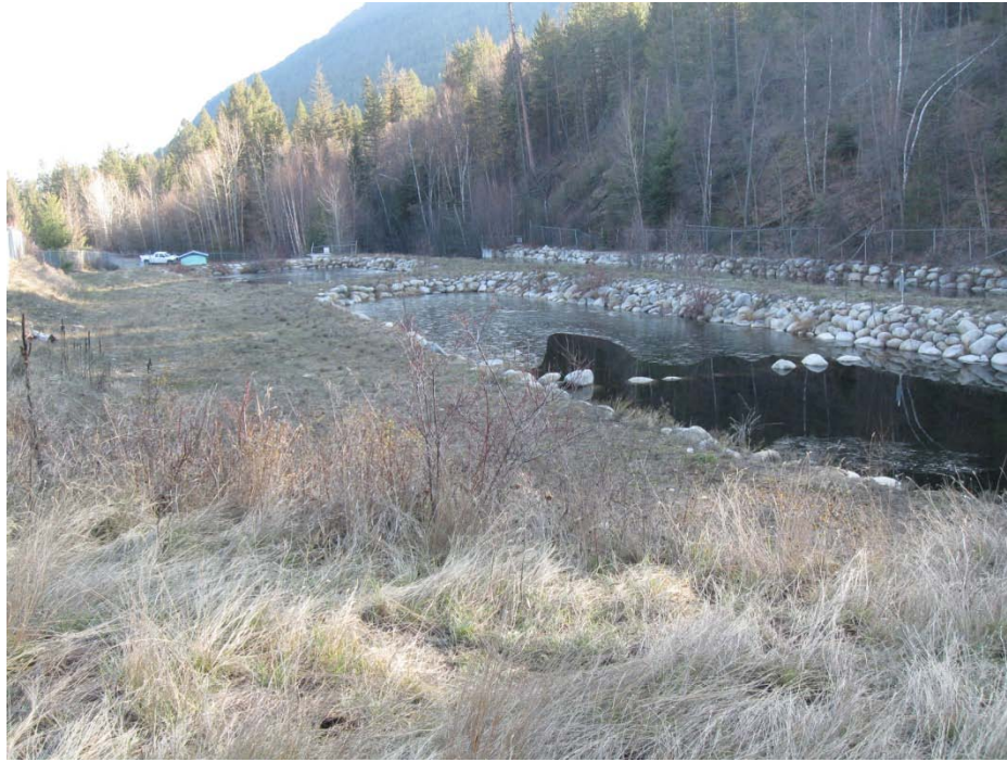
Photo 13 – Settling Ponds at Trepanier Creek intake facility, looking downstream (southeast)
