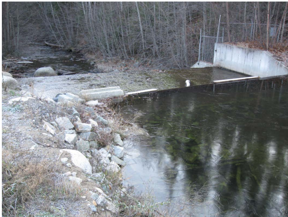
Photo 14 – Flow control weir on Trepanier Creek
