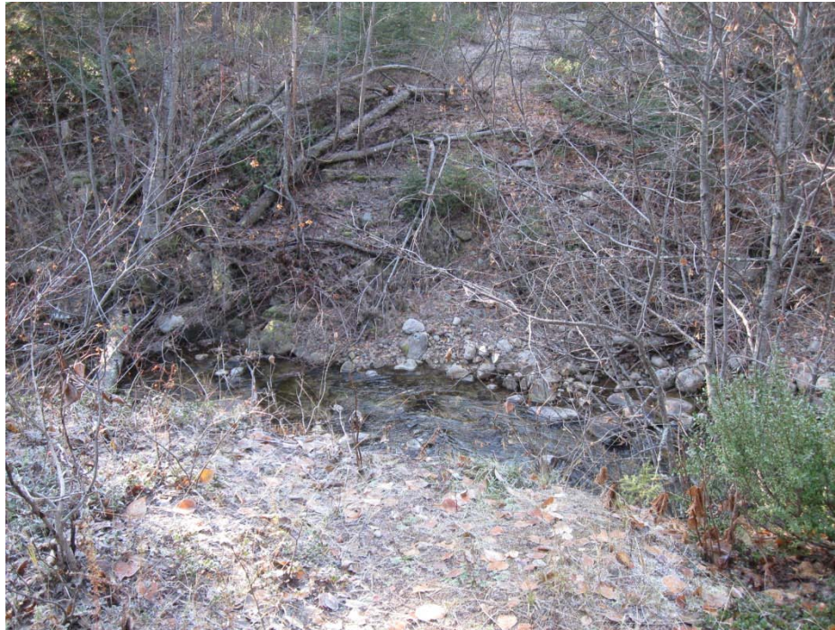
Photo 77 – Bridge removed at end of road to Trepanier Park (T-12)
