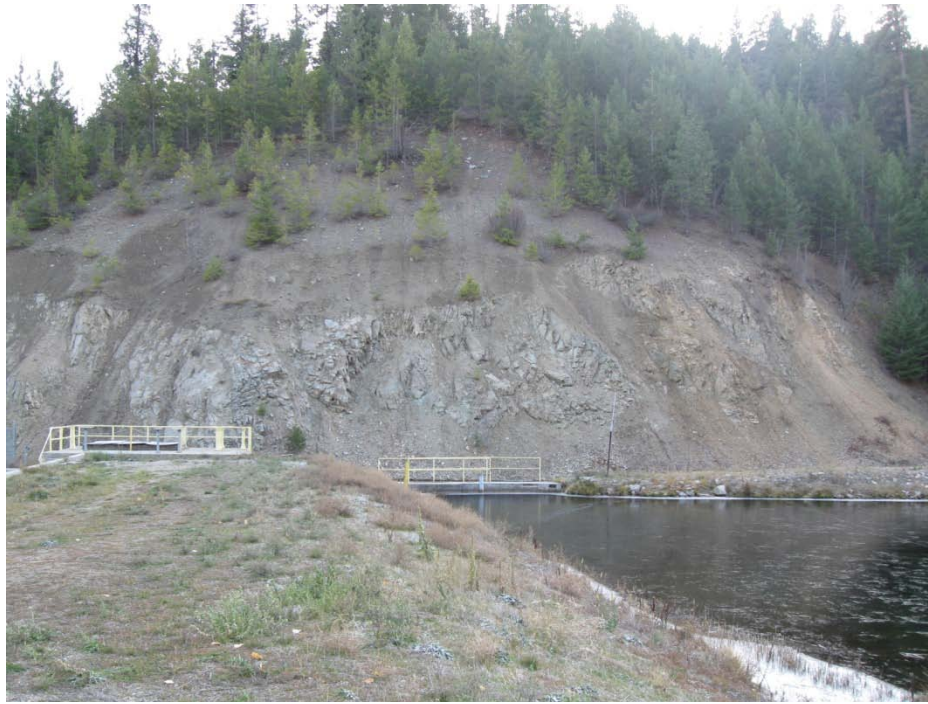
Photo 9– Sloughing slope on Peachland Creek beside the flow control weir
