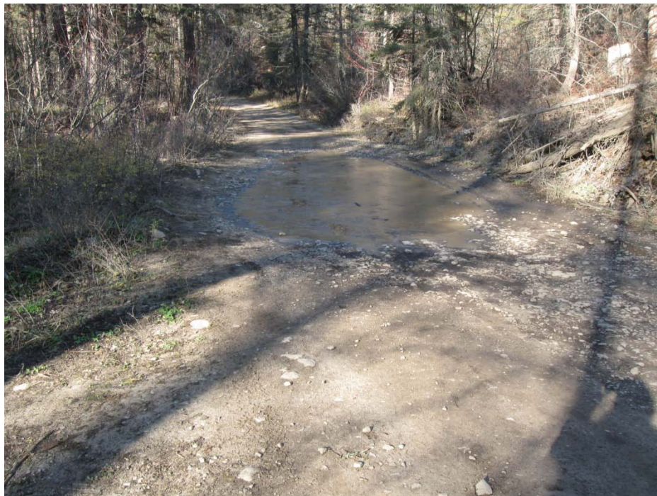
Photo 72 – Road to Trepanier Park – example of ponding on road (T-9)
