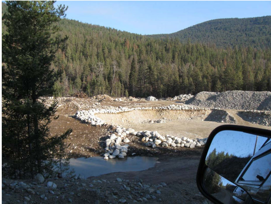
Photo 67 – Camper trailer at excavation site (T-6)
