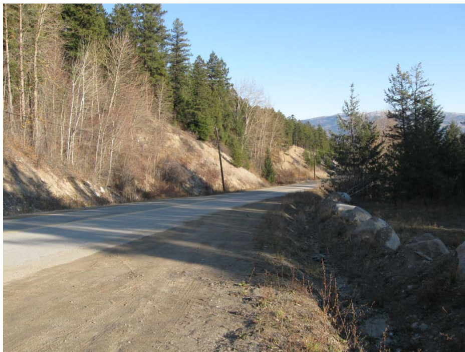
Photo 38 – Example of cutbanks on Princeton Ave. (P-13)
