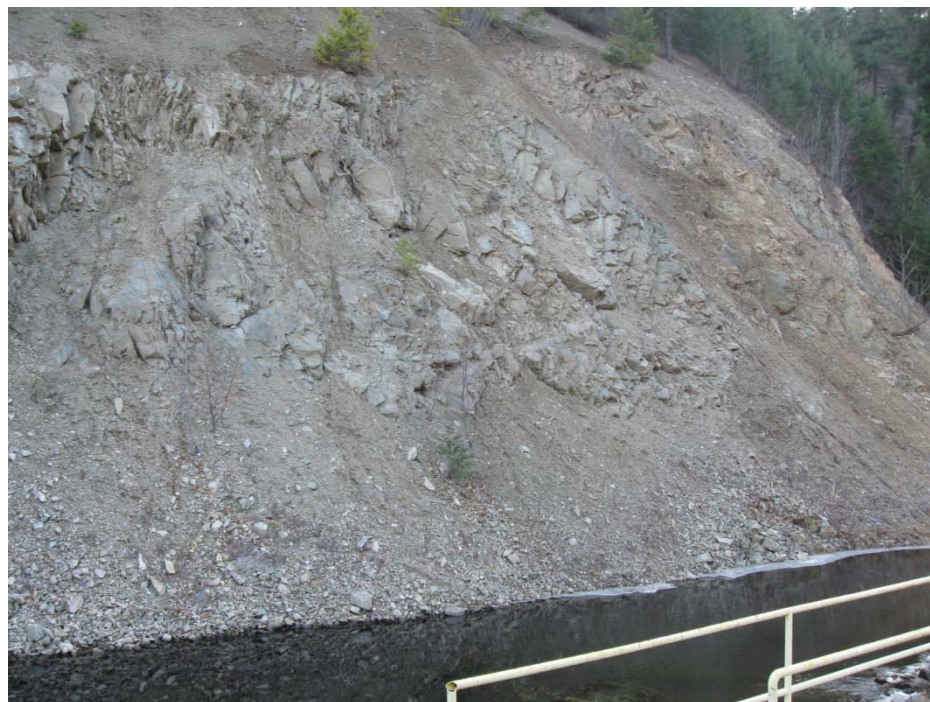
Photo 8 – Sloughing slope on Peachland Creek beside the flow control weir
