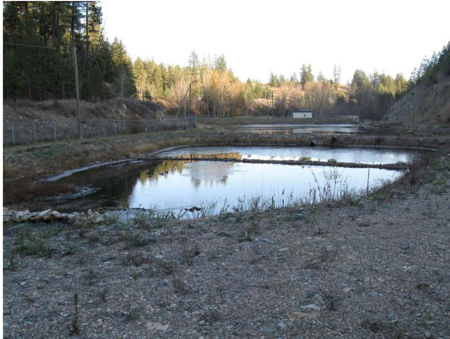
Photo 3 – Peachland Intake ponds, looking east from intake weir
