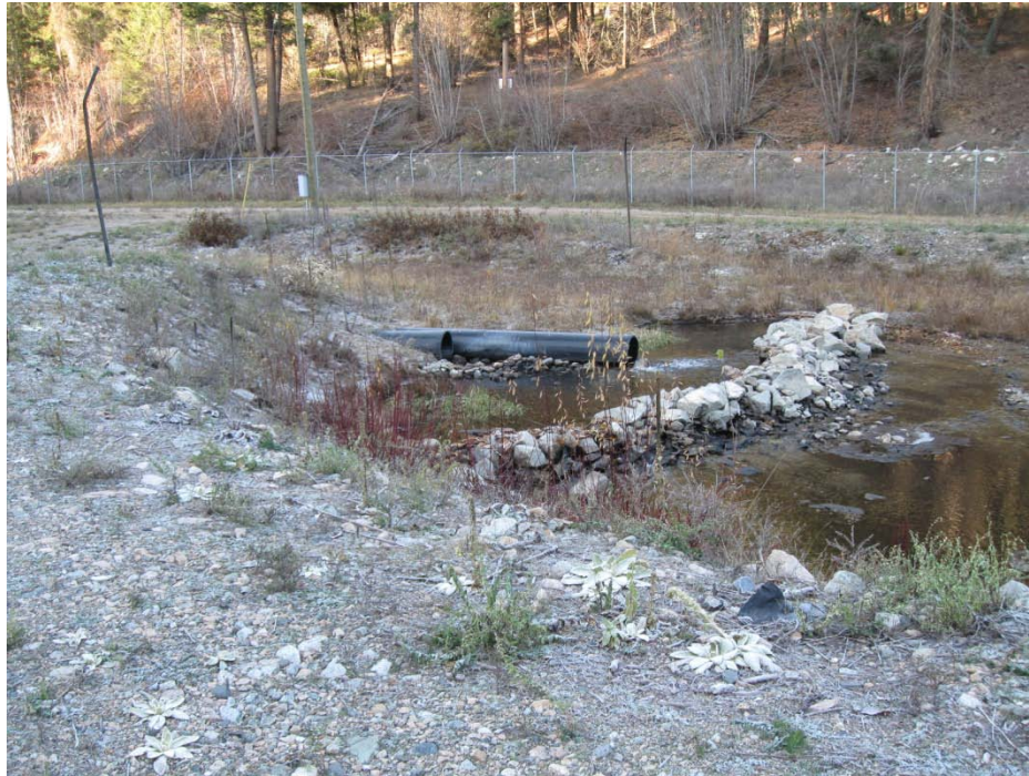
Photo 5 – Outlet of intake weir into the settling pond
