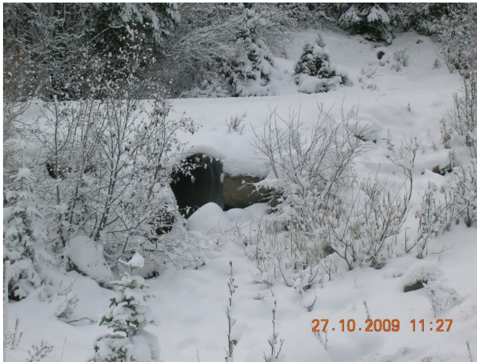
Photo 52 – Culvert on Peachland Forest Service Road (P-31)
