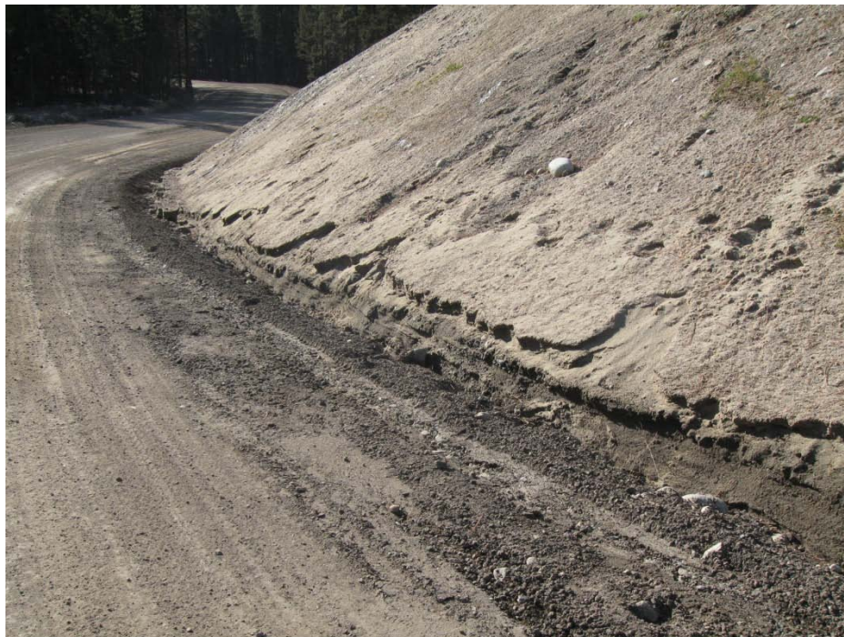
Photo 60 – Exposed and eroding cutslope on road to gravel pit (T-3)
