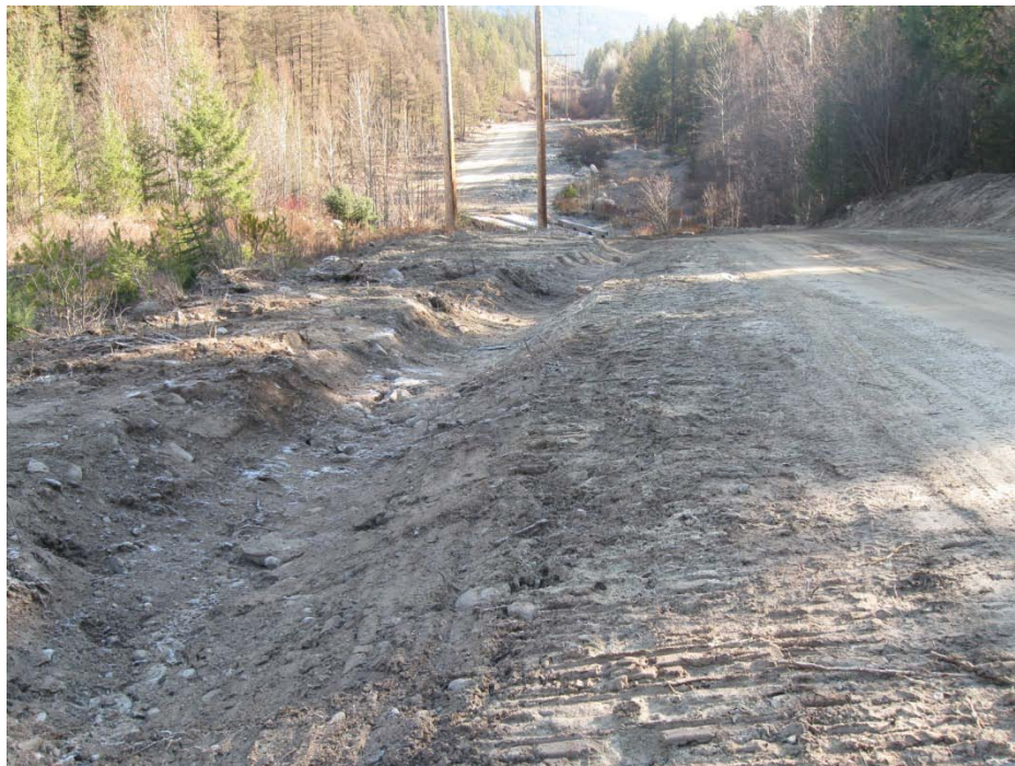
Photo 64 – Trepanier Creek Crossing – recent ditches draining directly to creek (T-5)
