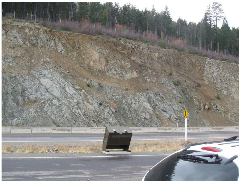
Photo 86 – Large exposed cuts on Highway 97C (T-34)
