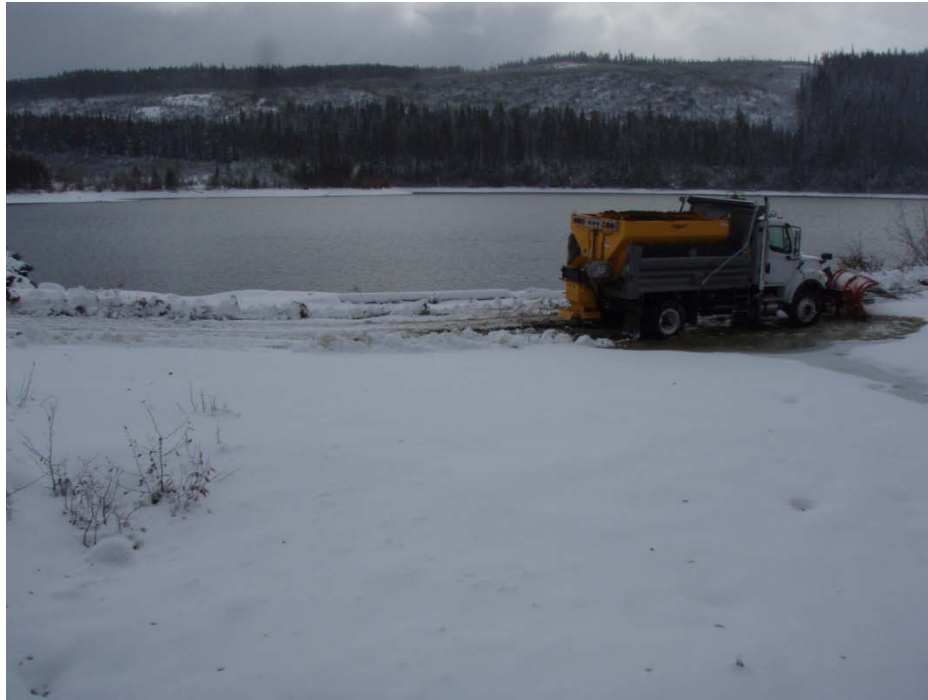
Photo 49 – Road crossing spillway (P-28)
