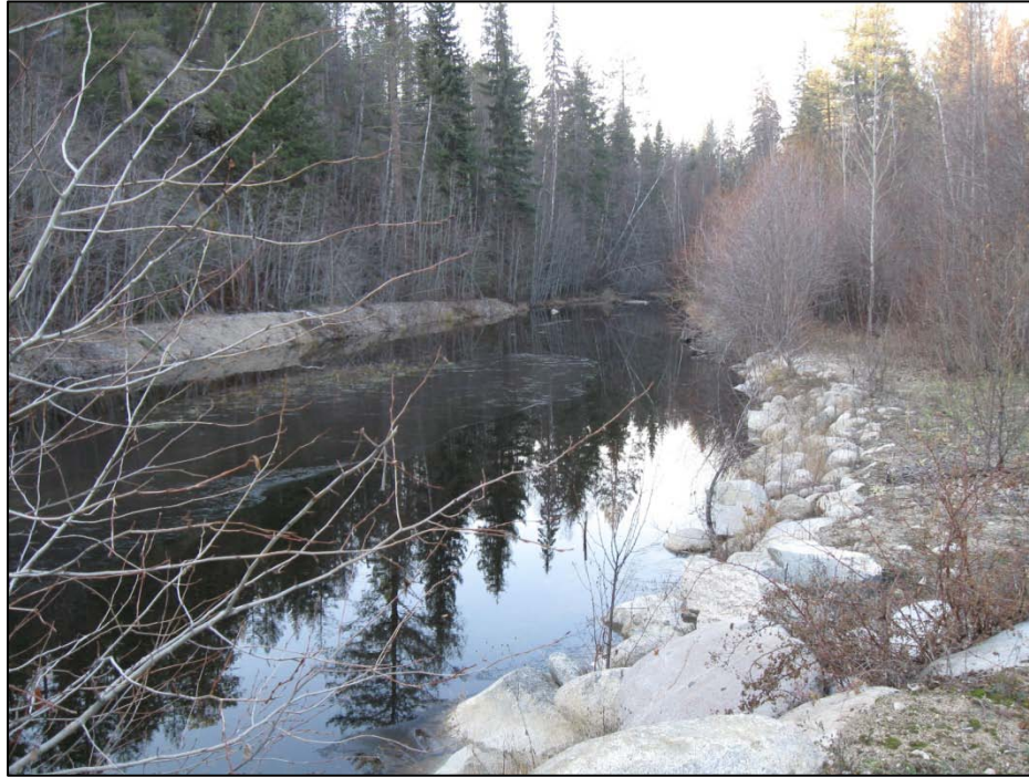
Photo 15 – Trepanier Creek at intake pipes, looking upstream (northwest)
