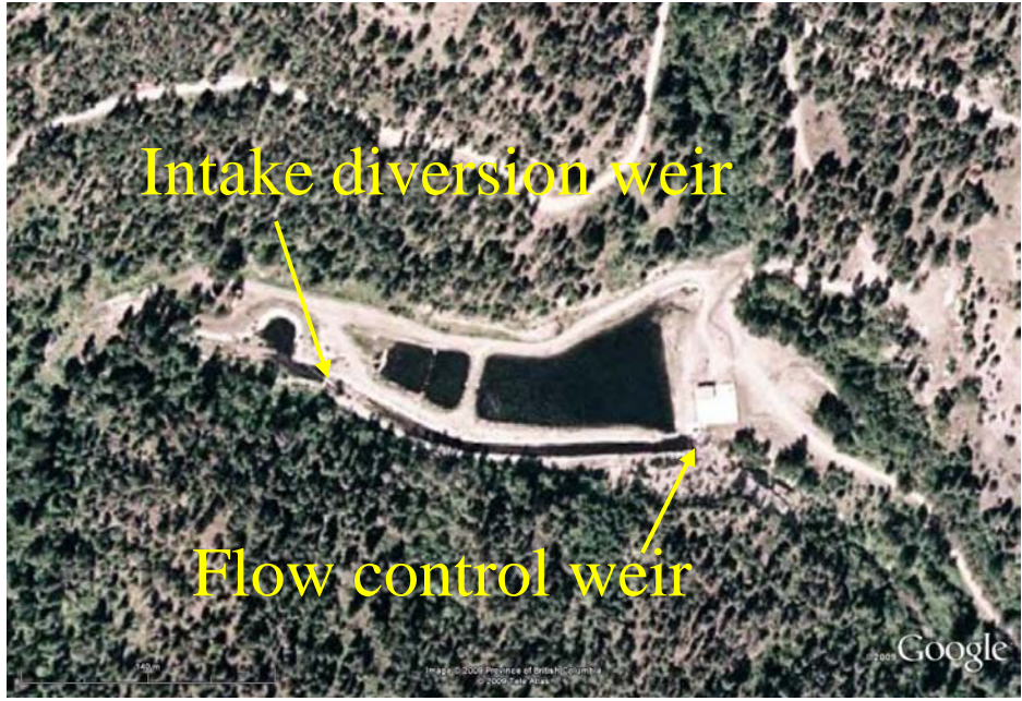
Photo 1 – Peachland Creek Intake Facility
