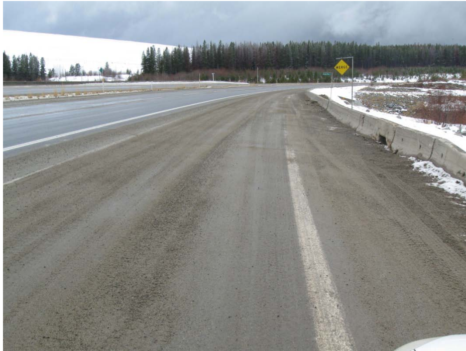
Photo 81 – General winter road condition of Highway 97C – sand and salt application to surface (T-23)
