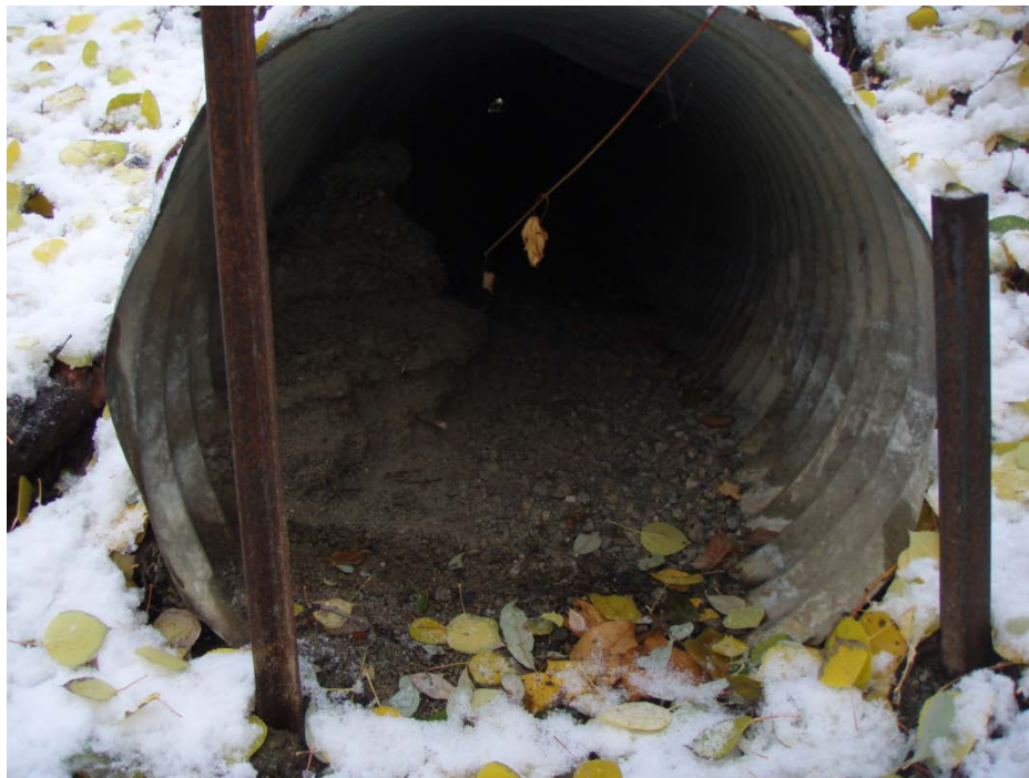
Photo 44 – Slope Peachland Creek –downstream—flow control-- weir
