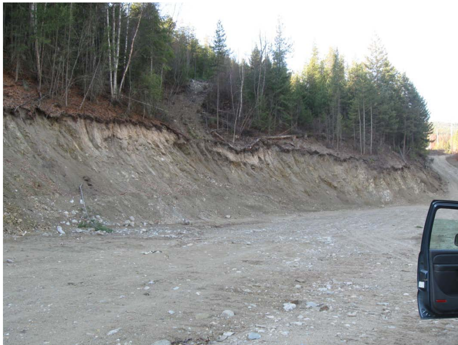
Photo 68 – Eroding cutbanks on newly created road to gravel pit (T-7)
