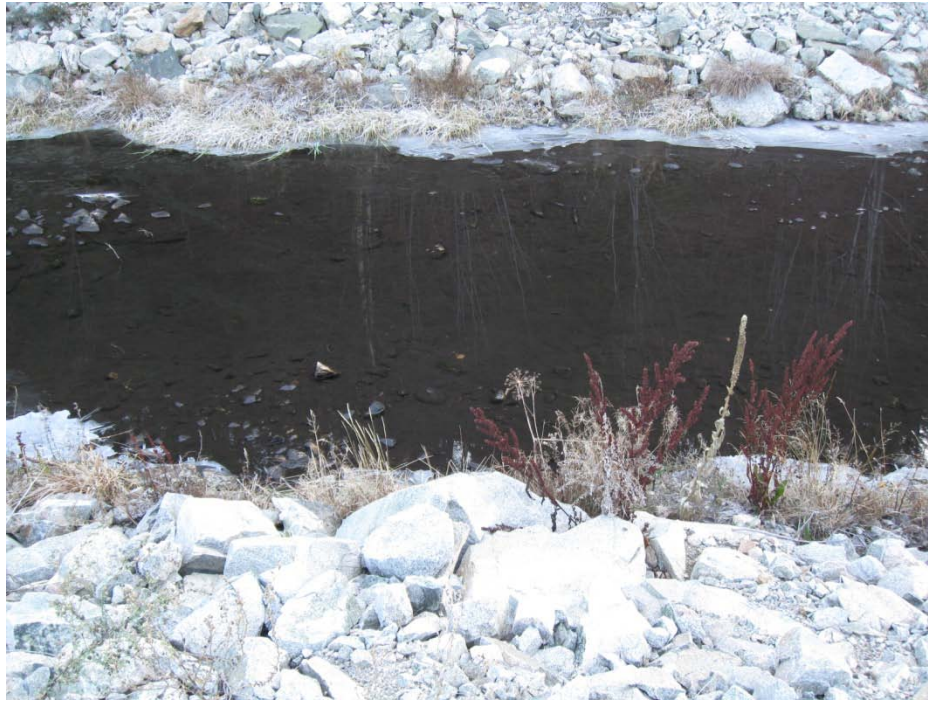
Photo 7 – Sedimentation in Peachland Creek between the Intake weir and the flow control weir
