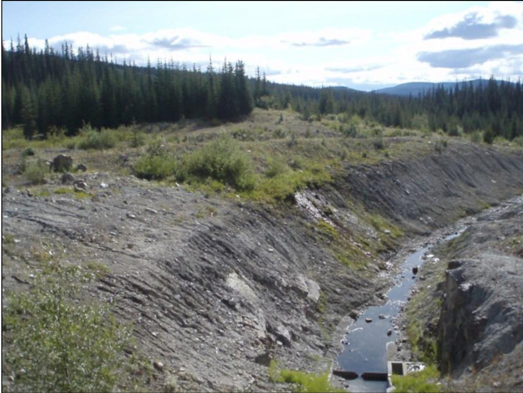
**Photo 3 – Diversion channel from Tadpole Reservoir to Dobbin Reservoir**
