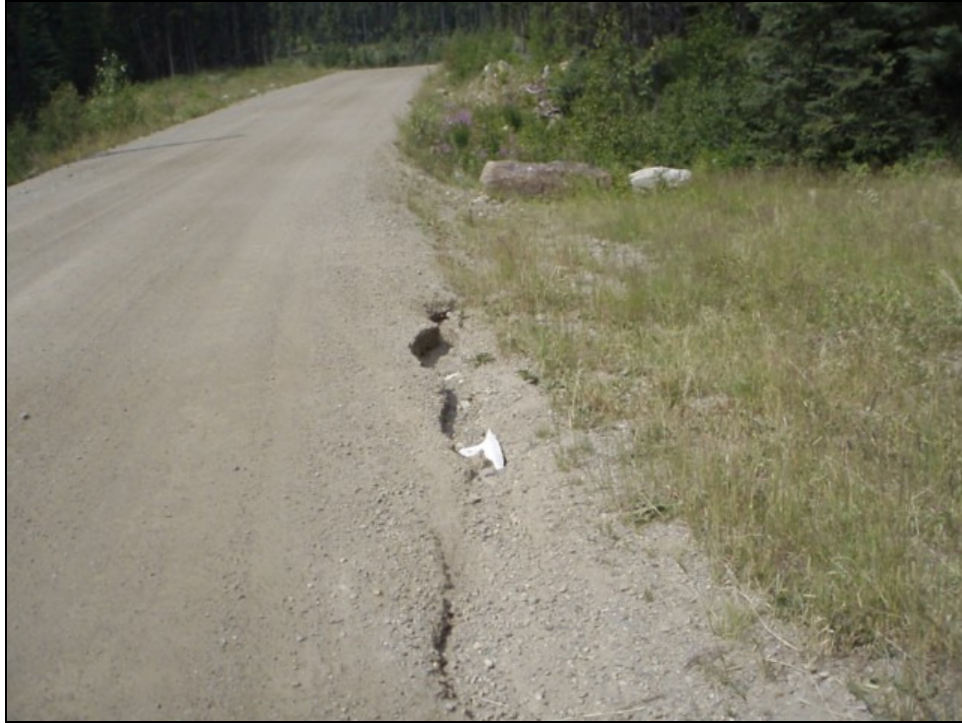
Photo 17 – Running surface erosion to Bulman Creek at Postill Lake Road, Site 9
