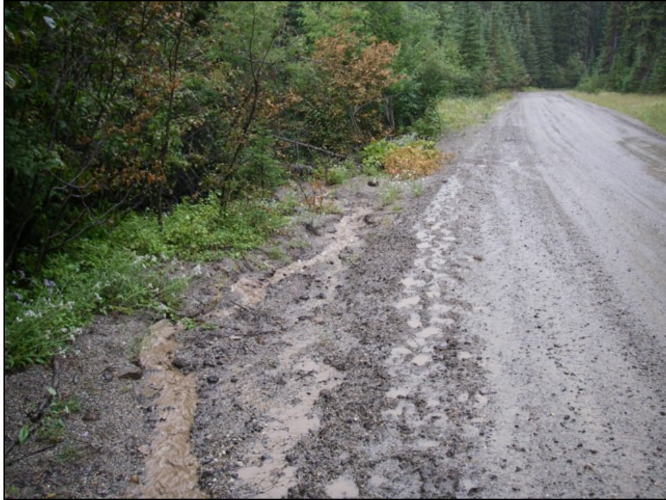
Photo 13 – Running surface erosion along Postill Lake Road during rain
