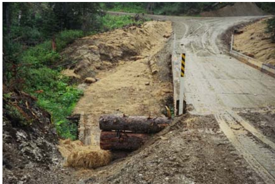
Figure 2. Hay mulch used effectively for both erosion and sediment control.
