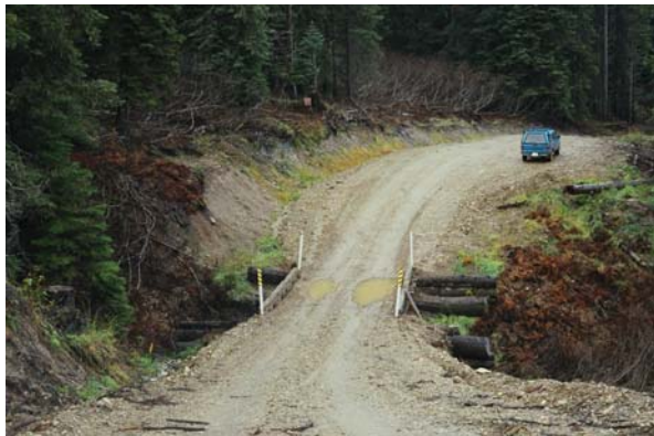
Figure 1. Ditches, road surfaces and cut/fill slopes can be significant sources of sediment at stream crossings.
