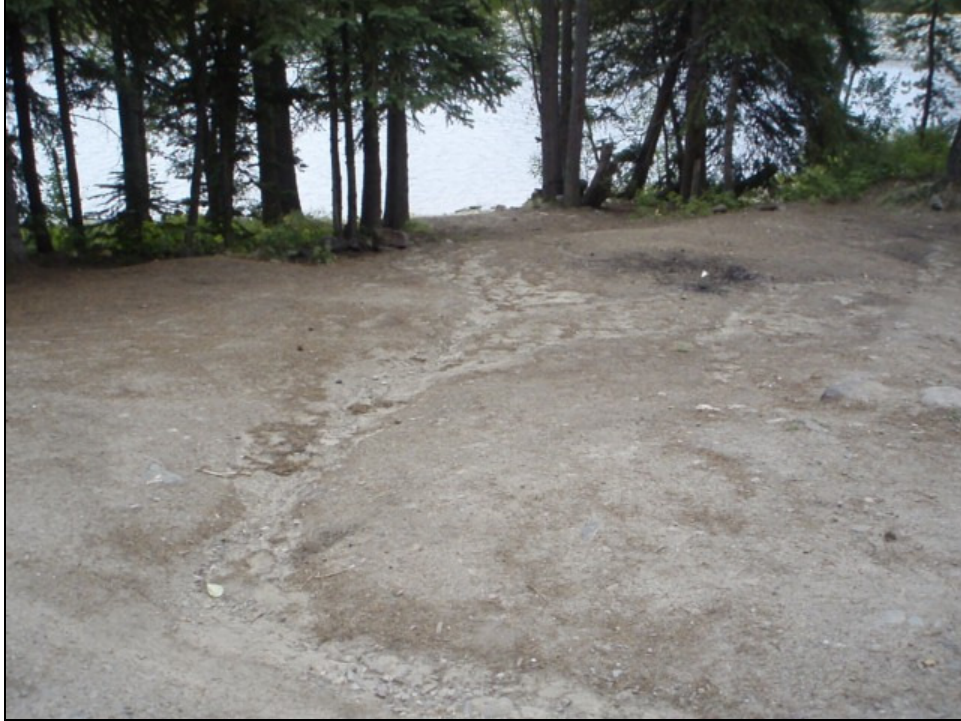
Photo 9 - Recreation site on Postill Lake showing surface erosion at boat launch
