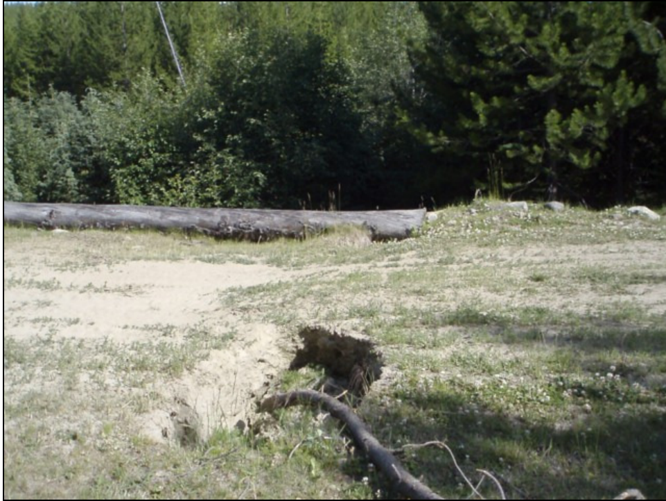
Photo 15 – Failing wood culvert upstream of Hereron Lake, Site 57
