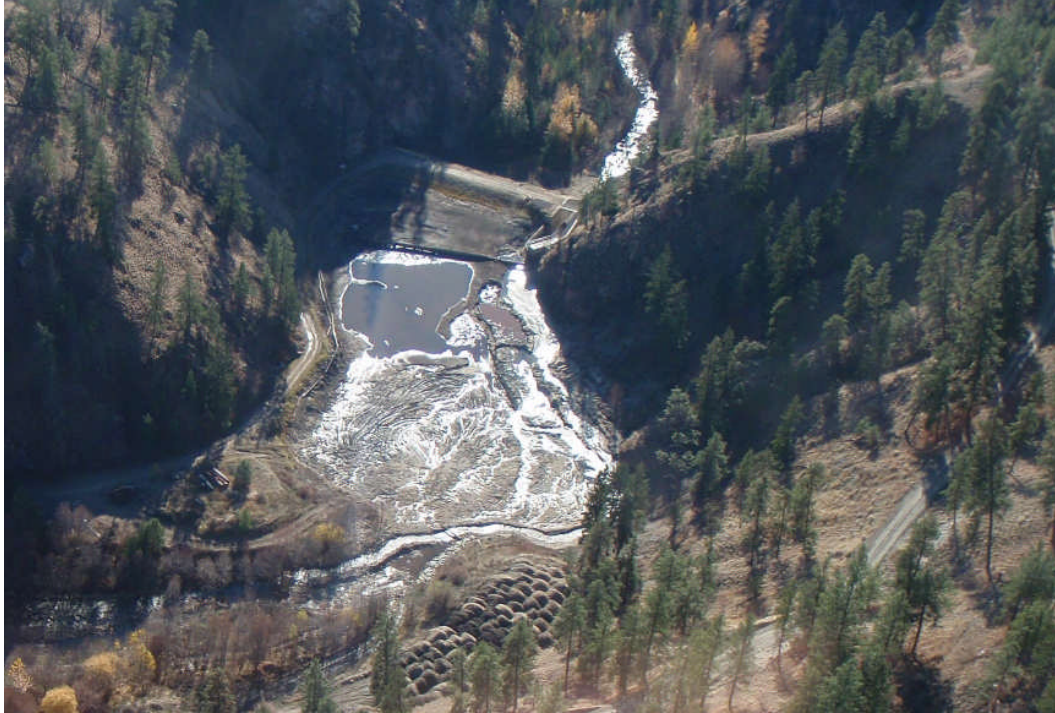
Photo 7. Intake reservoir for Campbell Mtn. irrigation diversion on Penticton Creek mainstem, largely emptied for maintenance and likely for removal of accumulated sediment from behind dam, which is stored to right of stream.
