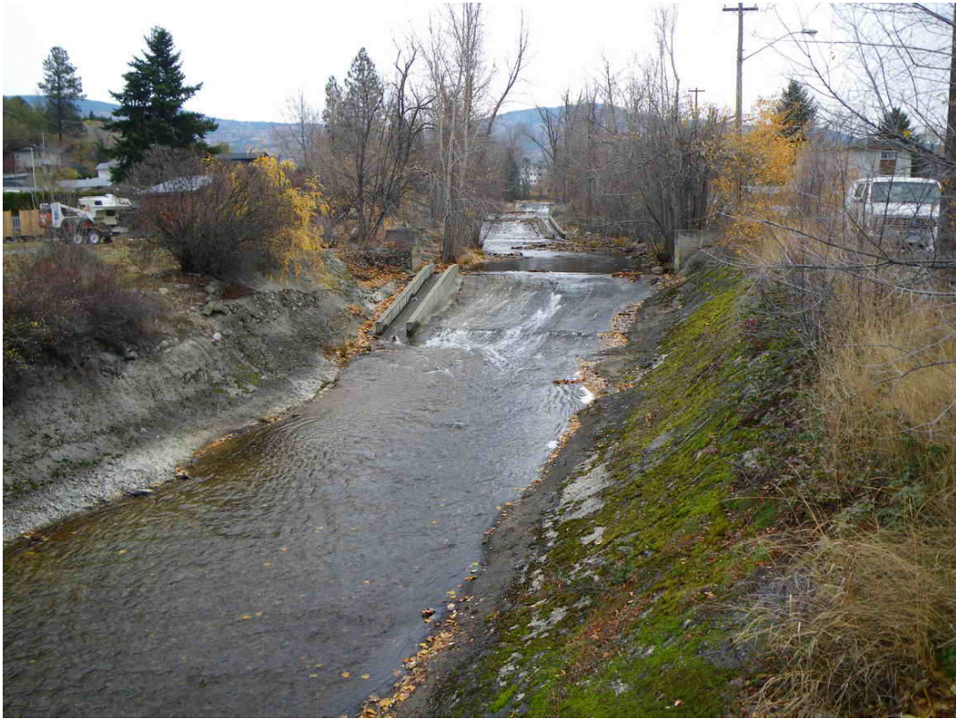
Photo 9. Concrete grade controls and channelization on the Penticton Creek fan.
