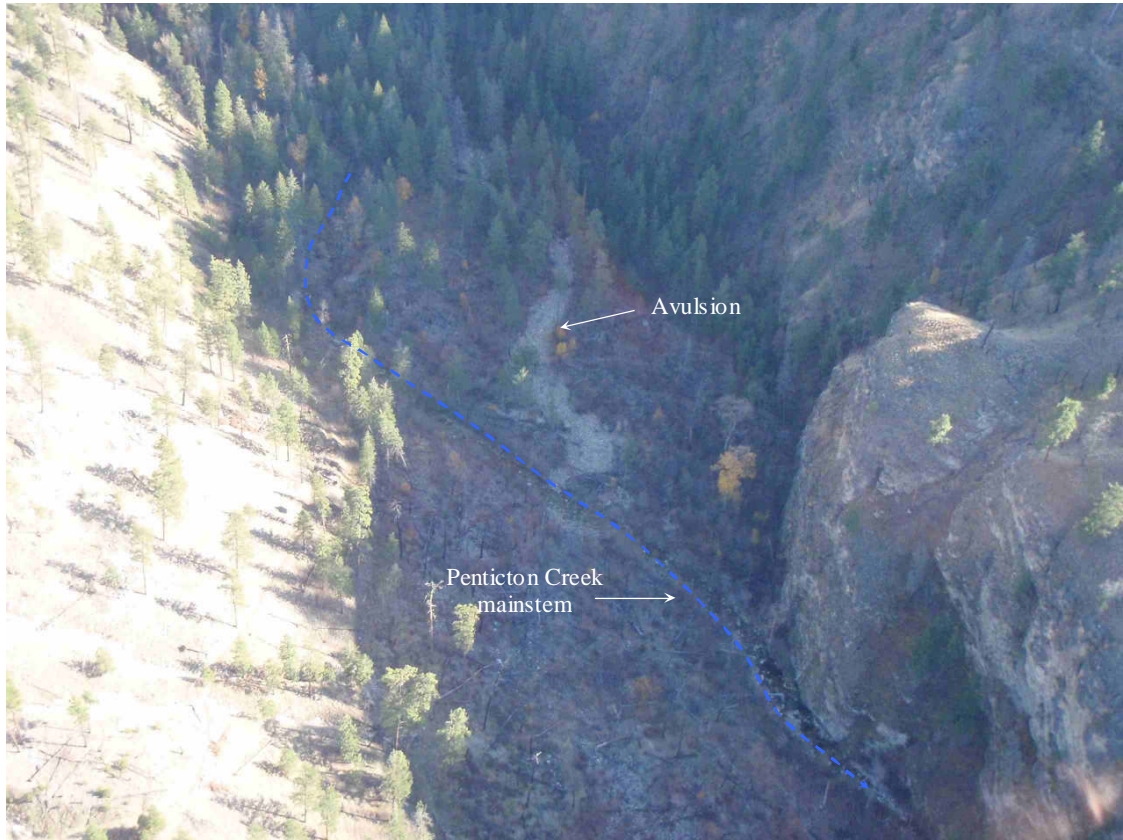
Photo 6. Penticton Creek channel avulsion on narrow floodplain in deeply incised reach upstream of Campbell Mountain Irrigation diversion reservoir. Note bedrock control on left bank.
