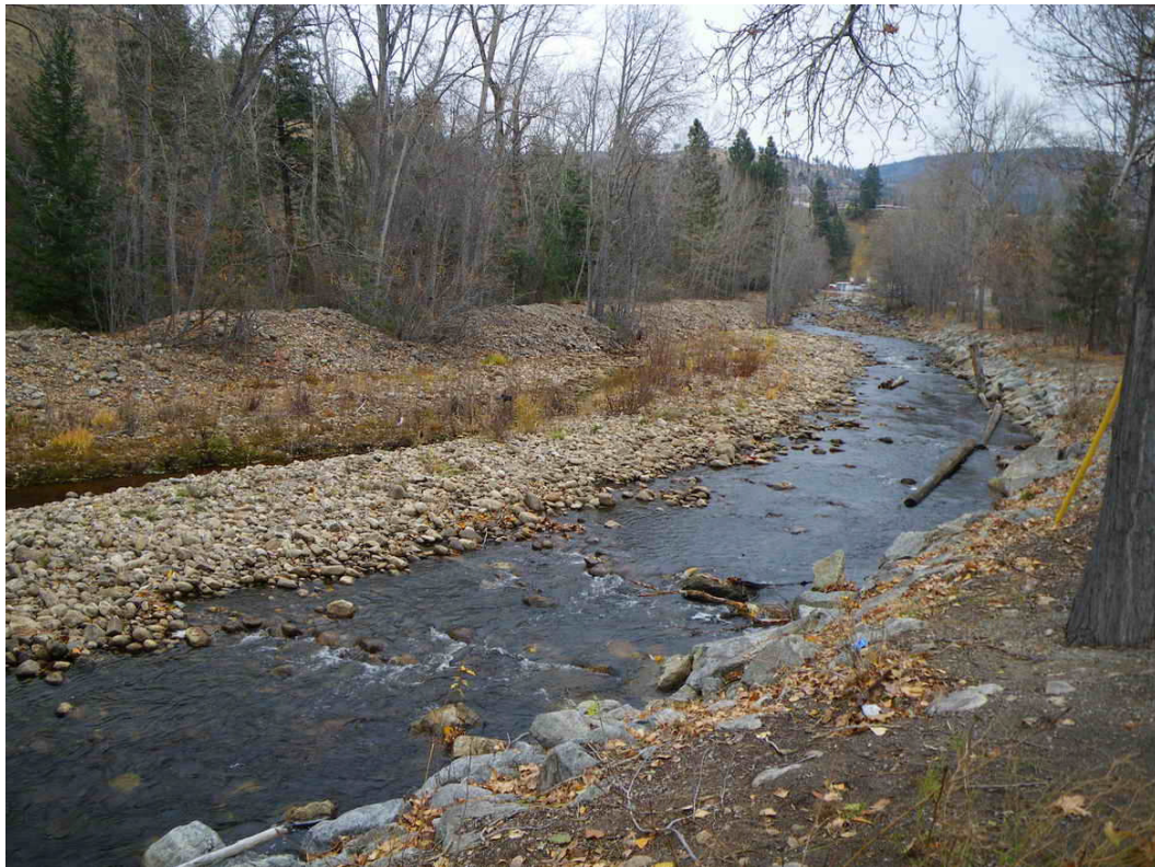
Photo 8. Channelized Penticton Creek on fan. Note dredged sediment stored on left bank.
