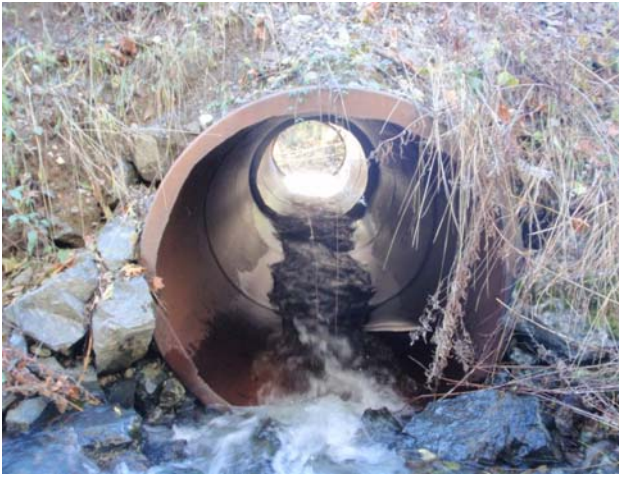
Figure 1: Inlet of a barrier culvert
