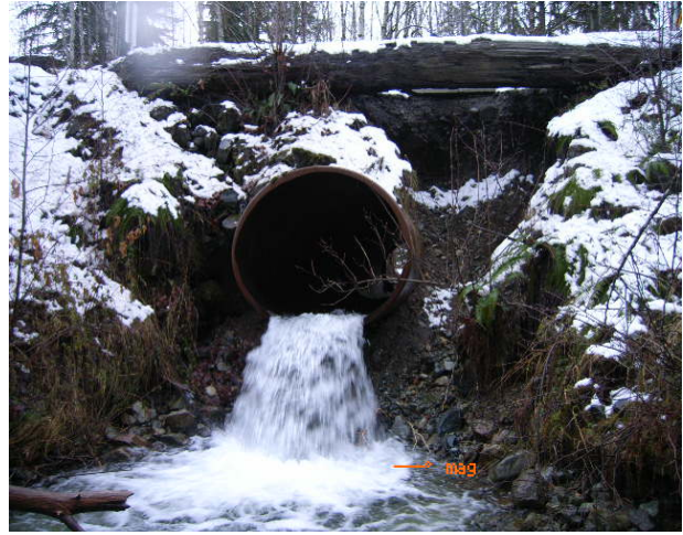
Figure 2: Outlet of a barrier culvert
