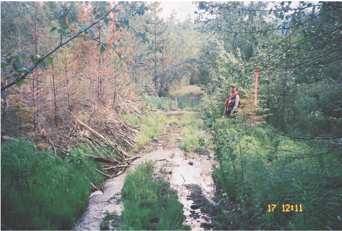
Site 25/1718 : Flow along road surface. Crew person standing above culvert outlet.
