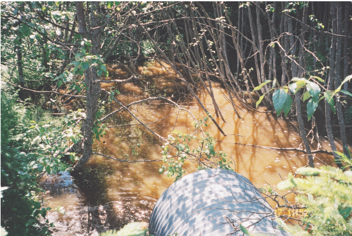
Site 25/1718 : Outlet downstream view.
