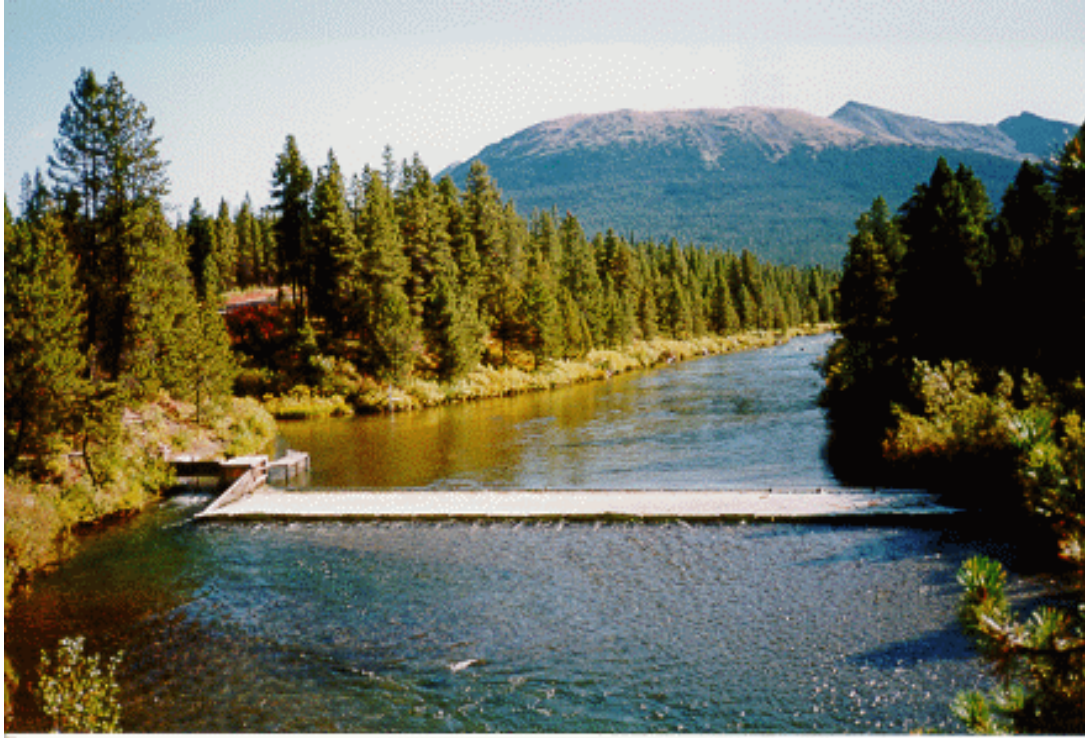
Figure 3. The upper Sustut River floating fish enumeration weir, located approximately 500 meters upstream of the Sustut River-Moosevale Creek confluence.
