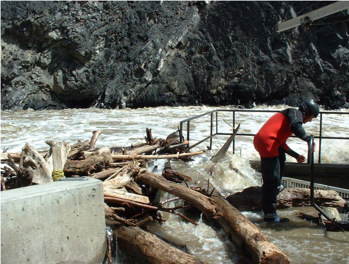
Figure 4. High water flows and debris accumulation at the Bonaparte Fishway, May 27, 2002.
