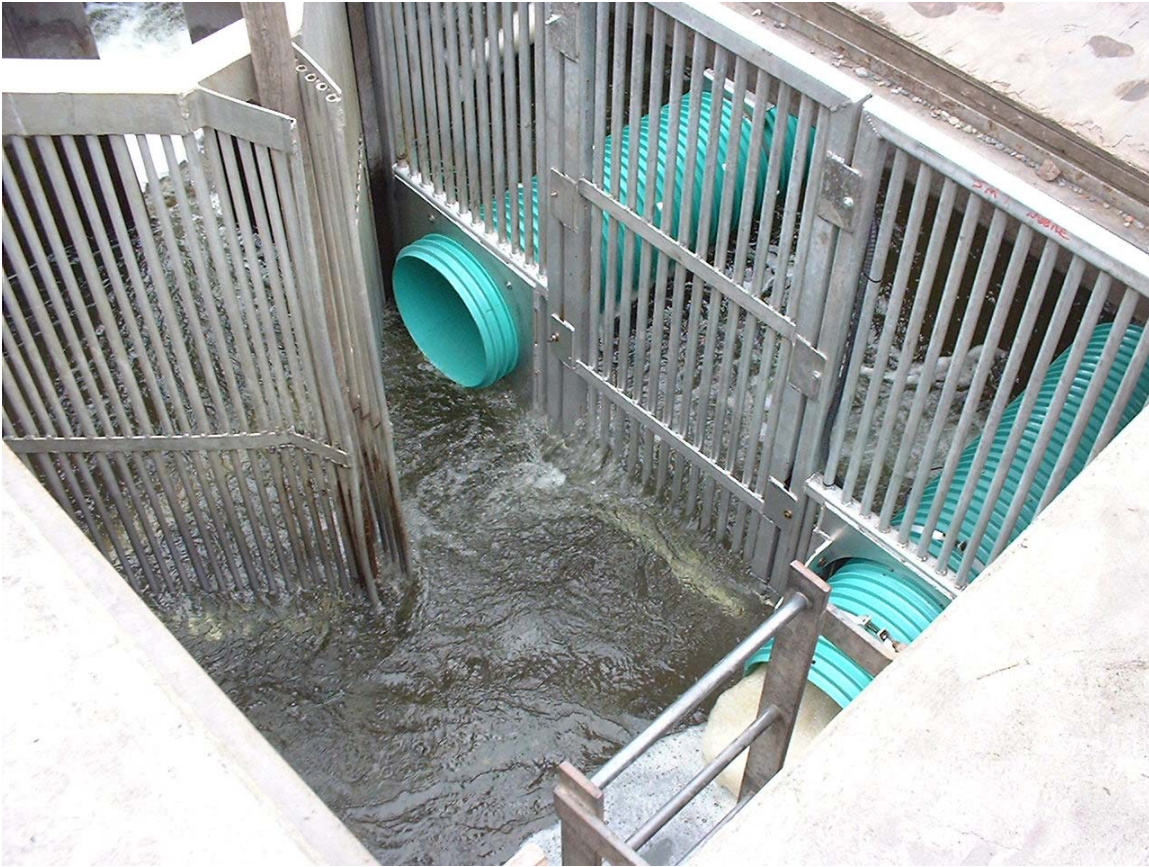
Figure 6. Resistivity counter tubes in the trap cell of the Bonaparte River Fishway.
