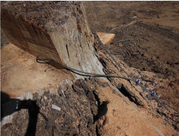
Figure 12. The island was anchored to four stumps with cables and Crosby clips that allow the island to rise and fall with water level changes.
