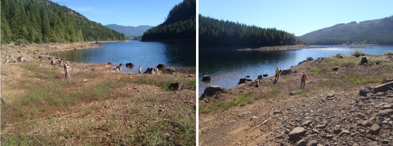
b) View of site looking southeast and southwest.
