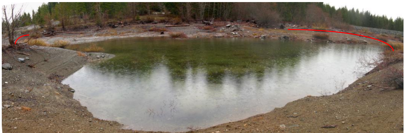
b) View east from existing partial berm.
