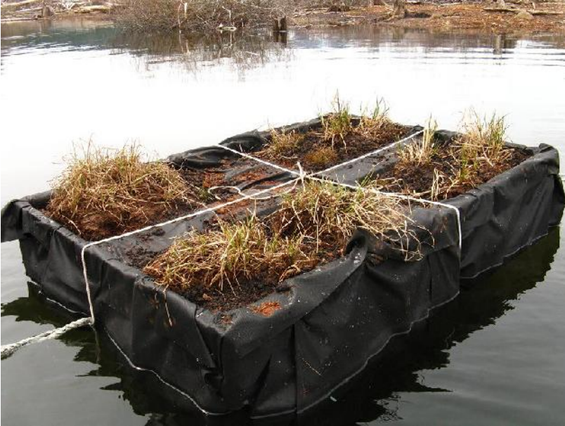
c) Largest island installed and anchored at Elsie Lake, with soil and vegetation added.
