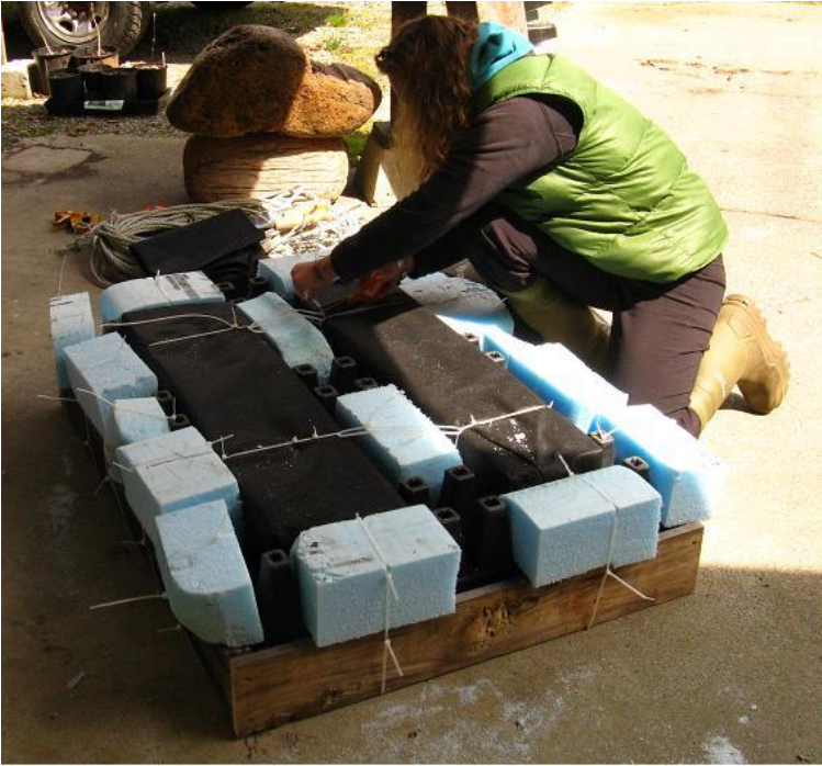
a) Bottom of largest homemade floating island—it was constructed from a plastic pallet, framed by wood, covered with erosion matting, and made buoyant with Styrofoam.
