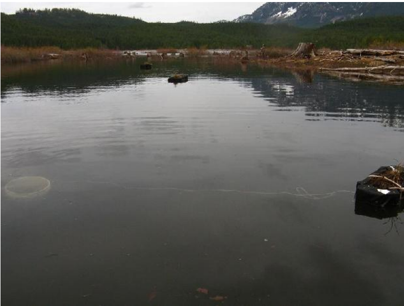
a) Three small vegetation islands made of Styrofoam installed at Elsie Lake (anchoring via rope attached to submerged and weighted bucket).
