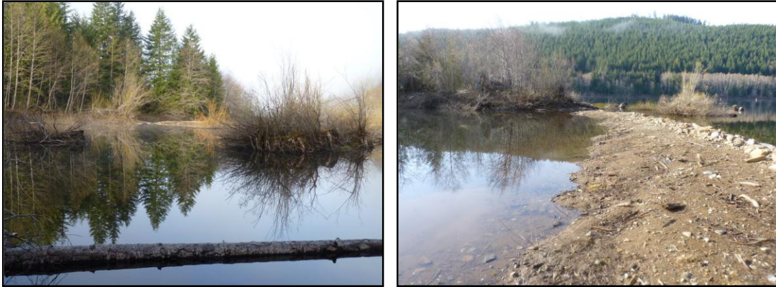
Figure 12: Constructed wetlands at Diversion Reservoir, April 13 th 2011. Photograph on left shows upper wetland; photograph on right shows upper and lower wetlands (left to right), reservoir in distance, and constructed berms.
