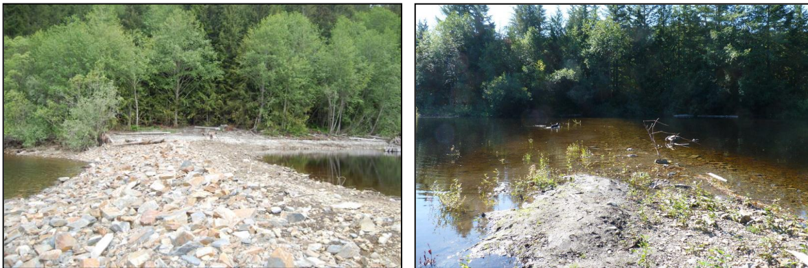
Figure 7: Photographs of middle berm at Diversion Reservoir constructed wetland in May (left) and September (right) 2011.
