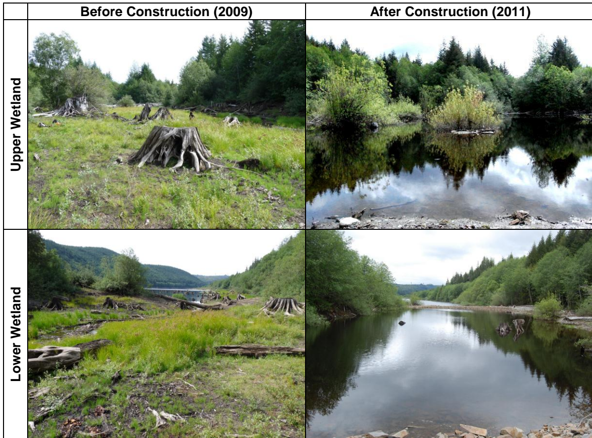
Figure 3: Photographs of wetland site location before and after construction, Diversion Reservoir, Jordon River Watershed, 2009-2011. Photo credits: Virgil Hawkes (2009) and Krysia Tuttle (2011).
