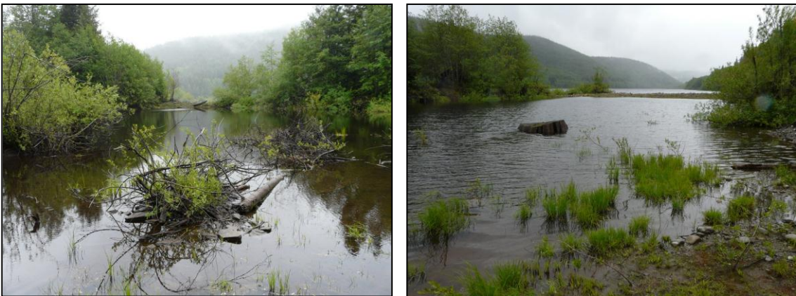
Figure 14: Constructed wetlands at Diversion Reservoir, June 13 th 2011. Photograph on left shows upper wetland; photograph on right shows lower wetland and berm with Diversion Reservoir in the distance.
