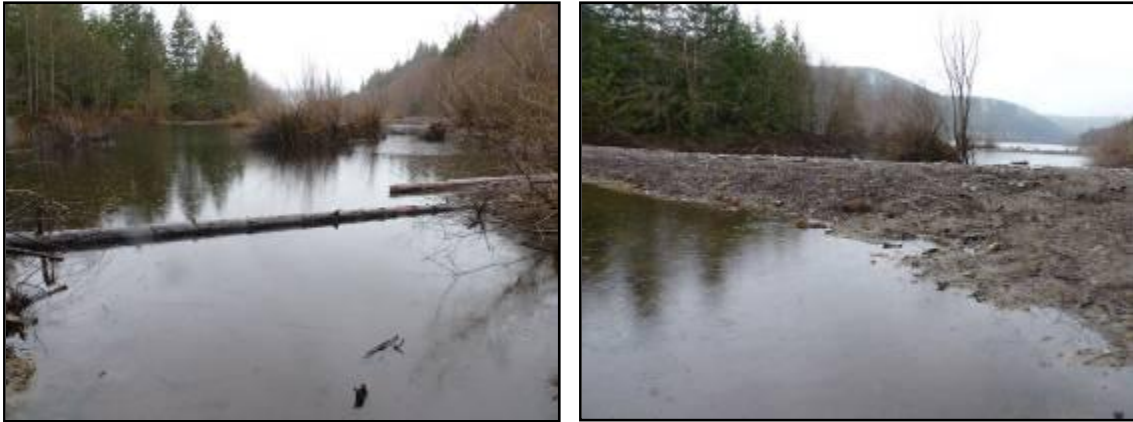
Figure 13: Constructed wetlands at Diversion Reservoir, May 4 th 2011. Photograph on left shows upper wetland; photograph on right shows lower wetland and reservoir (left to right), and constructed berm.
