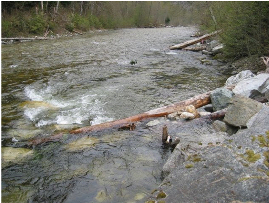
Figure 16: A modified J-hook vane that uses a ballasted log pair instead of boulders for part of the structure. View looking downstream
