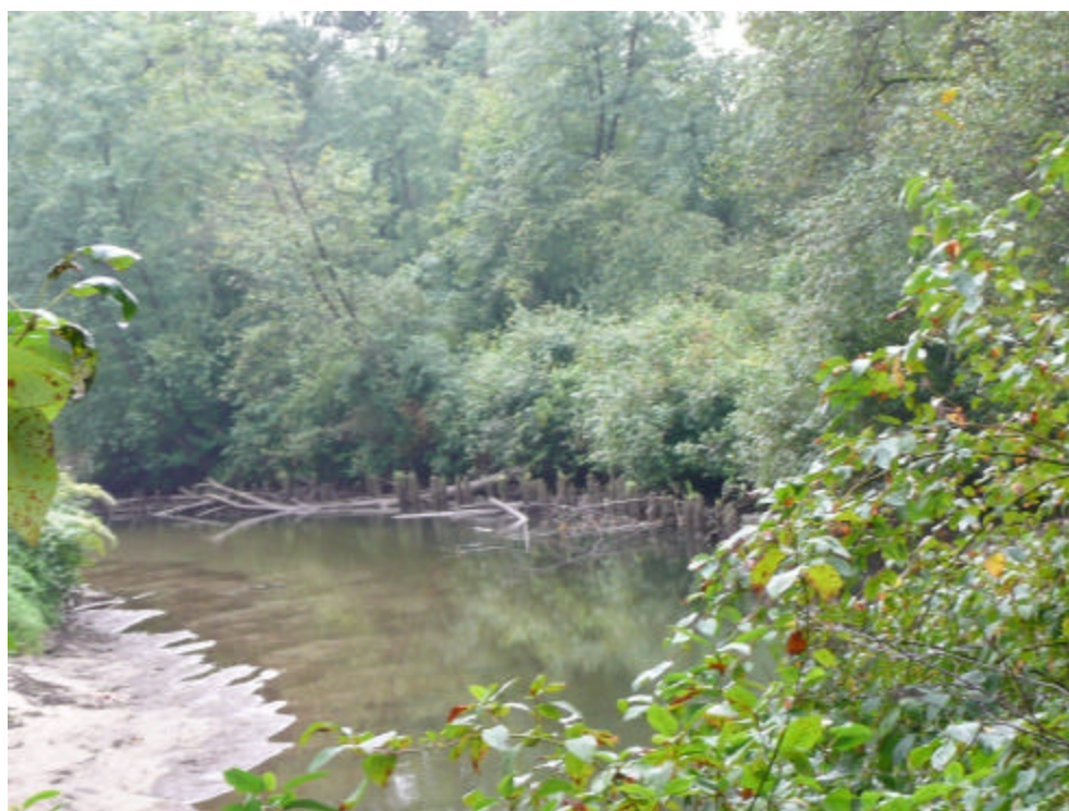
Figure 6: Reach C looking downstream towards historical bank protection works at km 3.75. The bank has eroded significantly from its original location.
