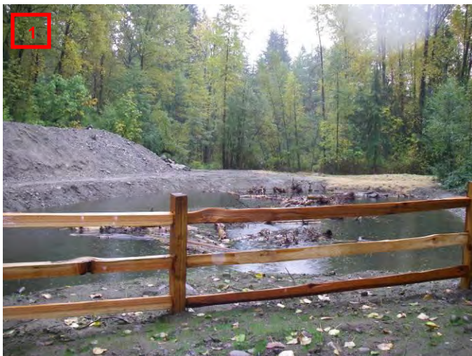
Rearing Pond, Split Rail Cedar Fence During Construction
