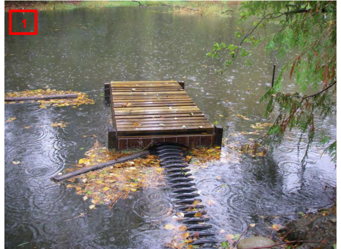
One of Two Beaver Boxes on Culvert Outfall
