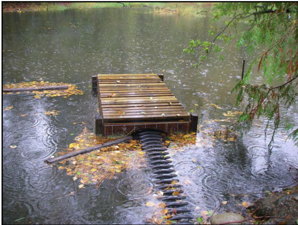
Figure 1 Beaver Baffle Installed on New Culvert
