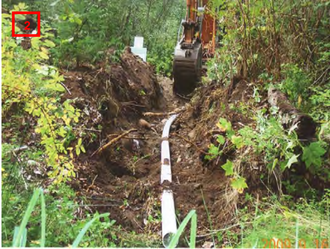
Installing Pipe to Flood Compensation Habitat
