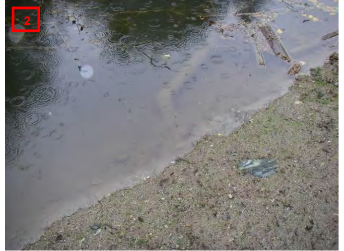
Installed Pipe to Flood Compensation Habitat
