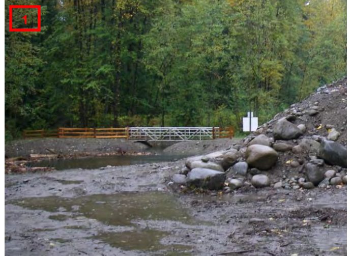
New Foot Bridge, Fencing and Project Sign #2
