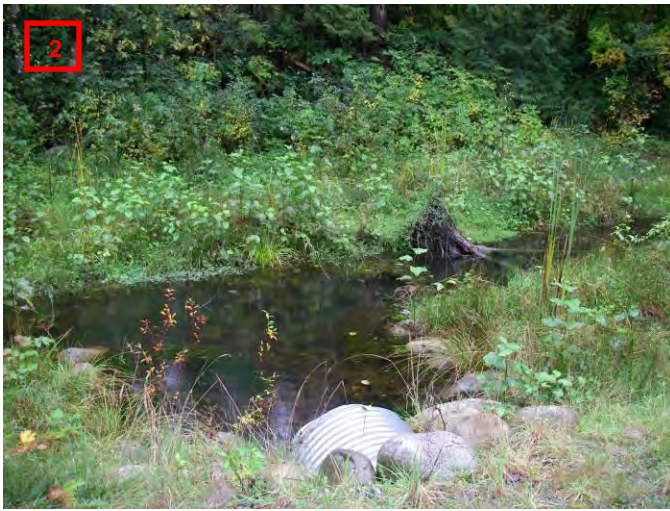
Flooded Habitat, Existing Culvert
