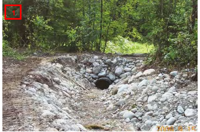
New Spawning Channel During Construction
