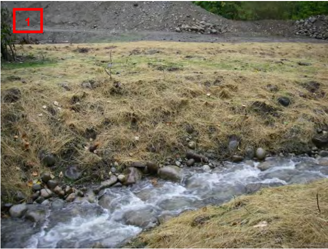
Soil Erosion Protection, Straw and Grasses
