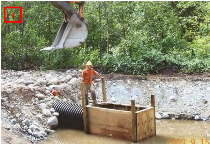
Beaver Box Installation
