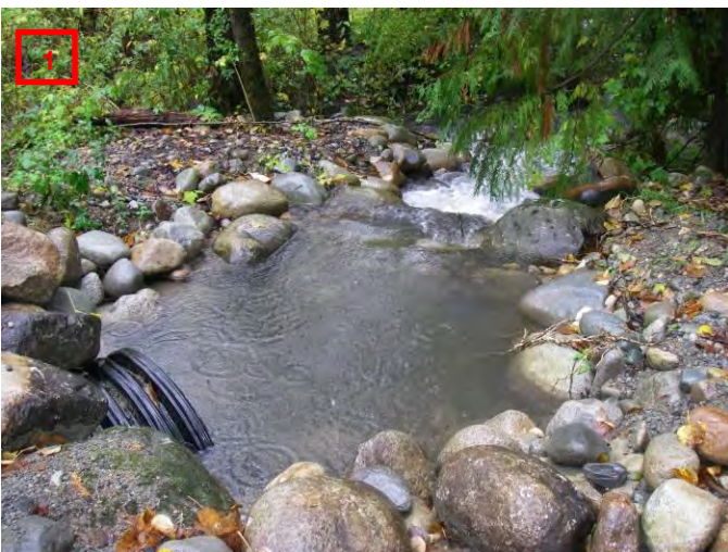
New Culvert, Access to Spawning Channel
