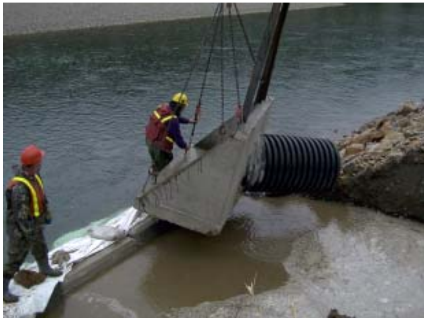
Photo 6 Installation of concrete intake with gate valve was conducted in isolation of the main river flow to control sediment.
