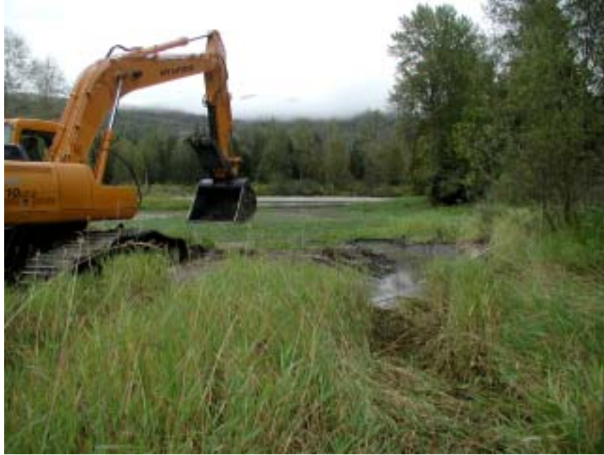
Photo 5 The outlet of the project was very low lying and required minimal excavation to ensure positive outflow. The high point was left till the end of the project to assist with sediment control.
