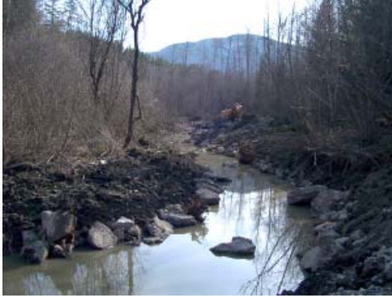
Photo 3 Near completed riffle section, woody material still to be placed. The rock at the toe assists in maintain an open channel by prevent erosion to the toe of the side slope due to spawning fish.
