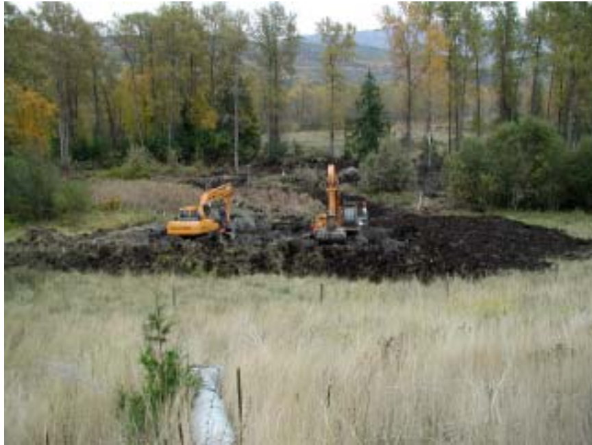
Photo 3 The pipeline for the intake was through a deep cut (up to 5 m). Two machines were used to speed up the installation and clean up process.
