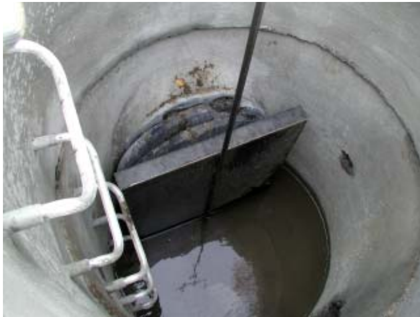
Photo 2 A slide gate was fabricated for the end of the corrugated plastic pipe for controlling the in flow from the Shuswap River. It can be adjusted without entering the man hole casing.
