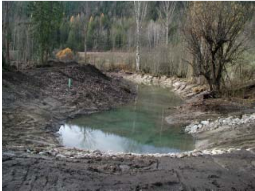
Photo 6 A blind groundwater fed pond was constructed to provide additional groundwater flow and habitat.
