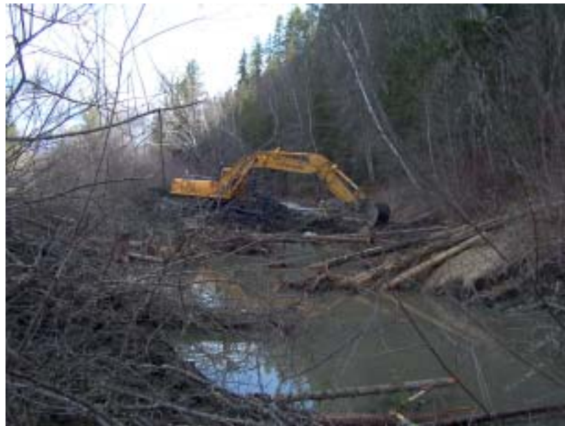
Photo 2 Excavators were used for placing rock and woody material for complexing in excavated pool areas.
