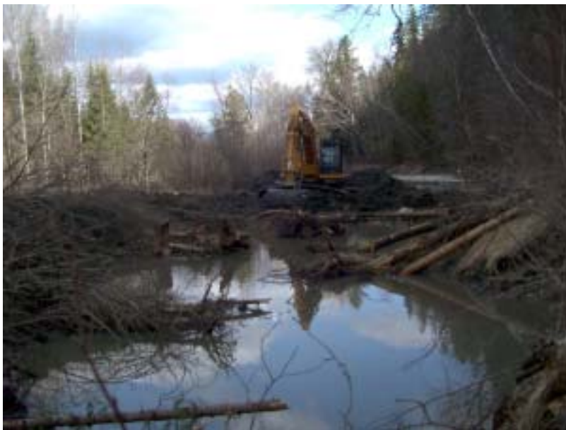
Photo 4 Additional pool habitat was created and complexed with wood.
