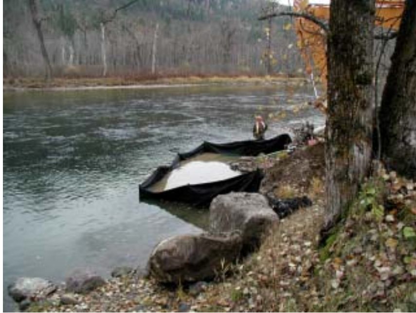
Photo 1 During the installation of the intake, a sediment curtain was used in conjunction with a fish screened pump to control sediment.
