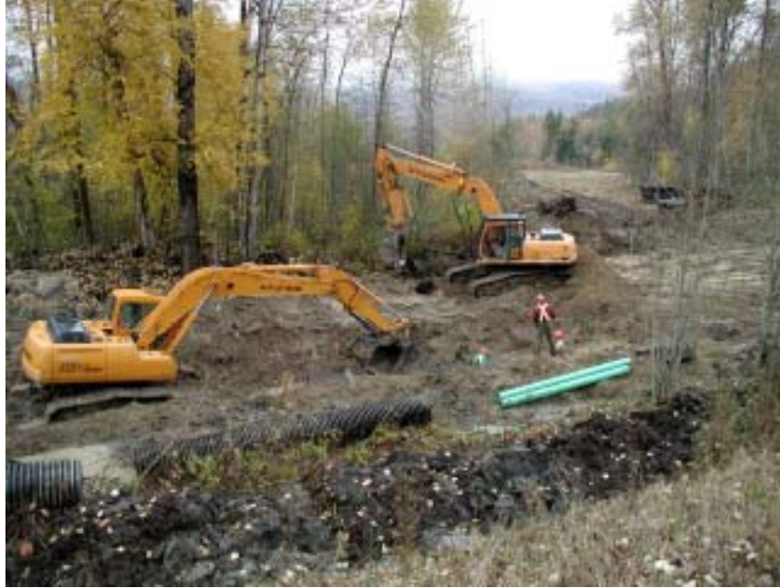
Photo 3 The pipeline for the intake was through a deep cut (up to 5 m). Two machines were used to speed up the installation and clean up process.
