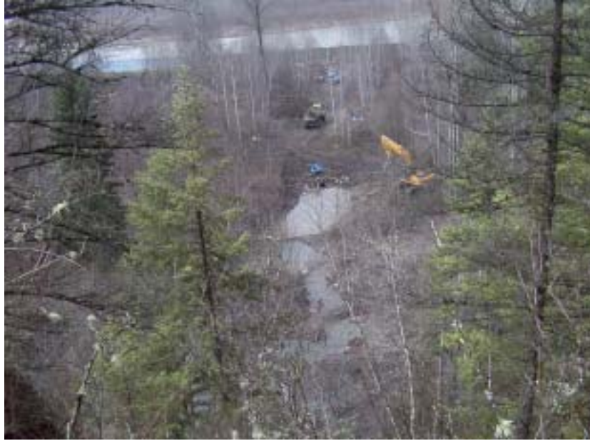
Photo 5 Hillside view of top end of channel with the intake pipe already installed..
