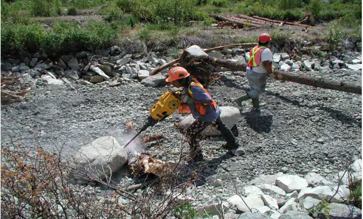
Fred James and John Frank bolting LWD and Rock Down
