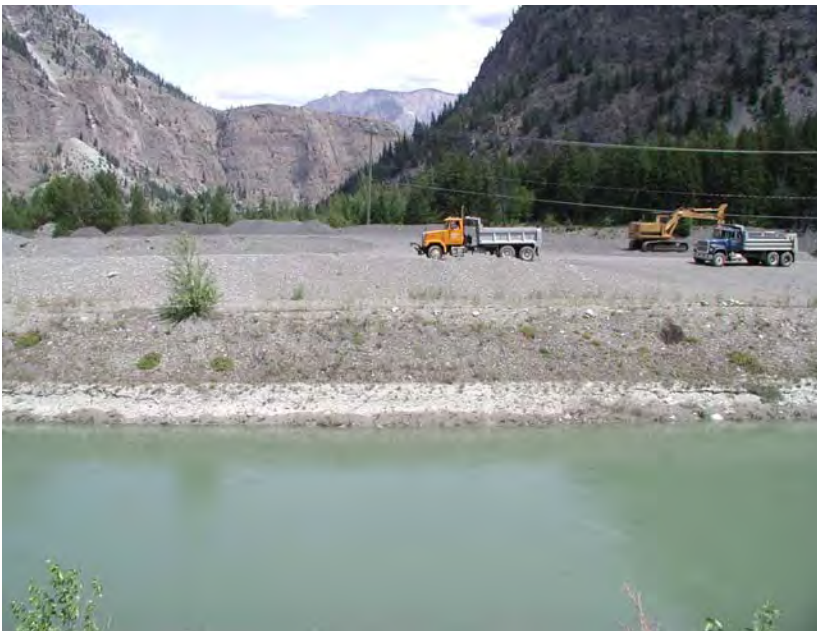
Gravel removed from Aquila site.
