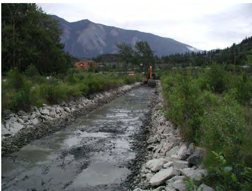
Cobble completely removed from berm
