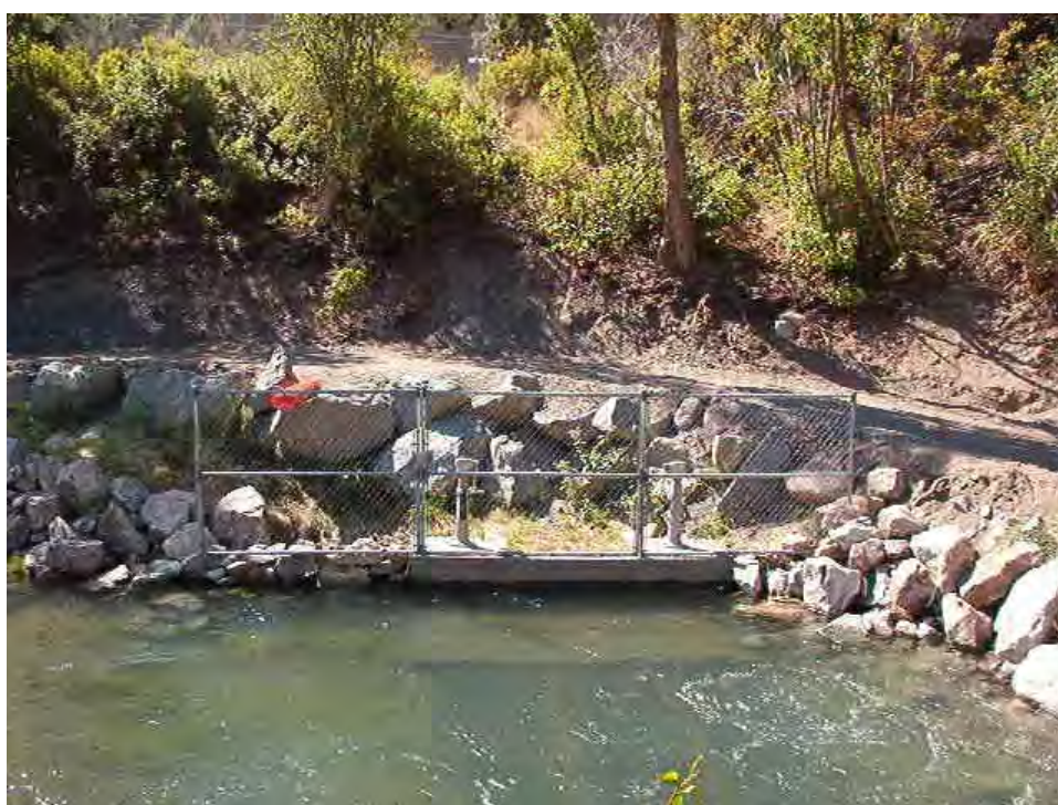
Newly Successful Coho Prevention Fence 2003 with plantings.
