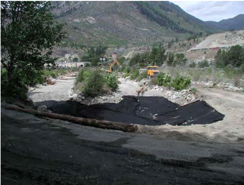
Pool lined with Clay and Geo-textile
