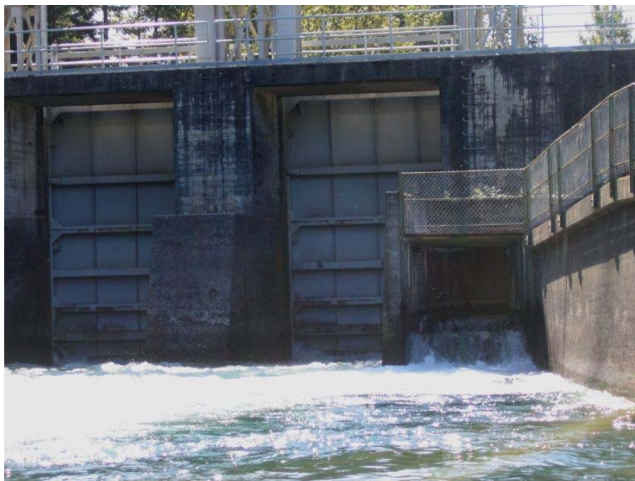
Photo 6. Entrance to fishway showing approximately 35 cms discharge over outlet weir.
