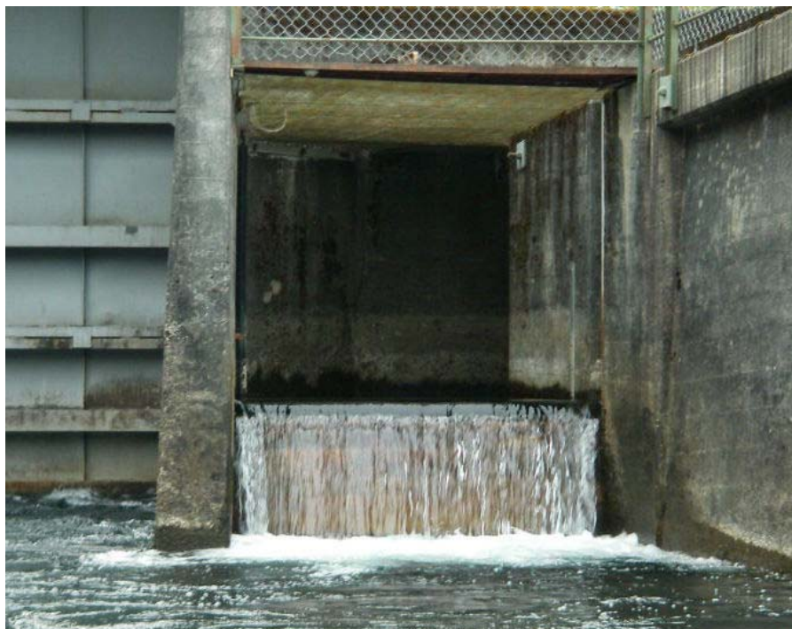
Photo 5. Comox Dam fishway entrance, October 24, 2006. Water level logger located in black PVC pipe on left of fishway outlet. Fishway Q = 0.15 cms (13 cm water flowing over weir).
