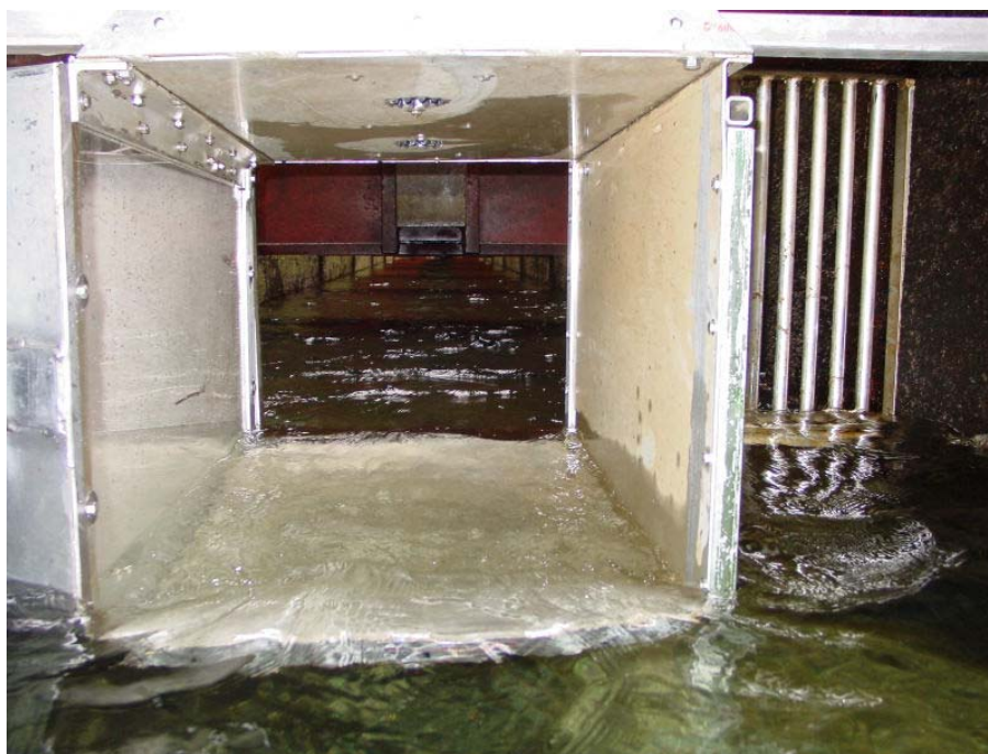
Photo 2. Tunnel assembly in the Comox Lake impoundment dam fishway showing new lighting system (top of tunnel) for improved night recording. Photo looking downstream at (submerged) fishway orifices.
