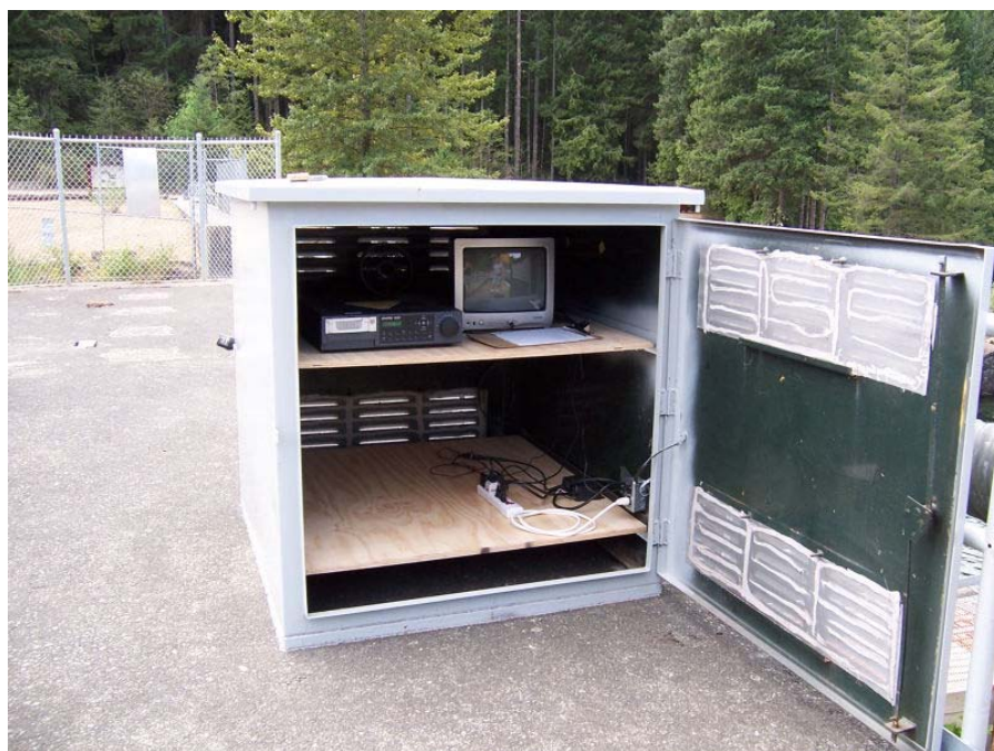
Photo 3. Installation of new protective shelter for DVMS digital recording equipment at Comox Dam, July 2006.
