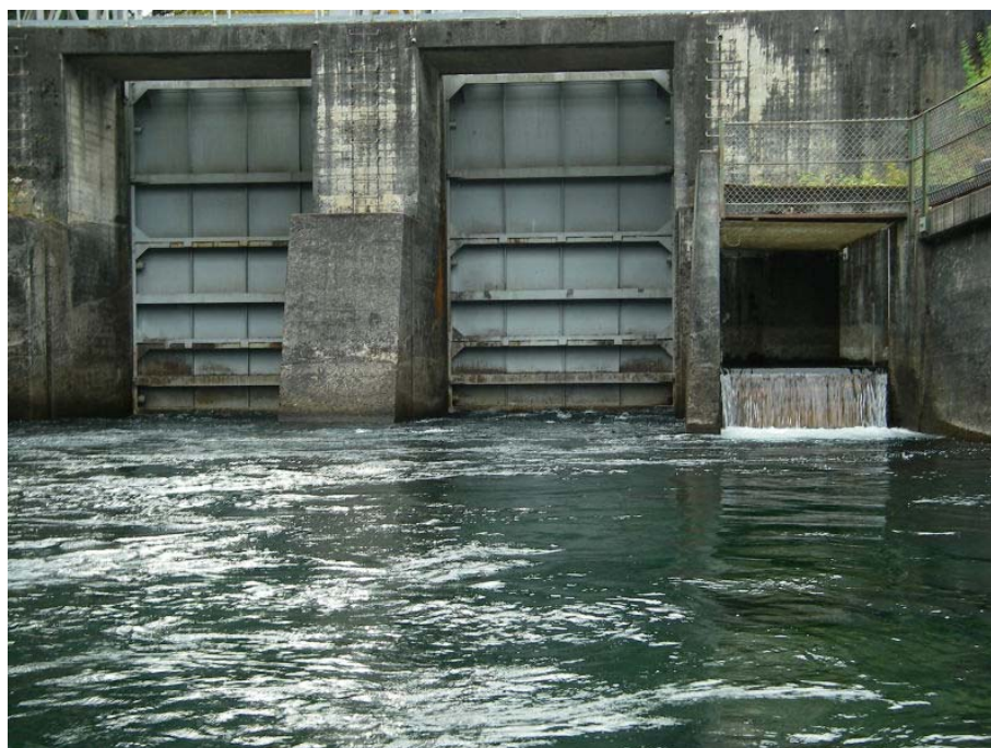
Photo 4. Comox impoundment dam sluice gates and tailrace pool, and fishway entrance, October 24, 2006. Sluice gate Q = 9.1 cms; fishway Q = 0.15 cms.
