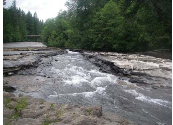
Photo 10. Upstream view of the diversion channel after completion June 19, 2007. Gauge 6 discharge = 7.5 \text{ m}^3/\text{s} .
