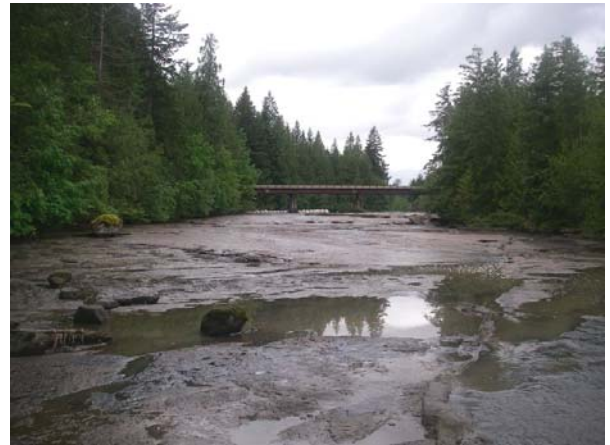
Photo 6. Access route for equipment on right side of river after site isolation measures, June 4, 2007. Cofferdam visible at bridge.
