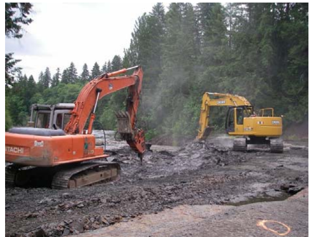
Photo 8. Commencement of channel excavation work looking downstream, June 5, 2007.
