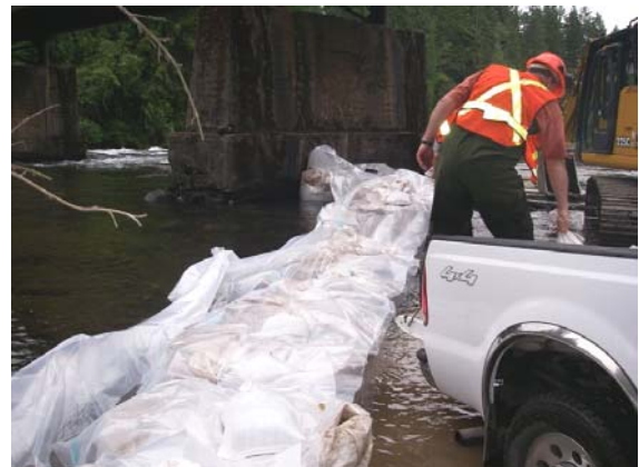
Photo 4. Placement of pre-filled mega bags, plastic sheeting and sandbags for coffer dam construction at upper end of equipment access route.
