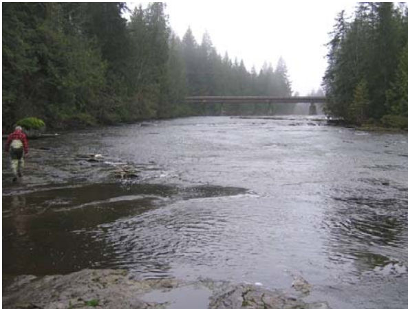
Photo 5. Access route for equipment on right side of river between Duncan Bay Mainline Bridge and work site ~200 m downstream. Photo taken during base flow conditions (5.7 m 3 /s) looking upstream from proposed work site.
