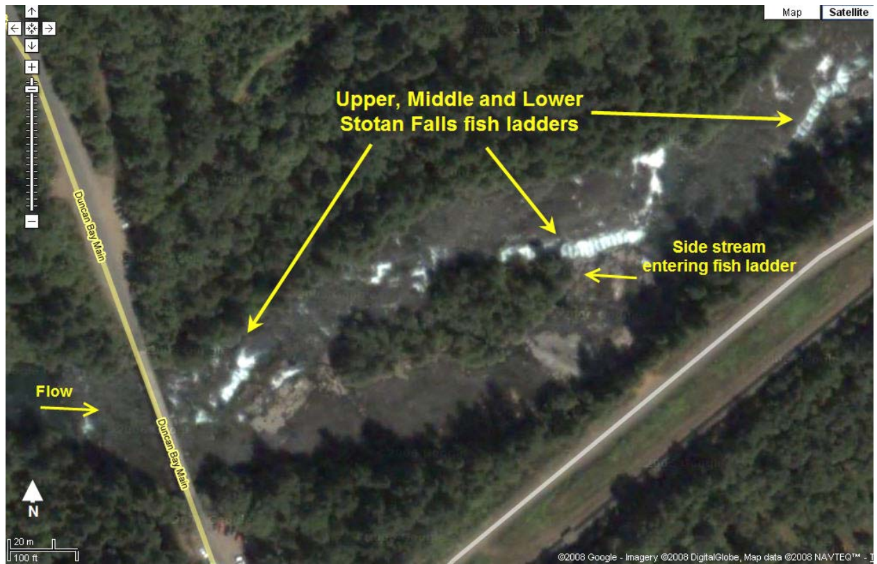
Figure 2. Location of the Stotan Falls area showing fish ladders and location of attraction flow into middle fish ladder.
