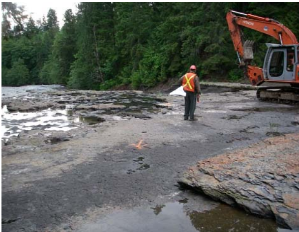
Photo 7. Location of proposed diversion channel looking downstream before excavation work, June 5, 2007.
