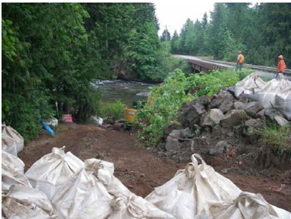
Photo 3. Existing access ramp to Puntledge River located on upstream side of Duncan Bay Mainline Bridge, beside Bevan Creek confluence (left of photo).
