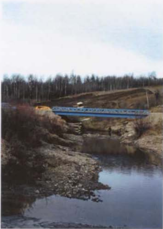
Aitken Creek site 1, below proposed crossing: View upstream; from bottom of site.
