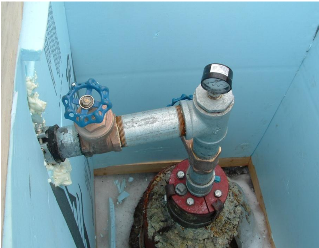
Figure 3. Flowing artesian well brought under control by equipping the well with a flow control device (e.g., cap and valve) to stop the flow with no leakage.
