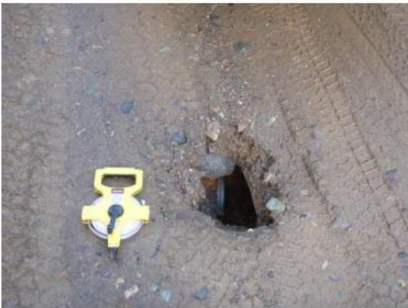
Bull River Road_culvert damage at BULL017
