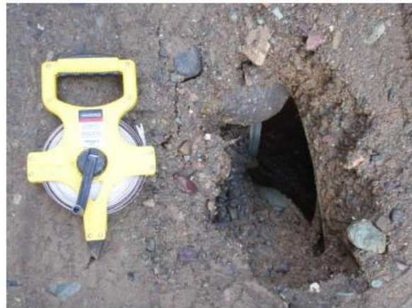
Bull River Road_collapsed culvert damage at BULL017
