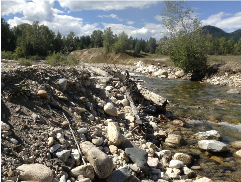
Photo 16. Looking upstream at bank on right where flow from bermed area is eroding bank
