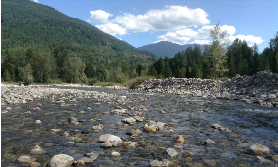
Photo 14. Looking downstream at portion of constructed berm that is contributing sediment and creating scour along opposite bank
