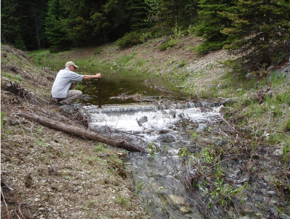
Figure 32. Upstream view of spillway crest at Nicklen Lake outlet on June 20, 2012.
