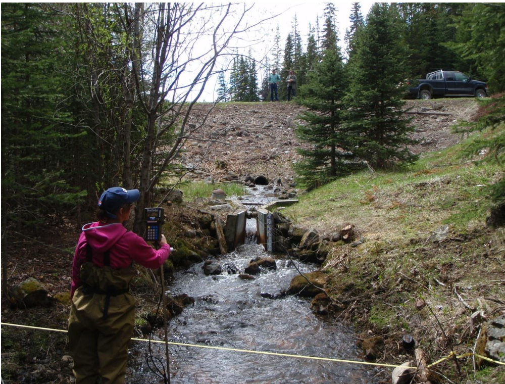
Figure 33. Upstream view of Nicklen Creek with old flume and water release pipe in background taken on May 29, 2013.
