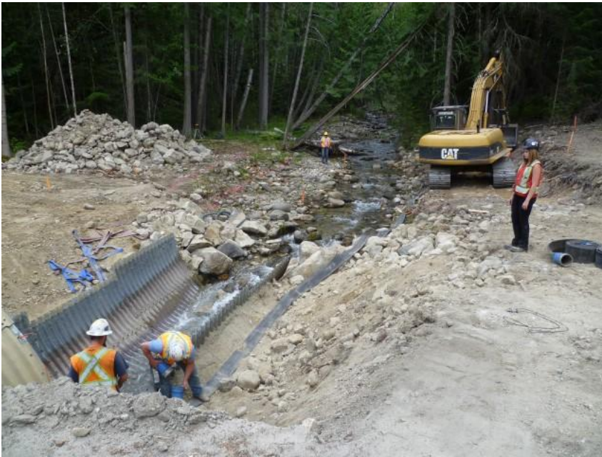
Photo 1 – July 23 – Existing culvert exposed, top have removed
