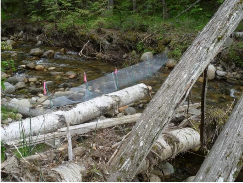
Photo 3 - July 23 – Fish barrier installed upstream of dewatering sump
