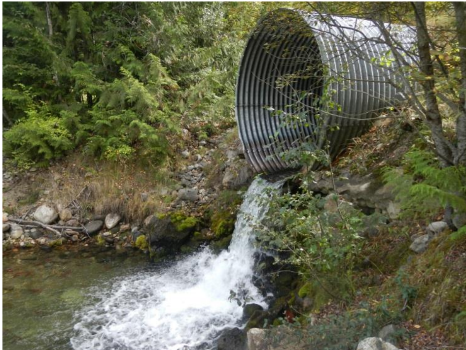
Figure 6. Highway 6 Crossing of Heart Creek (September, 2014)
