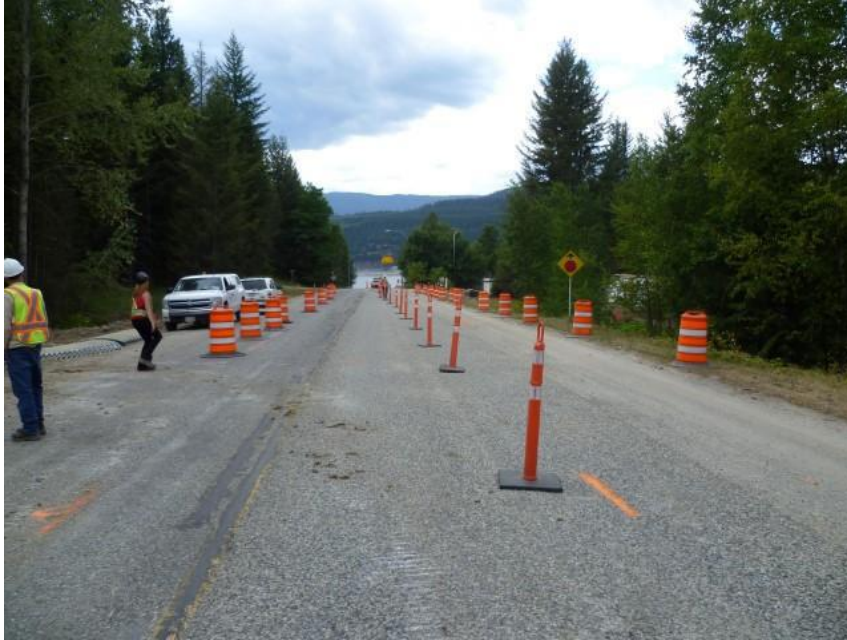
Photo 5 – July 23 – Temporary lane shift, looking west on Hwy
