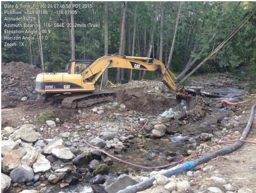
Photo 6 – July 24 – Excavating for riprap placement south of Hwy on east side of creek
