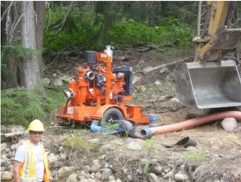
Photo 2 – July 23 - 6 inch water pump being installed under the supervision of the Environmental Monitor
