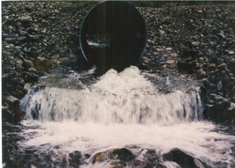
Figure 1. Culvert under Highway 6 – August 1978
