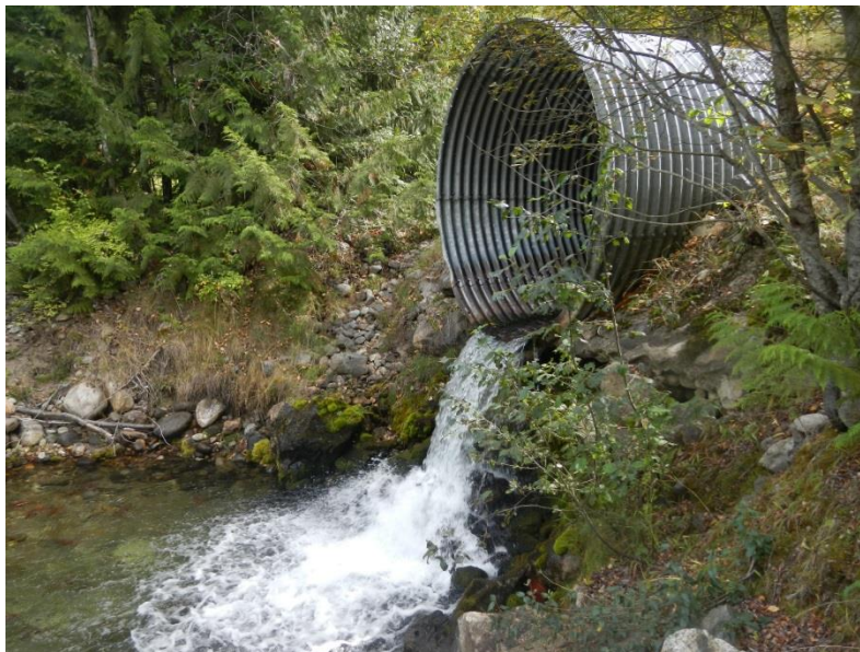
Figure 2. Culvert under Highway 6 – September 2014
