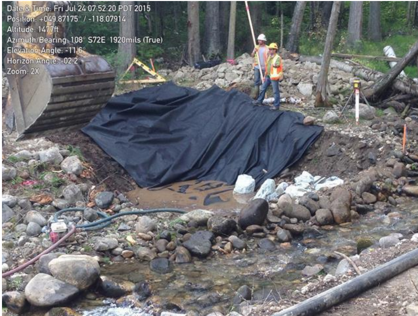
Photo 7 – July 24 – Riprap excavation lined with geotextile and starting placement of 500kg riprap
