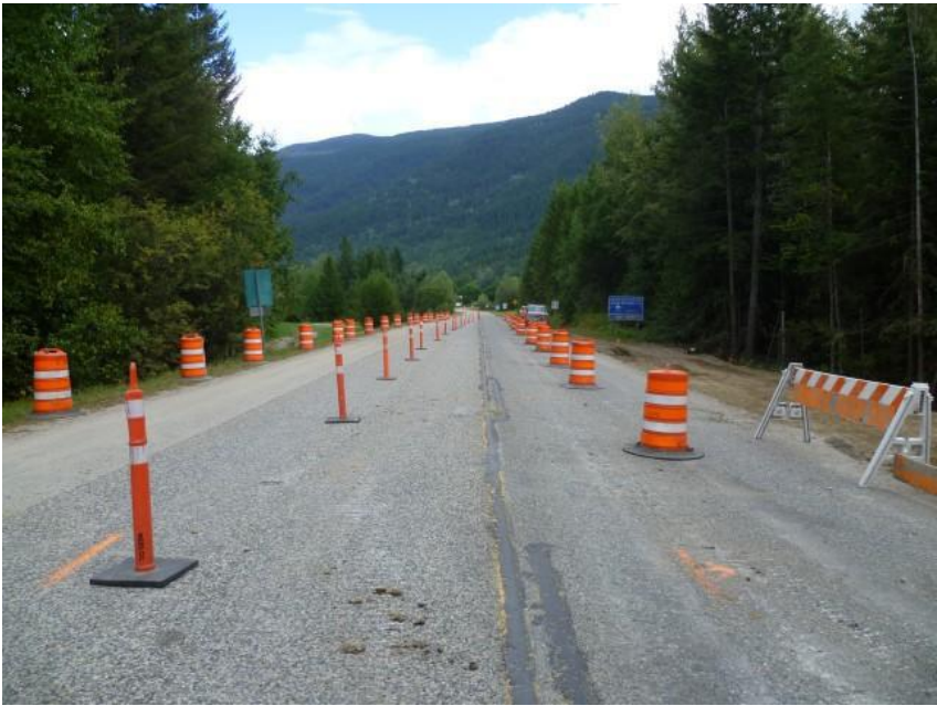
Photo 4 – July 23 – Temporary lane shift, looking east on Hwy
