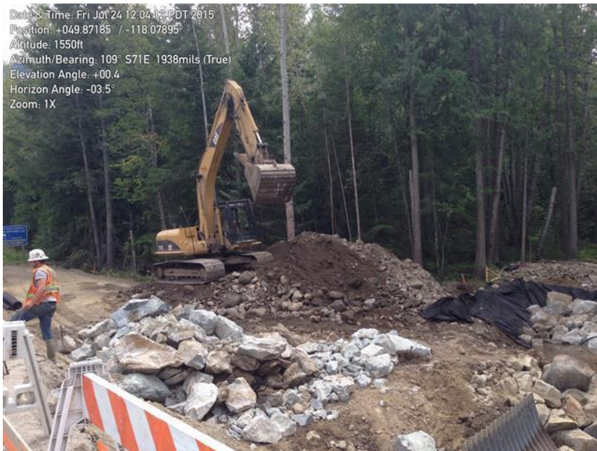
Photo 8 – July 24 – Placement of 500 kg riprap south of Hwy on east bank of Heart creek
