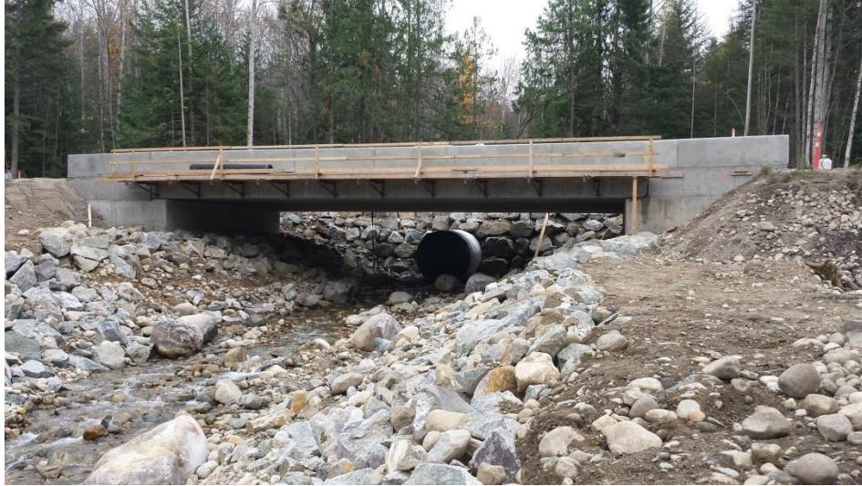
Figure 7. Highway 6 Crossing of Heart Creek (October, 2015)
