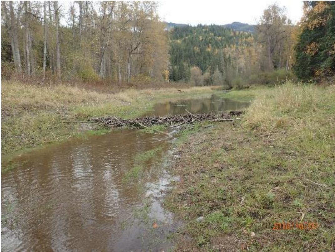
Photograph 21 – Site H2, File Photo 684 (Looking upstream from Waypoint 82)
