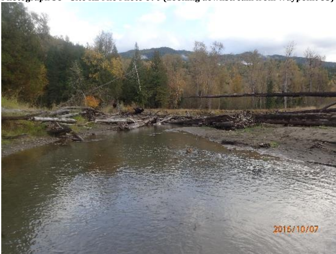
Photograph 39 – Site K2 File Photo 689 (Looking upstream from Waypoint 85)
