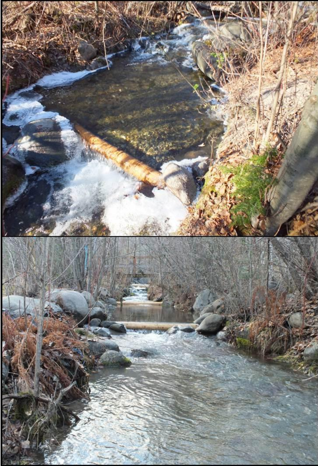
Figure 10. Peeled cedar logs installed in the Murphy Creek spawning channel were used to increase pool depths in a number of shallow pools (Dec 2016)
