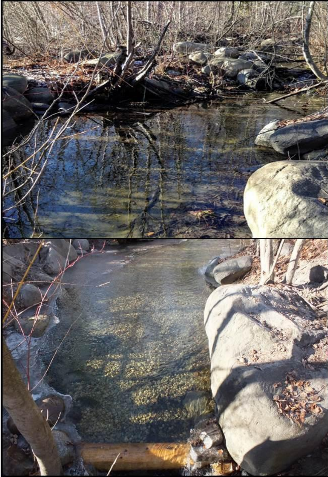
Figure 9. (top) The pool upstream of the walking bridge at the Murphy Creek spawning channel before removal of woody debris and fine sediment (Nov 2015), and (bottom) the pool after removal of woody debris and fine sediment and gravel addition (Dec 2016)
