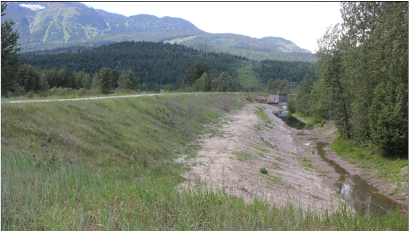
Example dike around Downie Timber's lumber yard in Revelstoke, maintained by BC Hydro. Dike includes clay core, impermeable membrane, topsoil dressing for small shrubs and grass and paved walkway.
