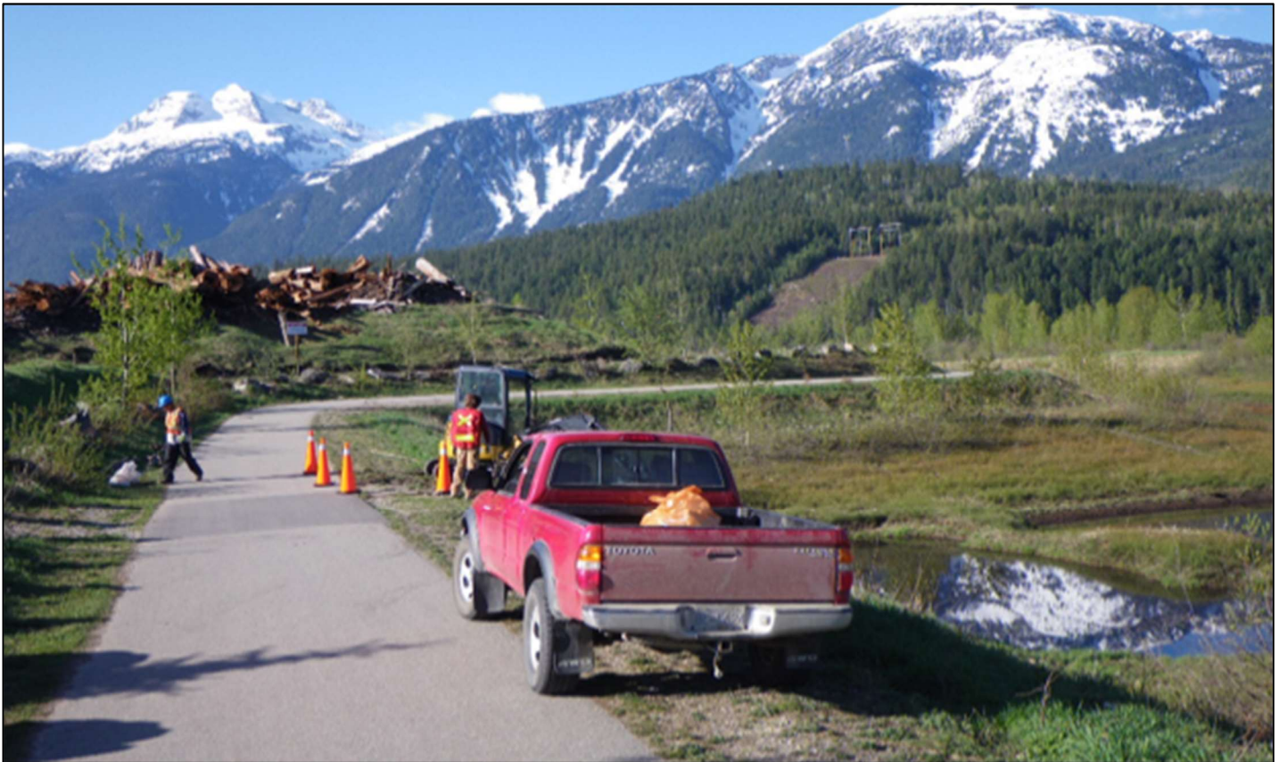
Example dike around Downie Timber's lumber yard in Revelstoke, maintained by BC Hydro. Dike includes clay core, impermeable membrane, topsoil dressing for small shrubs and grass and paved walkway.
