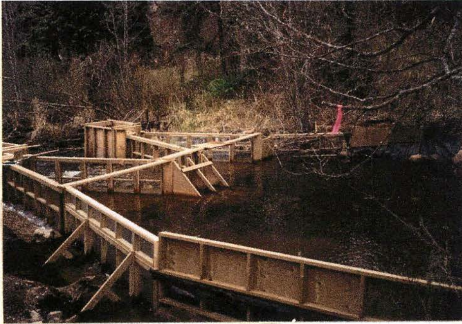
Figure 2. Wolf type weir (above) and inclined plane trap (below) used at Toboggan Creek in the spring of 2001.
