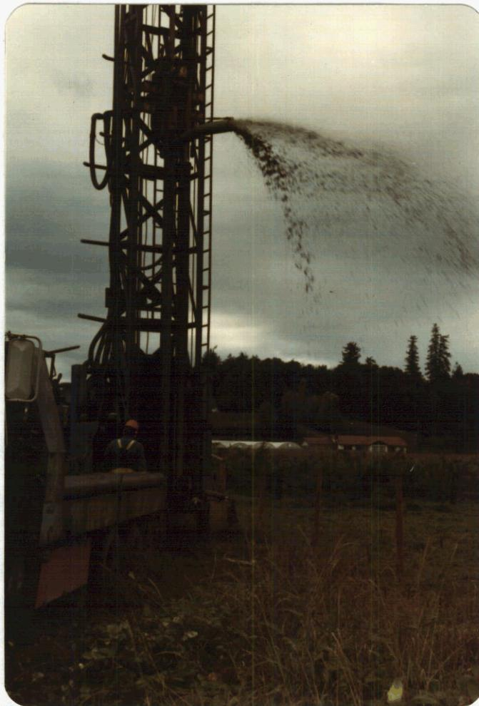
3. Dark brown-black discharge from Obs. Well No. 272, at completion of drilling and flushing.
