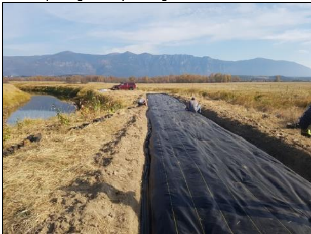
Photo 3. Keying in landscape fabric, Habitat Island 4 solarization plot.
