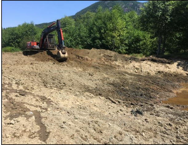
Figure 7: Regrading slope adjacent to pond.
