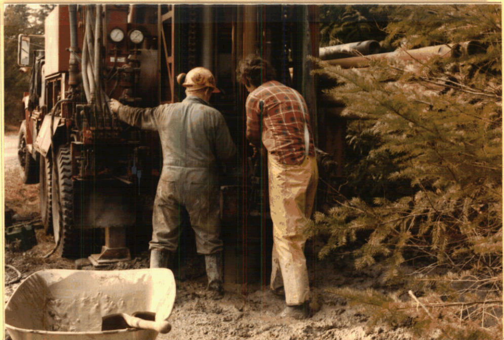
Picture 5. Pulling out the 254 mm (10") \emptyset surface casing
