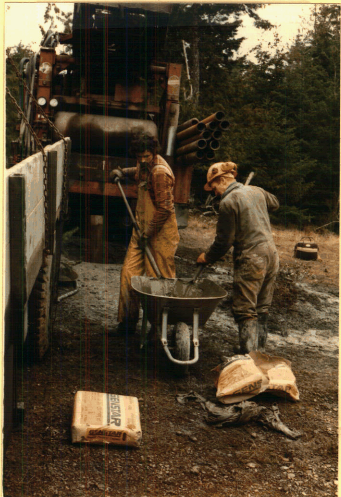
Picture 13. Mixing cement for grouting surface seal
