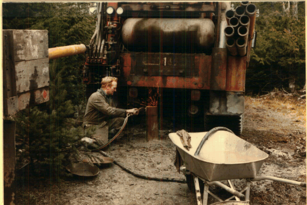
Picture 15. Constructing the well lid
