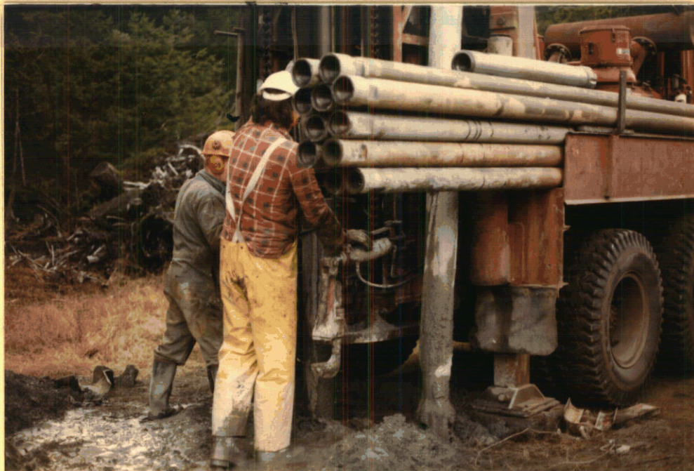
Picture 10. Pulling out 152 mm (6" \emptyset ) surface casing and abandoning testhole #1
