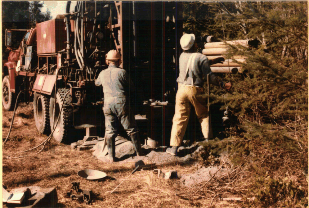
Picture 2. Drilling Obs. Well no. 287 at site #2, Coombs
