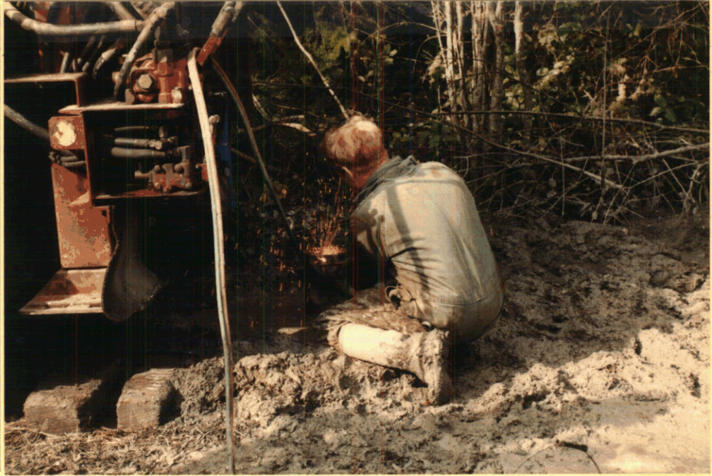
Picture 6. Constructing the well lid
