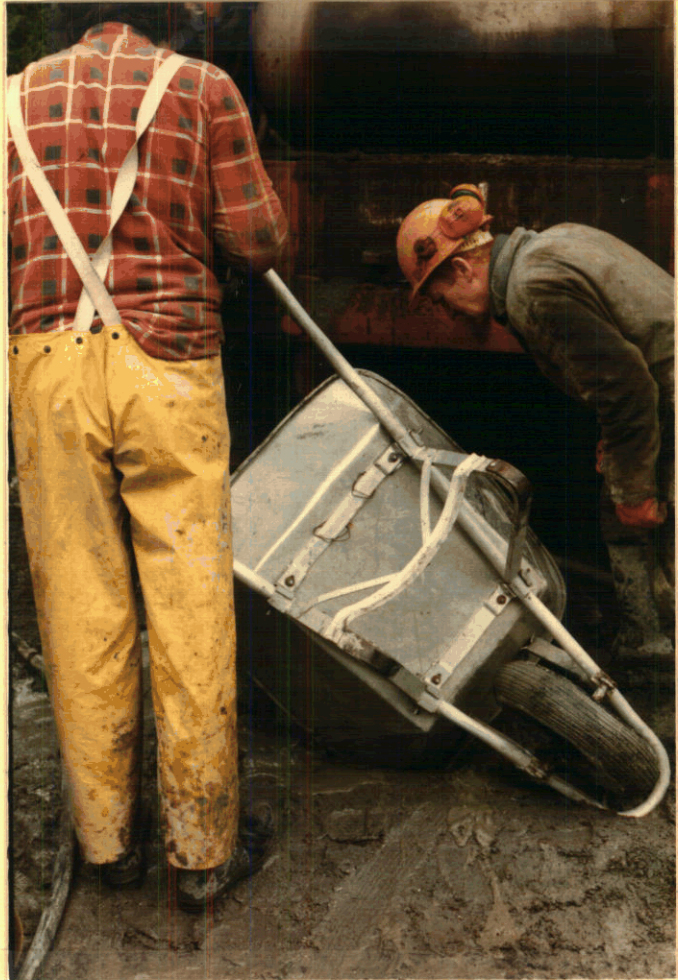
Picture 14. Grouting surface seal
