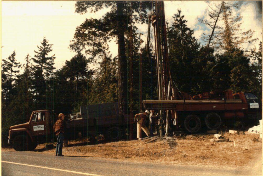
Picture 12. Drilling Obs. Well no. 288 at site #2, Hornby Island
