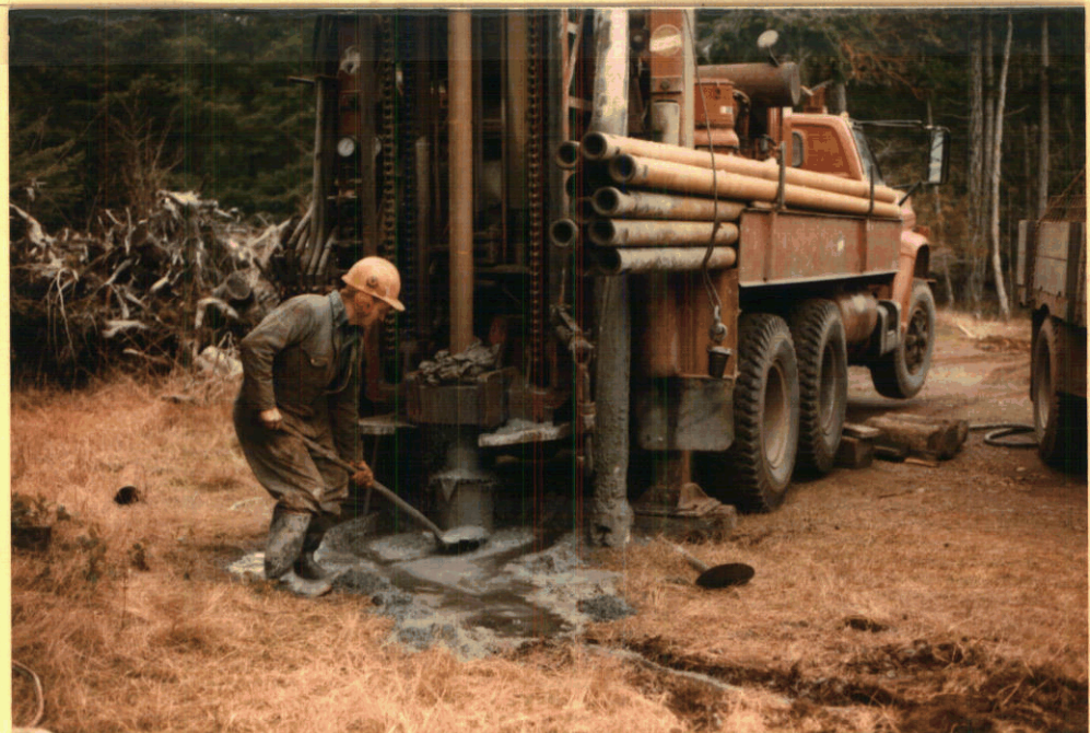
Picture 9. Drilling testhole #1 at site #1
