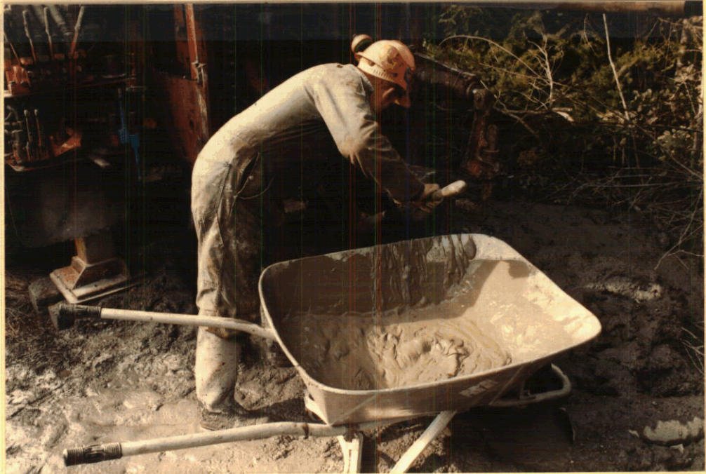
Picture 4. Grouting the surface seal
