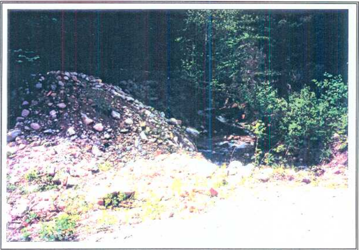
PHOTO 14. Tributary channel to Camp Creek at 25.25 km on Glen Lake Main. Channel deposits are associated with two road related landslides. (June 1996 - ID# 4-3)
