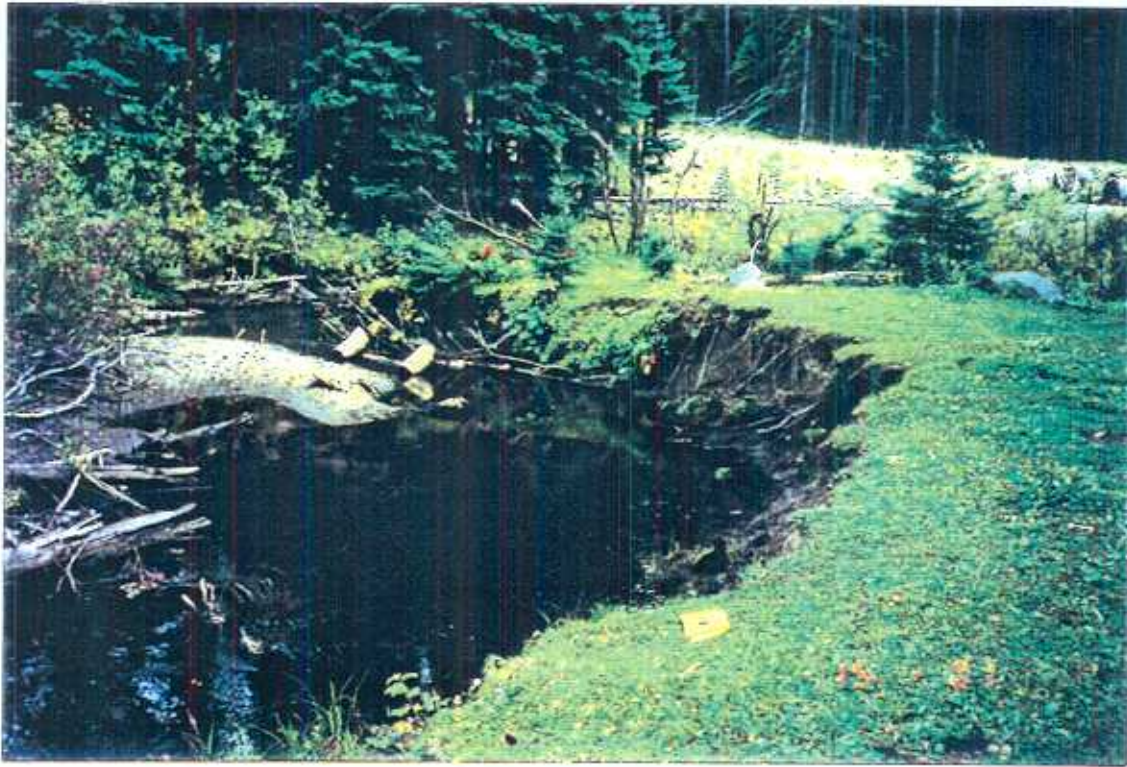
PHOTO 33. Bank erosion partially due to cattle trampling and compaction of streambanks in the Upper Trout Creek sub-basin. (September 1995 - ID# 8-2)
