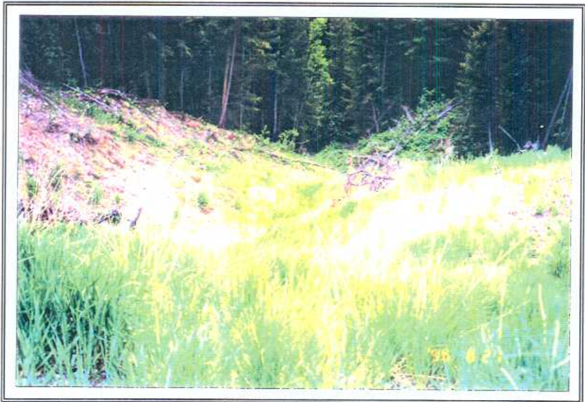
PHOTO 21. A road related landslide above the tributary shown in Photograph 14. (June 1996 - ID# 3-14)
