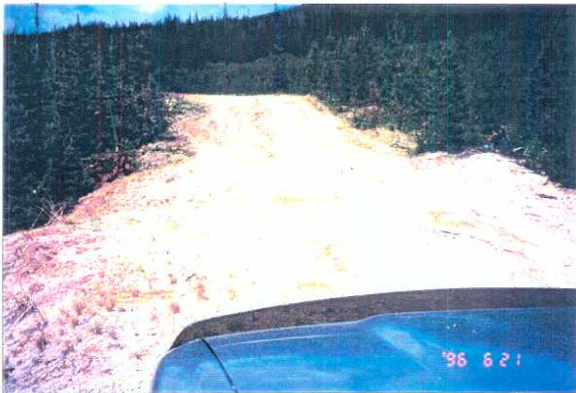
PHOTO 12. Road surface erosion in the upper Lost Chain Creek sub-basin. (June 1996 - ID# 5-1)
