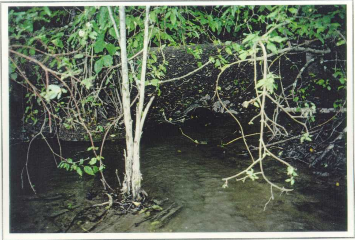
PHOTO 11. Culvert inlet at Beatrice Road crossing.
