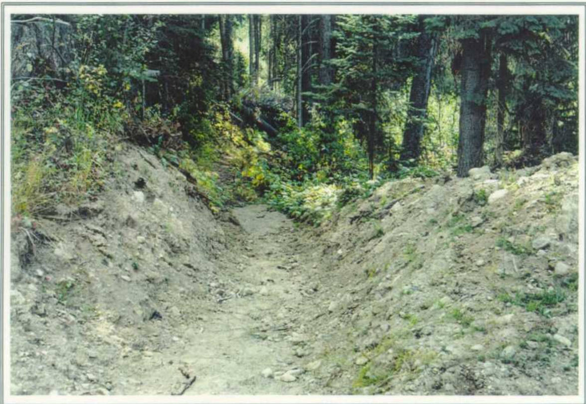
PHOTO 6. Recent (1998) ditchline cleaning and sump construction downslope of “throttle hill”. Fine sediment (sand and silt) still reaching Duteau Creek.
