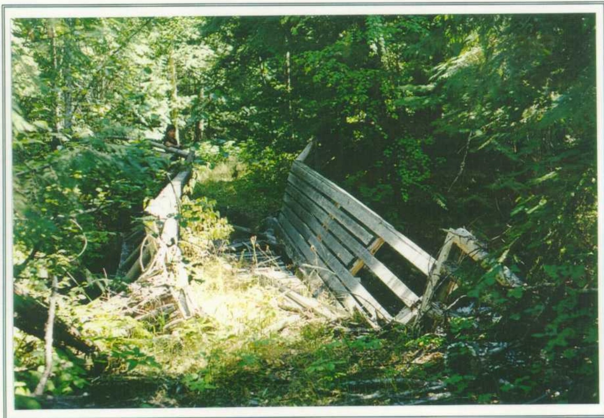
PHOTO 28. Old cattle bridge over mainstem channel (reach D) above Headgates reservoir.
