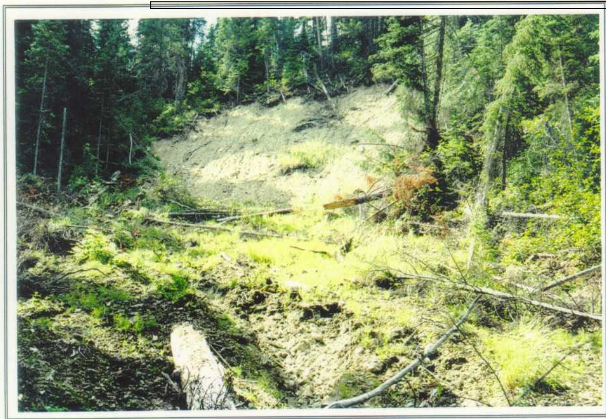
PHOTO 8. 1997 slide into Duteau Creek from canyon wall approximately 0.5 km downstream of the Haddo FSR road crossing. This site was bioengineered in the fall of 1998.
