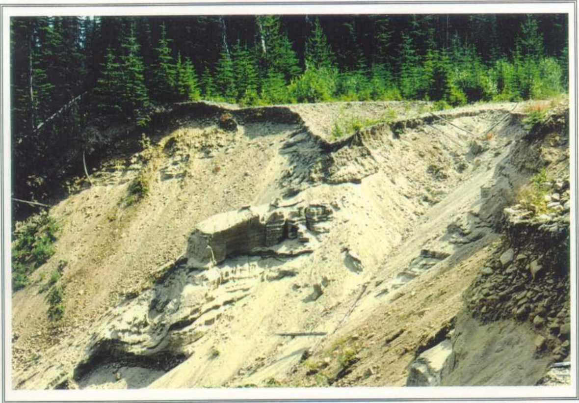
PHOTO 7. Failure from the 533.1 road in the upper Duteau Creek sub-basin.
