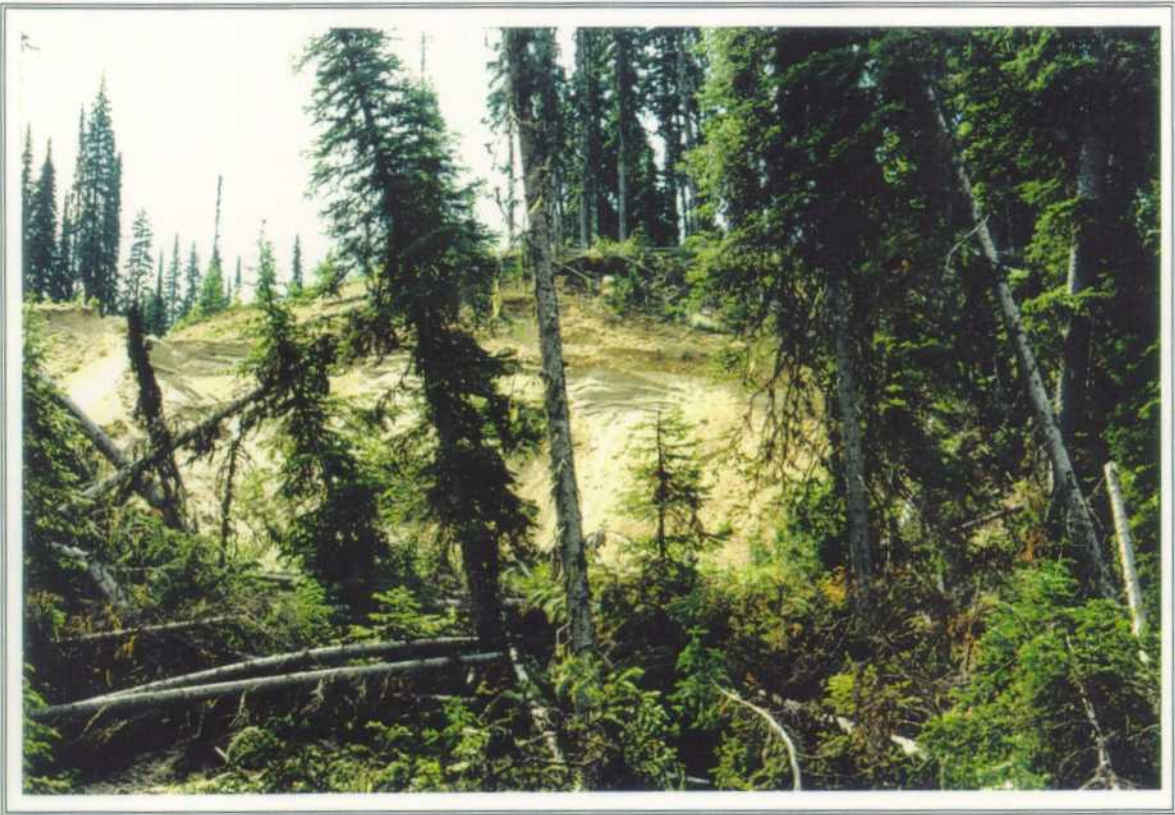
PHOTO 9. Failure from the 533.1 road showing cross-bedding in isolated glacio-fluvial gravel, sand and silt deposits in the upper watershed.
