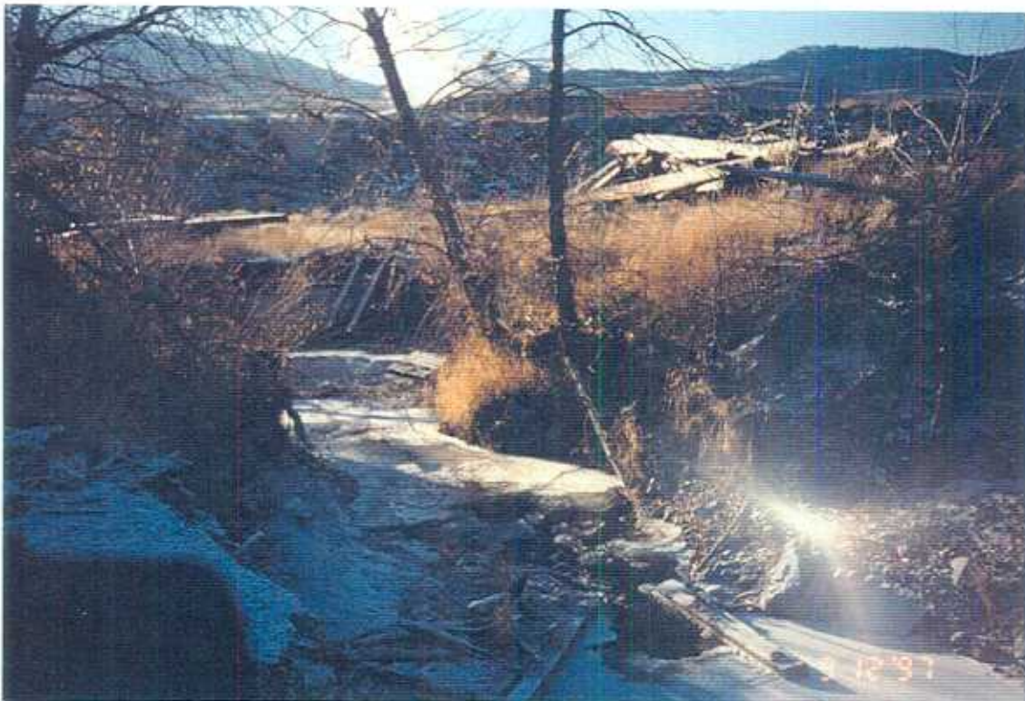
Plate 4: (Site 2) Approximately 30 metres upstream of bridge crossing Durand Creek looking upstream with Ainsworth Lumber Company, Savona Division in the background; debris in creek (December 9, 1997)
