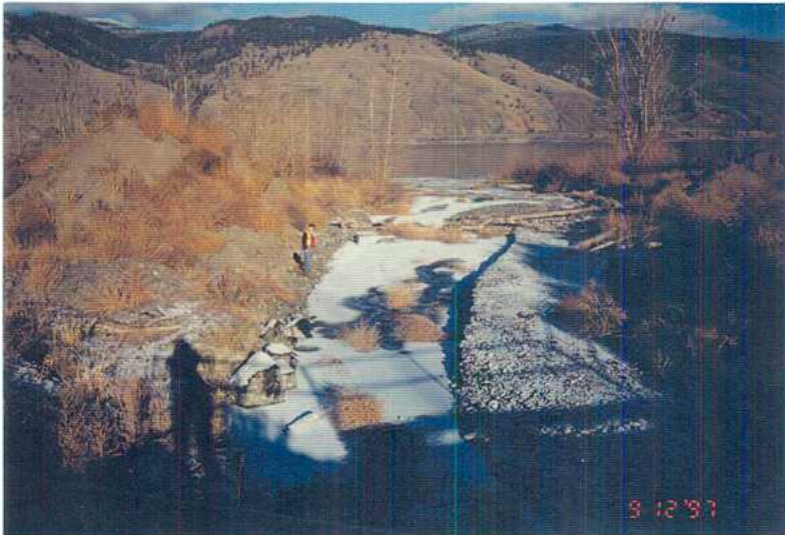
Plate 1: (Site 1) Mouth of Durand Creek and Kamloops Lake; looking north from bridge (December 9, 1997)
