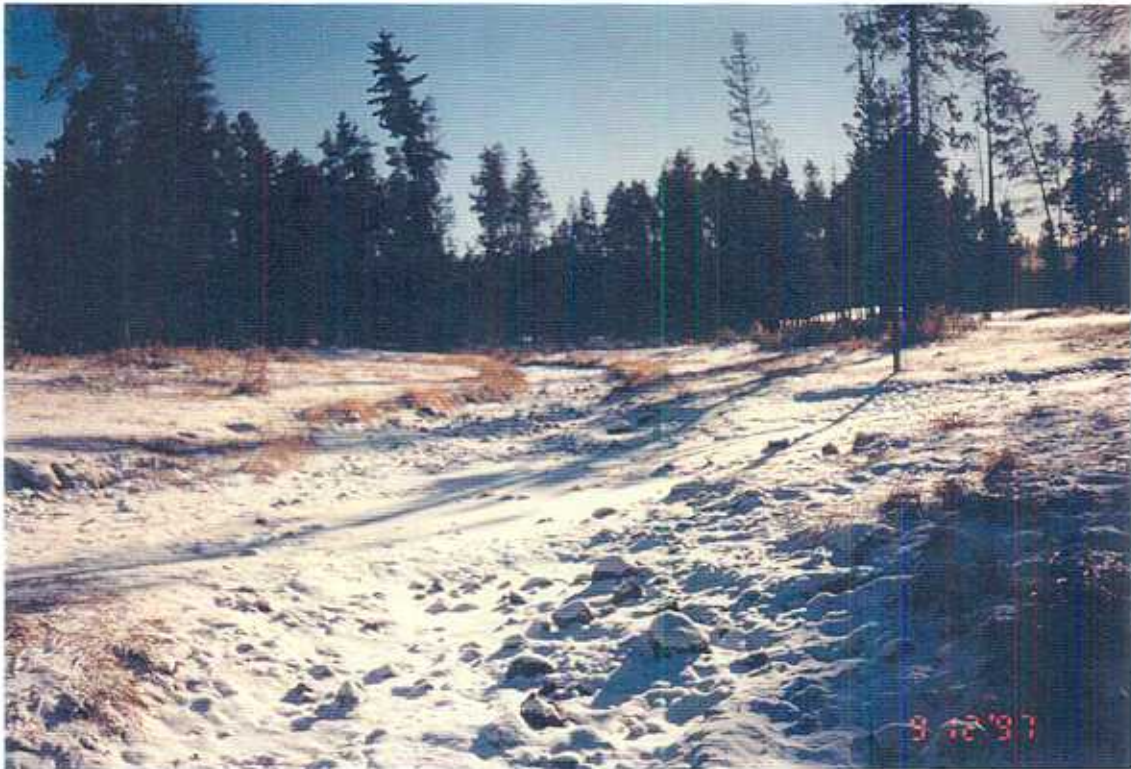
Plate 7: (Site 4) Spillways/diversion ditch on Leighton Lake at Tunkwa Creek (December 9, 1997)
