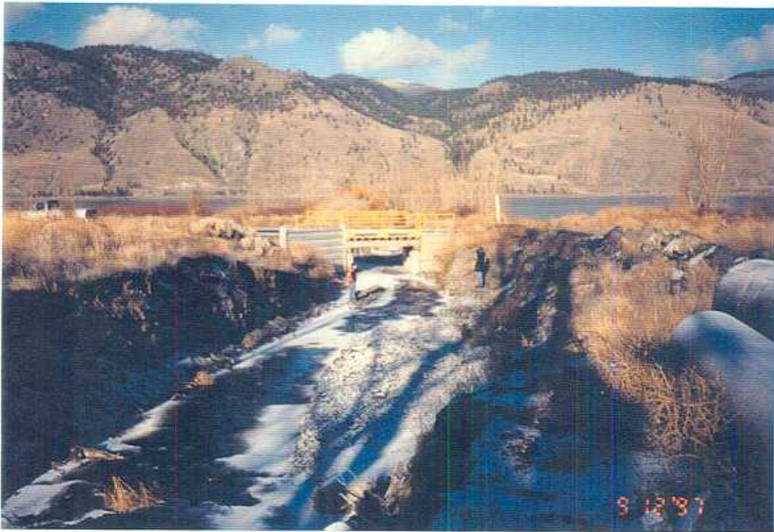
Plate 3: (Site 2) Approximately 30 metres upstream of bridge crossing Durand Creek looking north towards Kamloops Lake (December 9, 1997)
