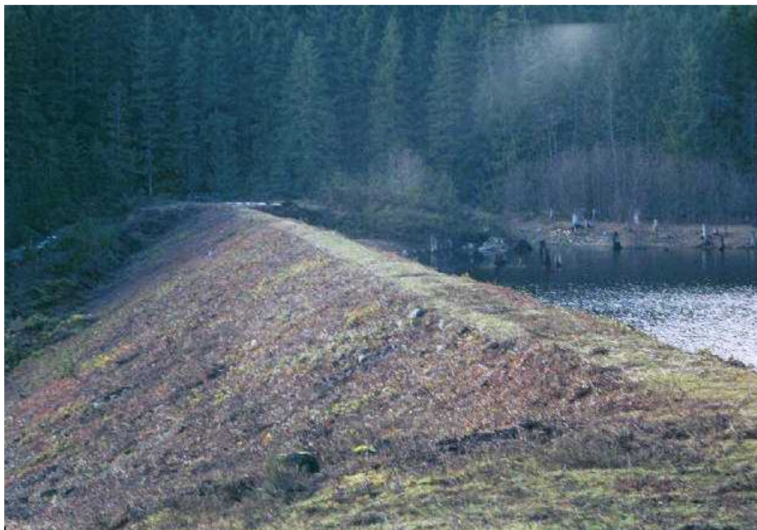
Dam at Jack Reservoir, Structural stage 3a.
