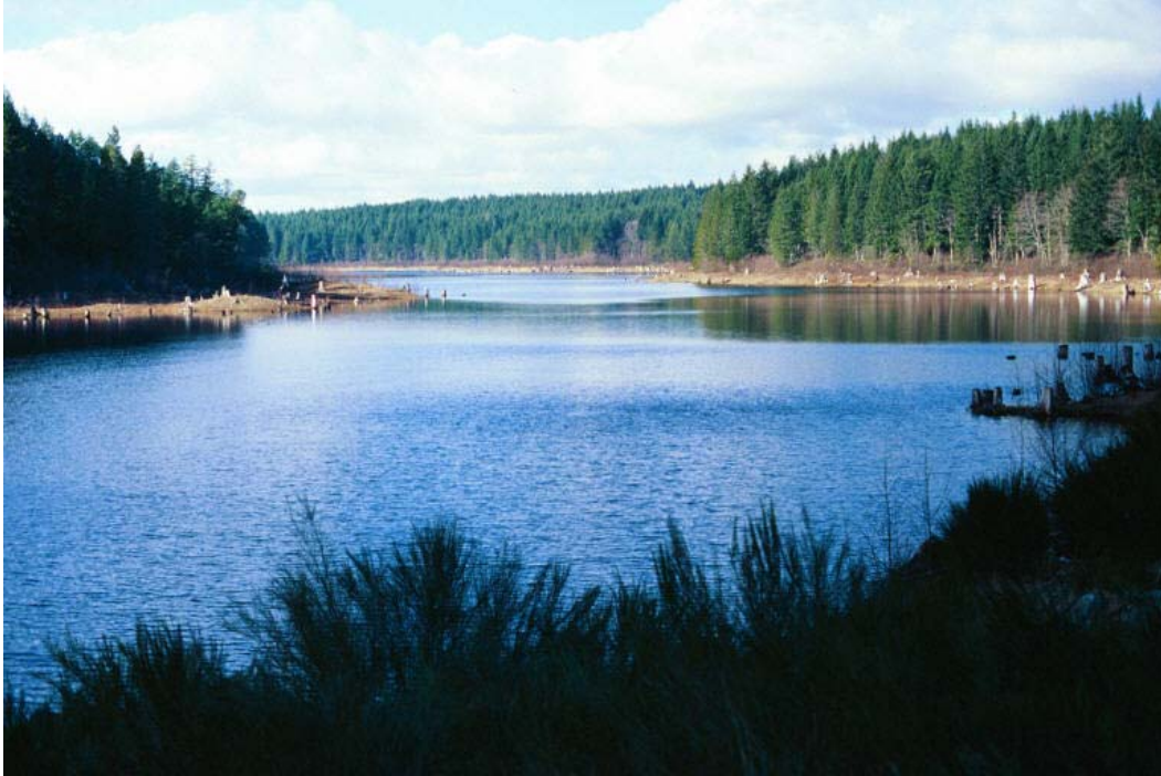
Figure 9: Basin of Jack Reservoir
