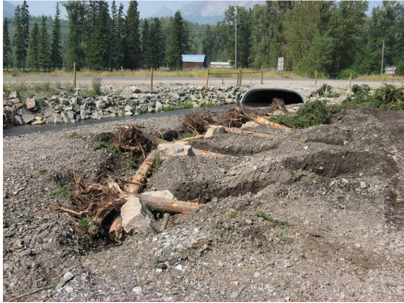
Figure 7: Series of six rootwads installed on deposition bank immediately downstream of the Highway 3 crossing.
