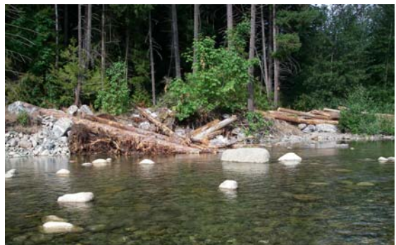
Photo 8. Newly constructed LWD structure at the bottom of the "Long Run".
