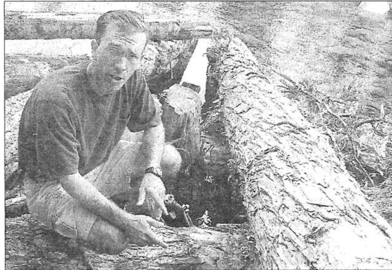
FISHERIES TECHNICIAN FOR the British Columbia Conservation Foundation, James Craig, indicates how boulders and large wood is anchored alongside the Englishman River to create a safe environment for fish.
