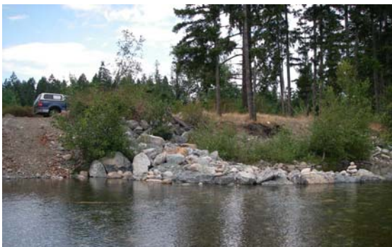
Photo 7. Constructed rock deflector groyne at the top of the "Long Run".
