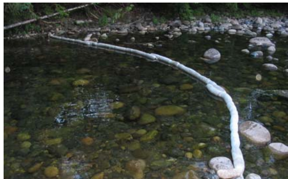
Photo 4. Typical environmental controls (oil boom) installed in the Englishman River.
