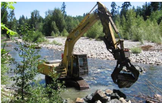
Photo 5. Excavator with clamshell bucket positioning deflector groyne rock.
