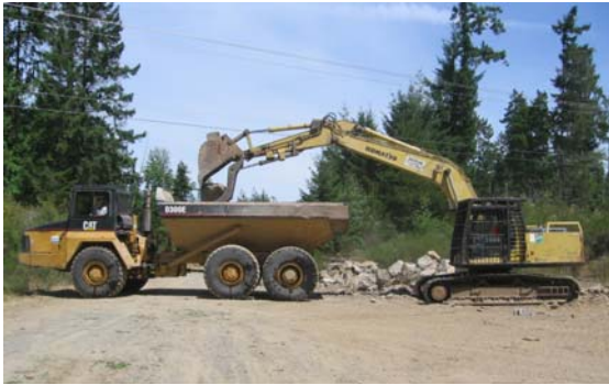
Photo 1. Ballast rock loading into the 6-WD articulated hauler.
