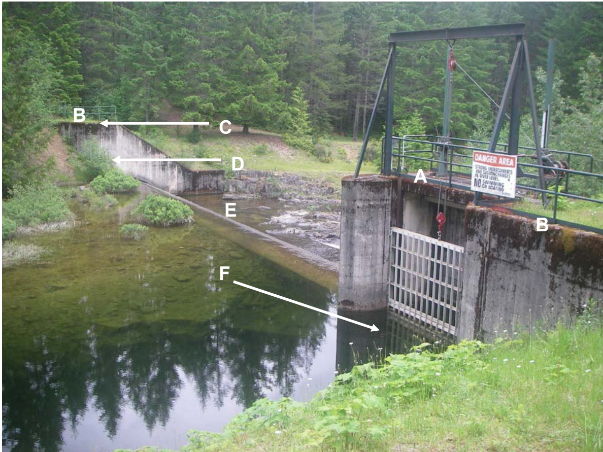
BC Hydro storage dam including spillway (E), sluiceway (F) and trash rack (A) at outlet of Wokas Lake, upper Quinsam River.
