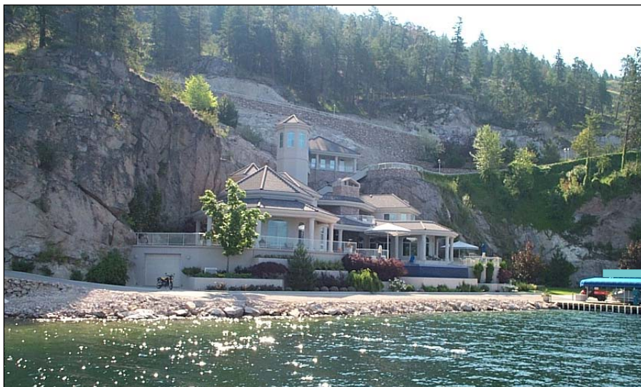
Foreshore modifications include lake infilling, removal of riparian vegetation, dock structures and blasting of parent foreshore material.
