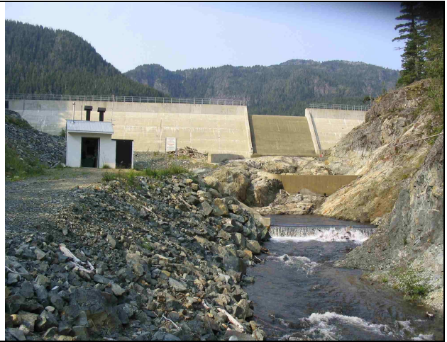
2. Arrowsmith Dam (July 2004)
