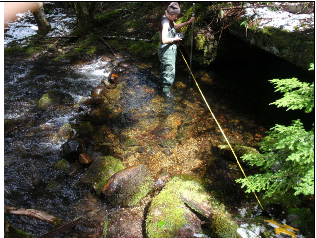
35. Measuring discharge in Shelton Creek, immediately downstream of Spur C-26 box culvert, May 14, 2009.
