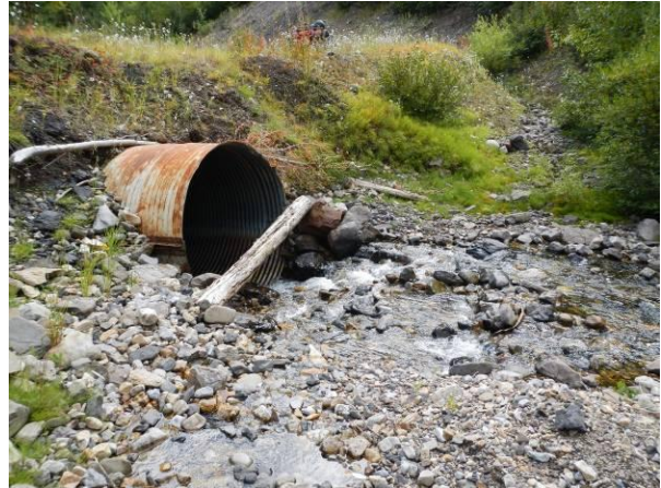
Inlet of culvert. Note high depth of road fill (> 1.00 m).
