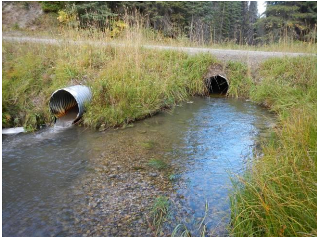
Outlet of culverts.
