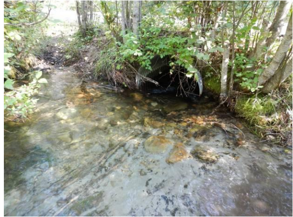
Inlet of culvert.
