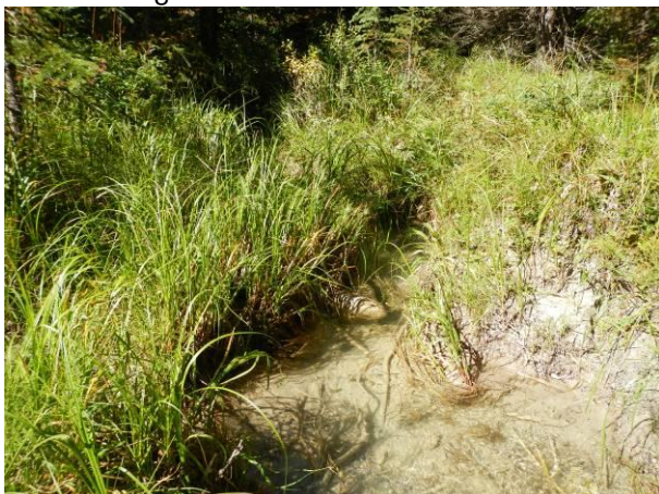
Downstream from culvert.
