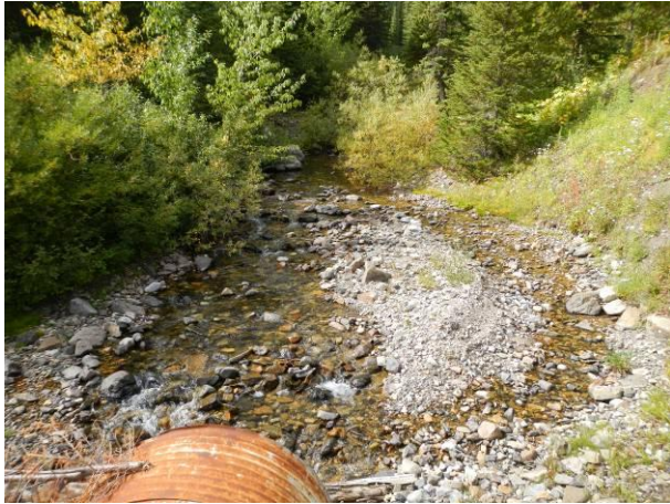
Upstream of inlet.
