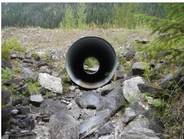
Culvert barrel at outlet of White20.
