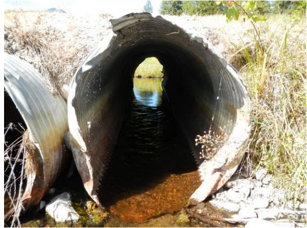
Barrel of left downstream culvert at outlet.
