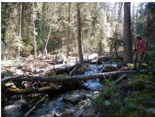
Channel is highly disturbed upstream of culvert with abundant large woody debris. Disturbance was caused by upstream cable logging.
