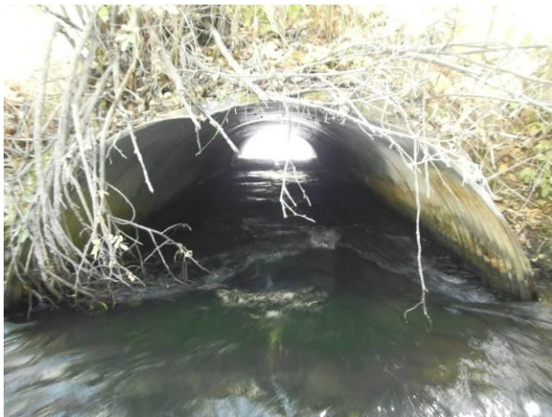
Culvert barrel at inlet.
