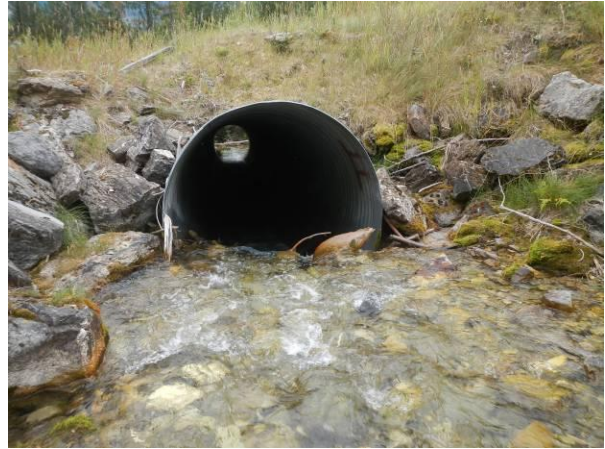
Inlet of culvert with inlet drop (0.70 m).
