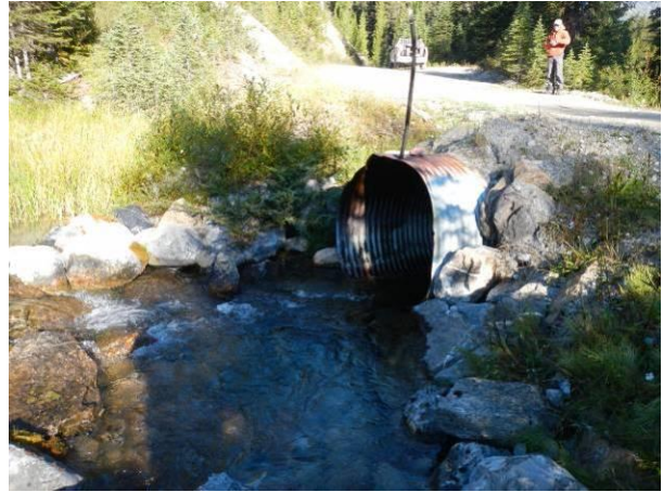
Inlet of culvert.
