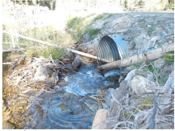
Inlet of culvert.
