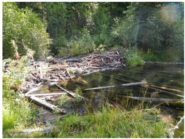
Permanent beaver dam upstream of culvert.
