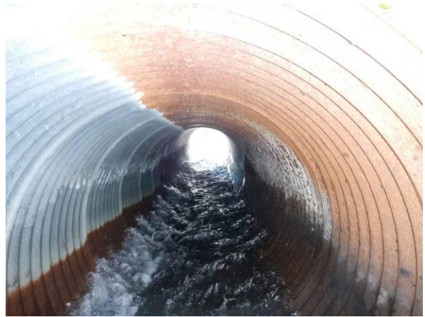
Barrel of right downstream culvert.
