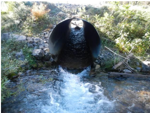
Culvert barrel at outlet.
