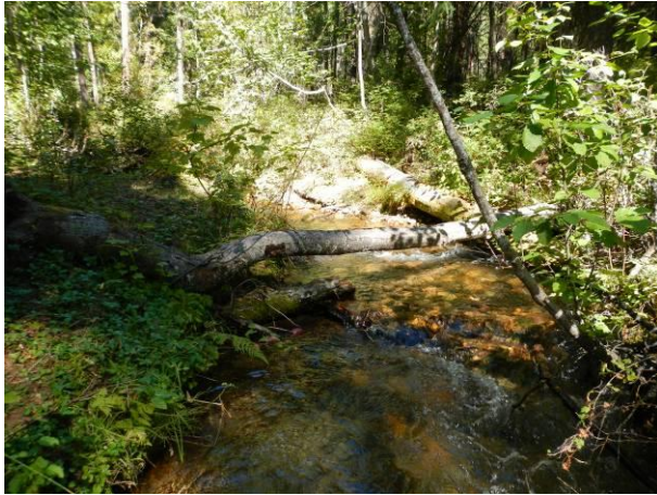
Upstream of culvert
