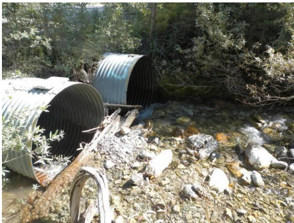
Inlet of culvert.
