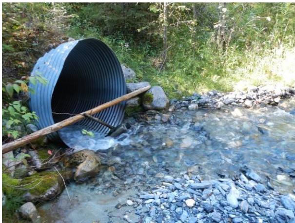
Inlet of culvert.
