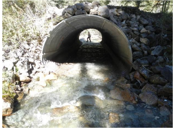
Inlet of culvert.
