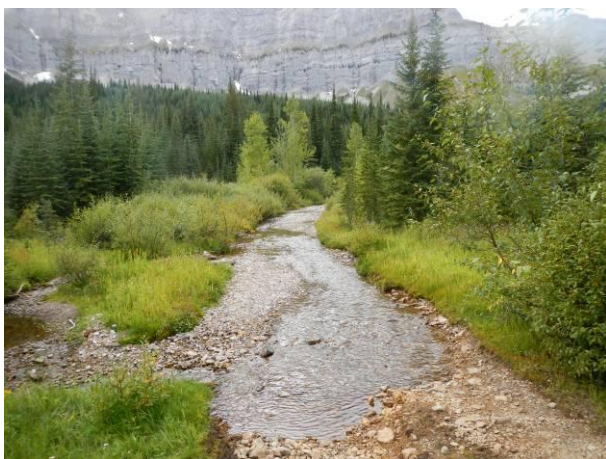
The stream washes out the road at approximately 1.93 km upstream from culvert. A 2.00 m high waterfall (>20% gradient) was also located at the washout area.
