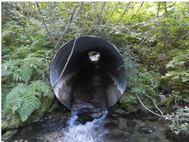
Outlet and barrel of culvert.
