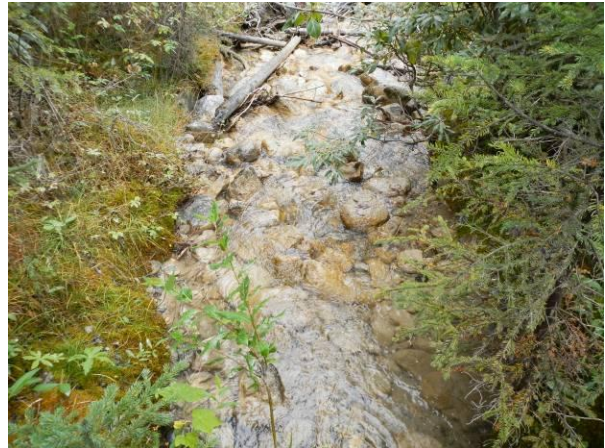
Downstream view from outlet.
