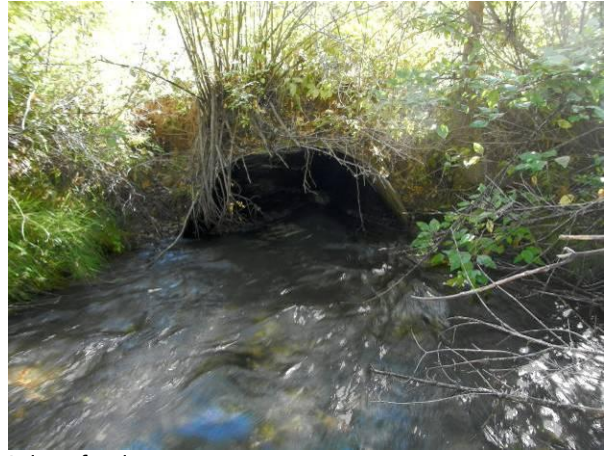
Inlet of culvert.
