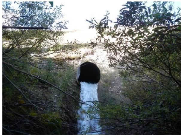
Road fill is approximately 10.00 m deep.
