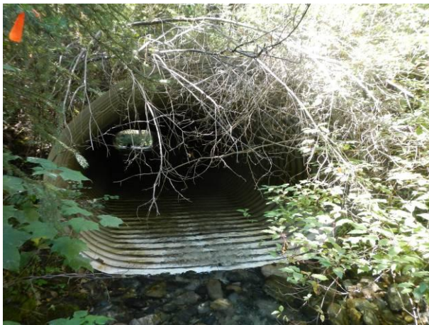
Inlet and barrel of culvert.
