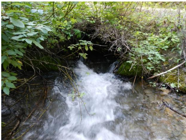
Outlet of culvert.
