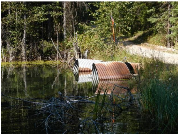
Inlet of culvert.
