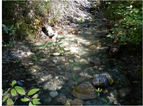
Upstream view from inlet.
