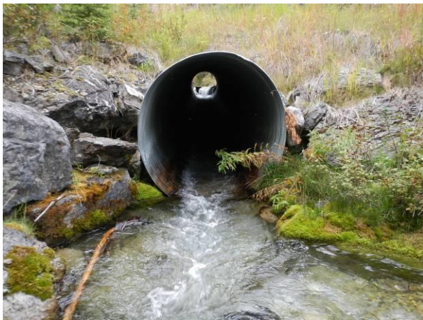
Outlet of culvert.
