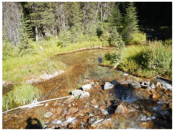
Downstream view from culvert.
