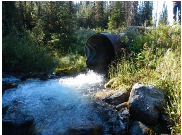
Outlet of culvert.
