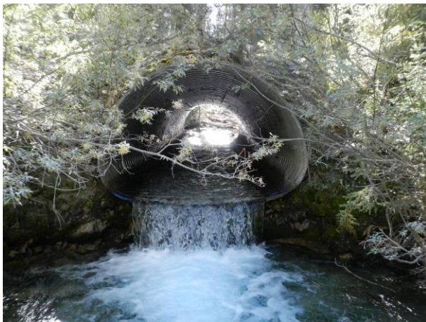
Outlet of perched culvert.
