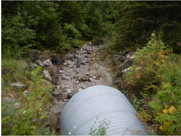
Upstream of inlet of White19.
