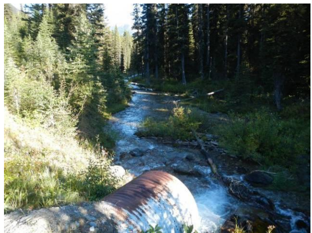
Downstream view from culvert.
