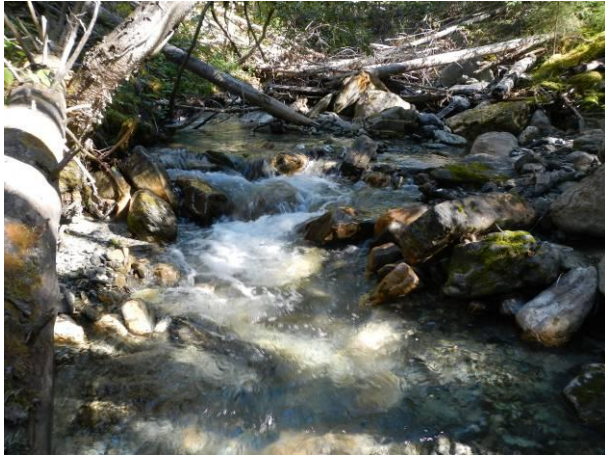
Upstream of culvert.
