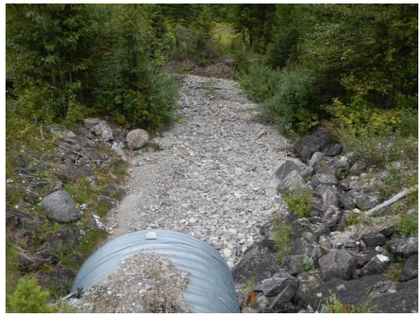
Upstream of inlet of White 20.
