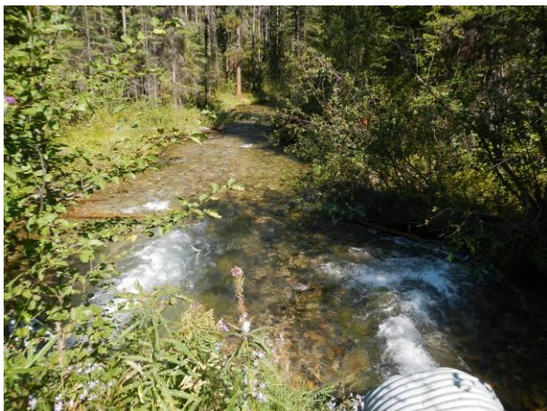
Downstream view from culvert.
