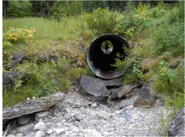
Culvert barrel at outlet of White19. Backwatering was attempted.
