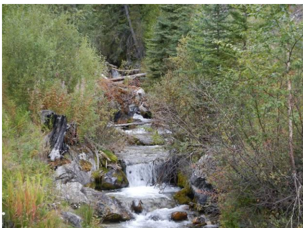
Waterfalls and large woody debris upstream of culvert.
