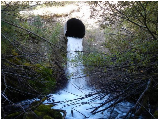
Outlet of culvert.
