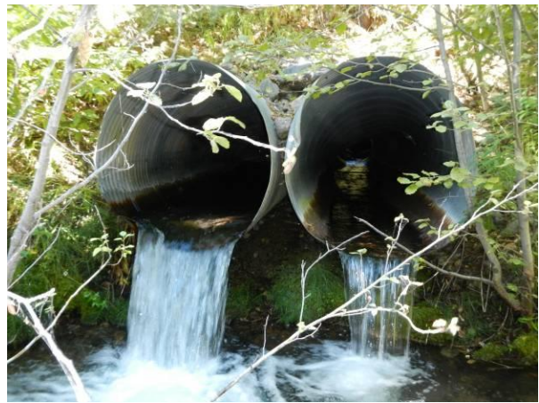
Outlet of culvert. Note that culverts are perched.
