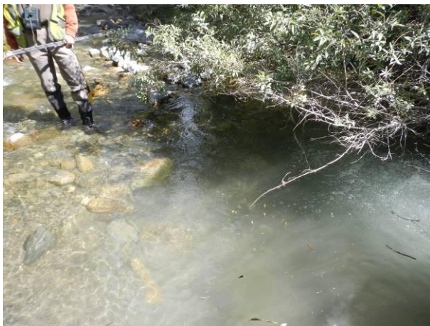
Downstream view from culvert. Pooling at outlet.
