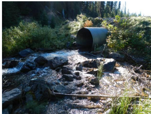
Outlet of culvert.
