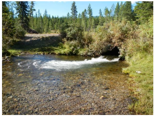
Outlet of culvert.
