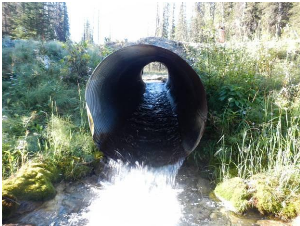
Culvert barrel at outlet.
