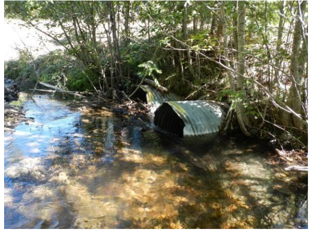
Inlet of culvert.
