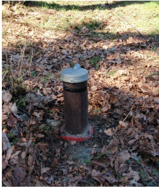
Figure 38 Well head located outside. Casing has been extended above ground with a bolted gasket so standing water does not accumulate within a depression around the well
