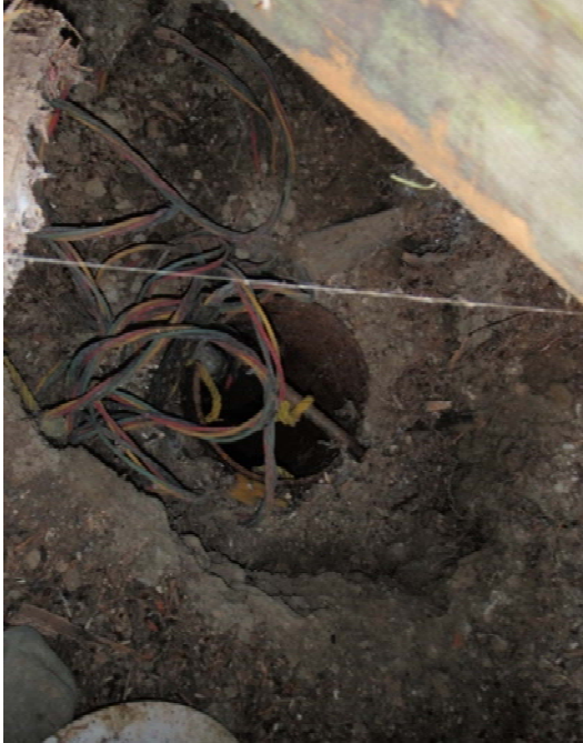
Figure 35 Well head located outside within wooden enclosure, with casing cut low to ground and no cap. The sample from this source had 260 CFU/100 ml total coliforms but no E. coli
