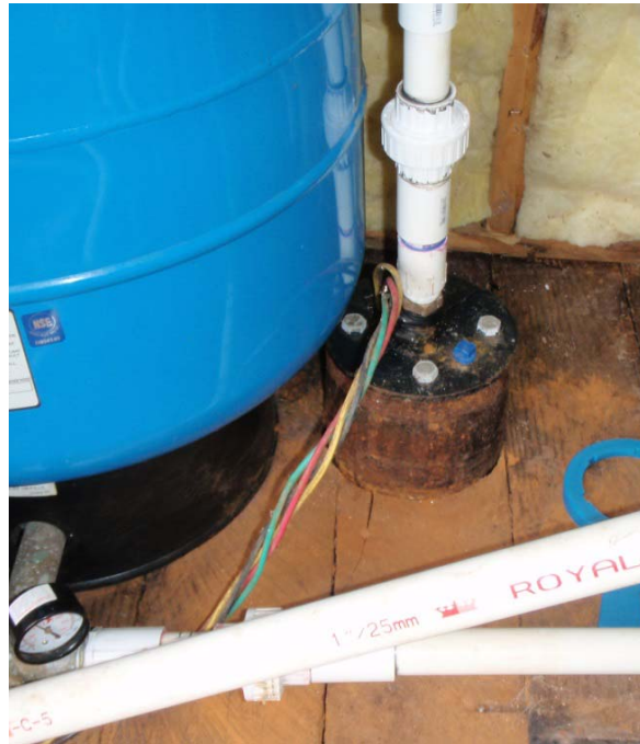
Figure 34 Well in pump house with sanitary seal that is properly installed and prevents contaminants from entering the well
