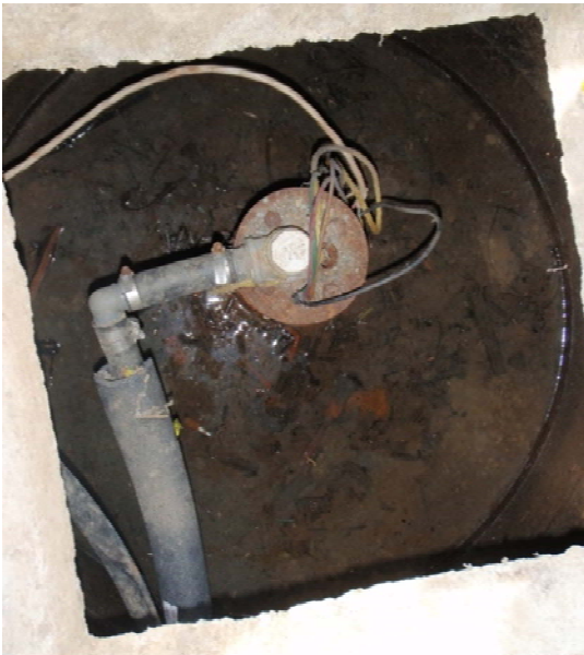
Figure 37 Well head located within a cement enclosure allowing accumulation of standing water around the well making it vulnerable to contamination
