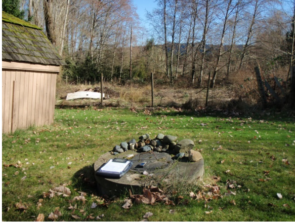
Figure 31 Older dug well with access hatch in the centre. Surface water and contaminants can enter in the gap around the cement insert/cover
