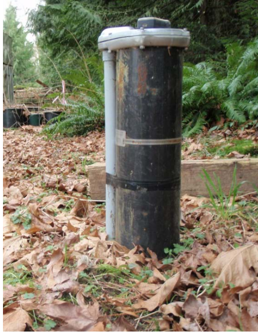
Figure 36 Well head located outside with pitless adapter and bolted cap is protected from contamination
