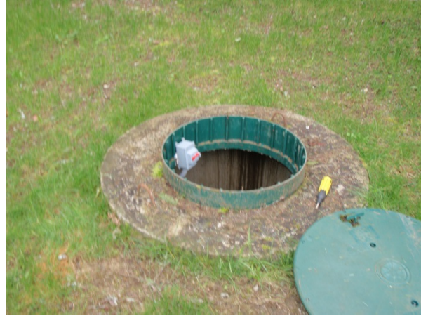
Figure 32 Dug well retrofitted with sealable lid that can be removed by loosening the bolts, and when in place provides a water-tight and vermin-proof seal
