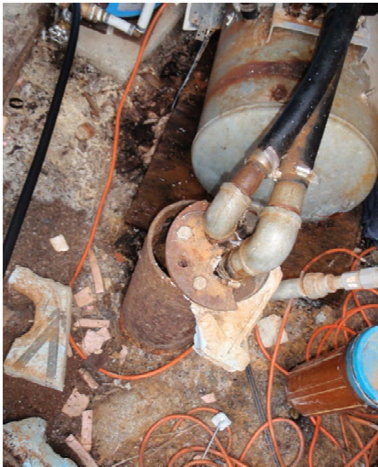
Figure 33 Well in pump house with sanitary seal type cap that has been partially removed allowing contaminants to enter the well
